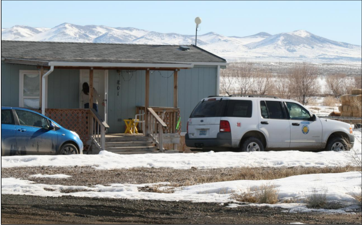
Figure 15. A building inspector calling on a house to conduct a post-earthquake inspection. The green flag indicates the house was deemed inhabitable by the initial safety inspectors.
