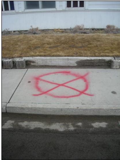
Figure 12. A spray painted circle with an “X” in it on the sidewalk indicates the building was inspected and is too damaged for human occupancy.
