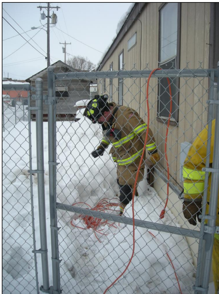
Figure 3. Fireman checking for leaking gases near a manufactured building that shifted on its support blocks. Photograph by Wells resident.
