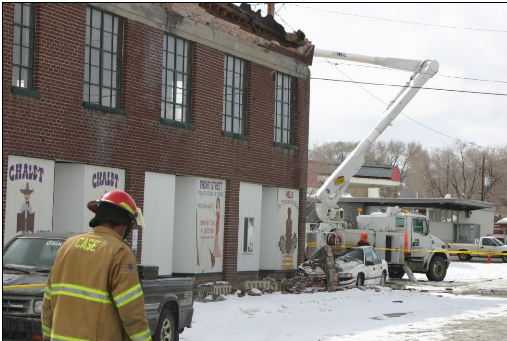
Figure 2. Disconnecting power to damaged buildings in the historical district. Photograph by the Utah Division of Homeland Security.
