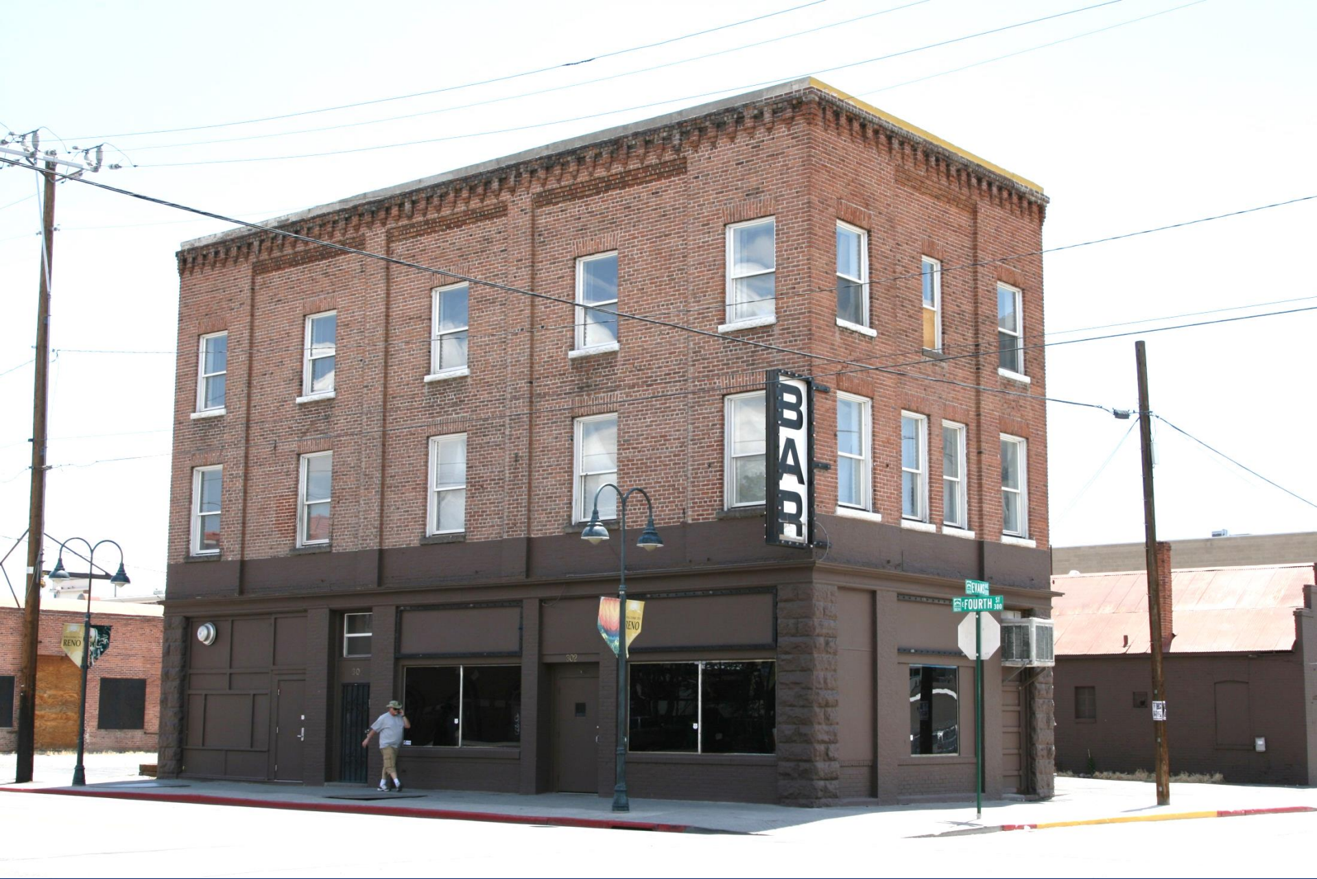
Three story URMB with some earthquake cracks; occupancy is variable
