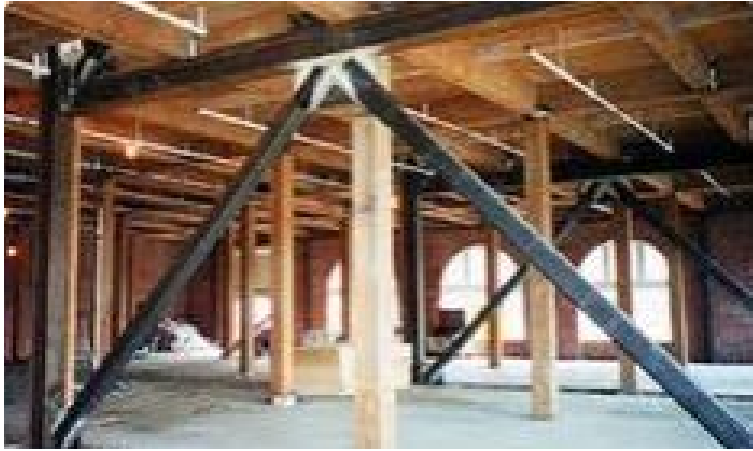
Interior cross bracing helps prevent building collapse
