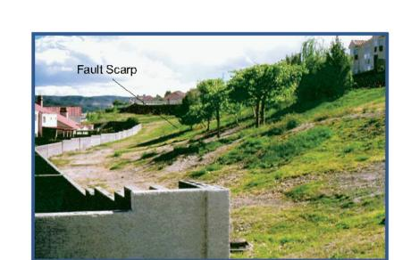
Figure 4. Setback of homes away from a Quaternary fault in Las Vegas. The
