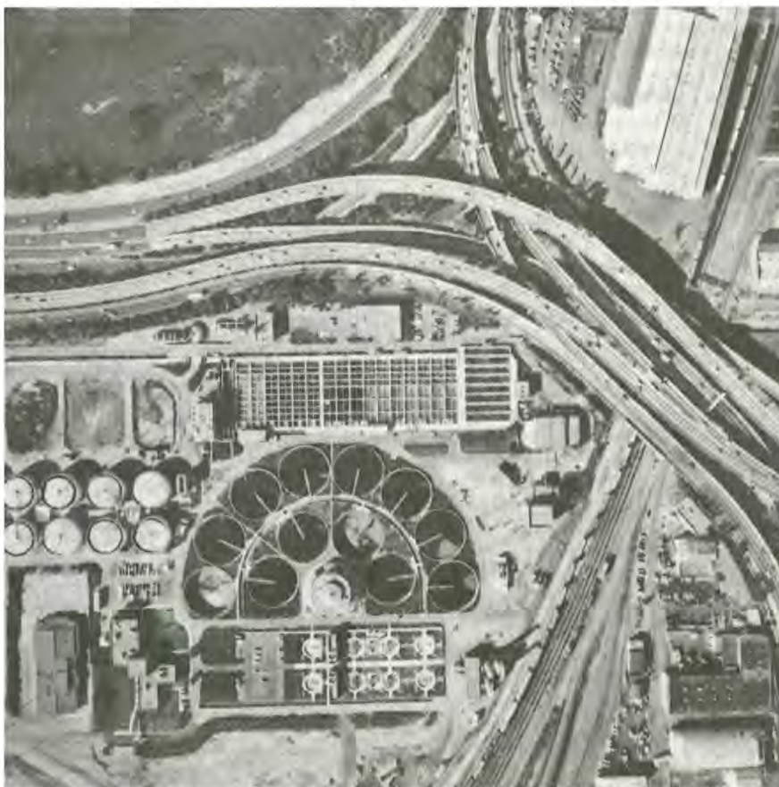
The Bay Bridge east approach interchange (I-80/580), main line railroads, and EBMUD's Special District Number 1 waste water treatment plant.
