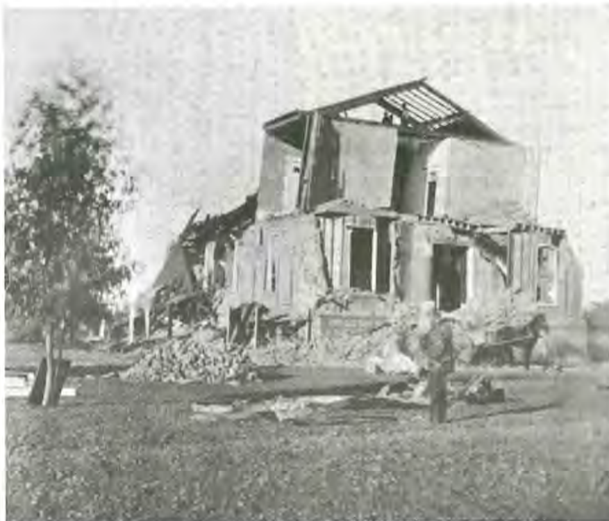
Courthouse at San Leandro after the Hayward earthquake of October 21, 1868.
