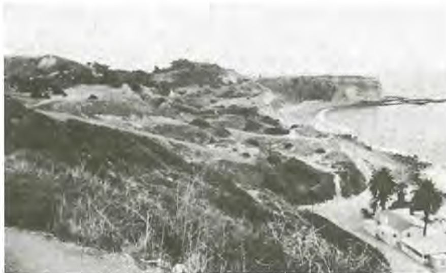
Abalone Cove landslide, Rancho Palos Verdes, Los Angeles County. The toe of the landslide is at the shoreline. The Abalone Cove Landslide Abatement District was formed in January 1981, and was the first district formed after the Beverly Act of 1979. Photo by Martin L. Stout.
