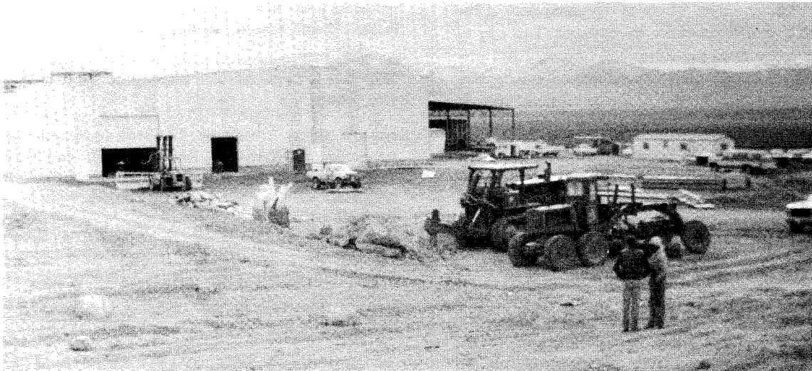
Figure 5. Vegetable-dehydration plant under construction in the San Emidio Desert. Larry Green photo.
