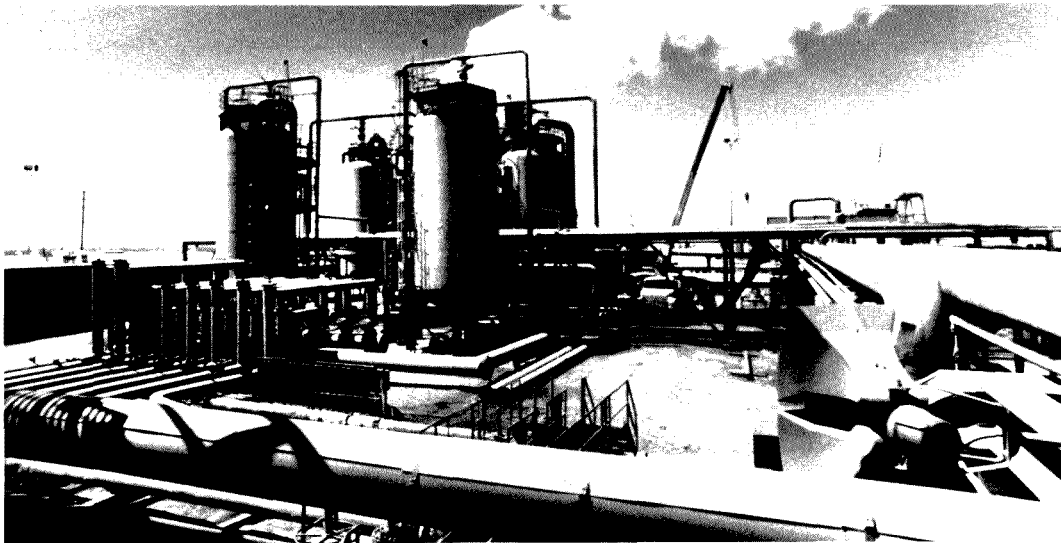
Vertical crystallizer tanks of a flash steam plant near the Salton Sea. This technology was developed at the GLEF especially to tap the Salton Sea reservoir's very desirable high temperature and 3,000 to 4,000 MWe electric generation potential. The crystallizer/clarifier concept will be used at many other high salinity sites. (Courtesy of Goslin Birmingham, Inc.)
