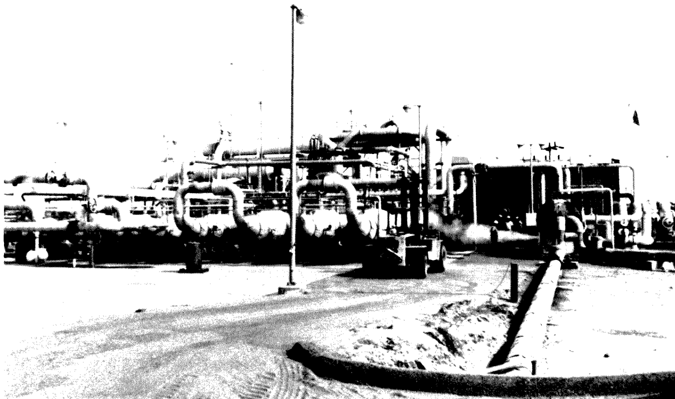
Magma Power Co. geothermal binary power plant at East Mesa, being enlarged from 10 to 12.5 MWe.
