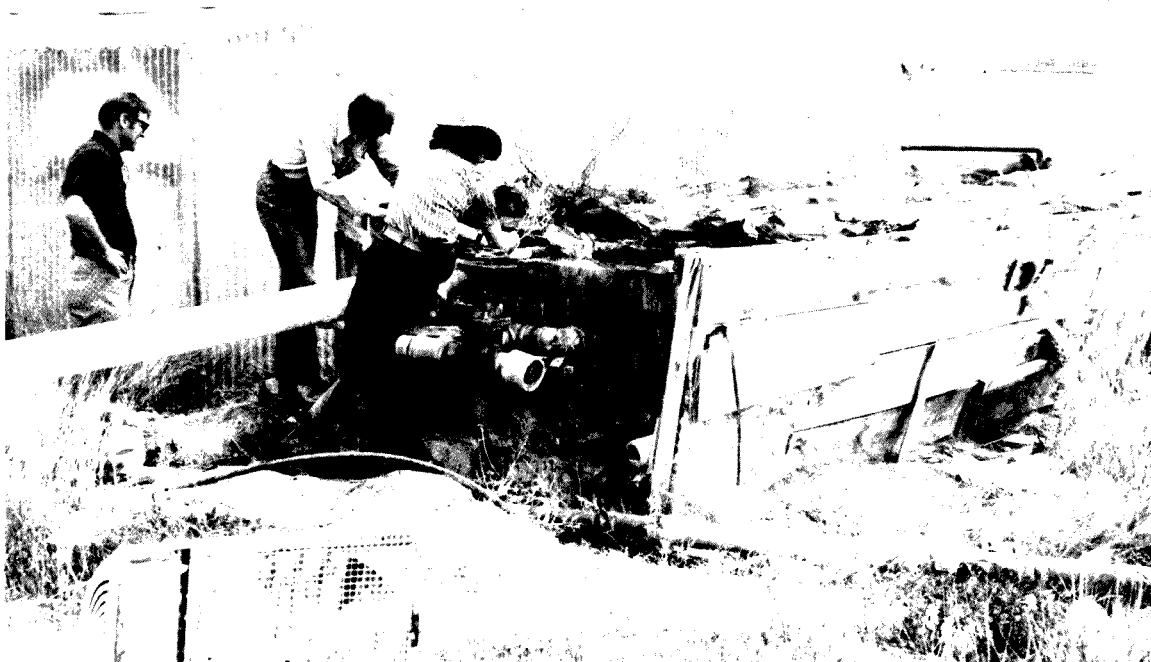
1974 geothermal greenhouse in Raft River Valley, Idaho. The heat exchanger (shown here) was a tub of hot geothermal water (180°F).
