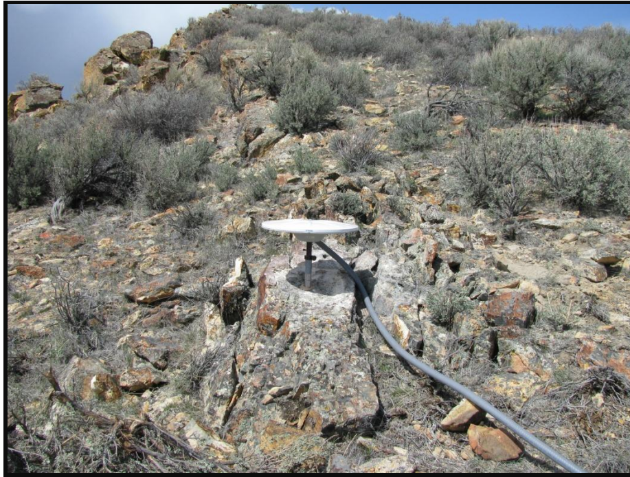
Figure 8. Photograph of antenna for GPS site WLLS, which is now transmitting data daily to the Nevada Seismological Laboratory and Nevada Geodetic Laboratory, with the option of streaming high-rate data in real time. The location of this site is within 7 km of the epicenter and is shown in figure 1.
