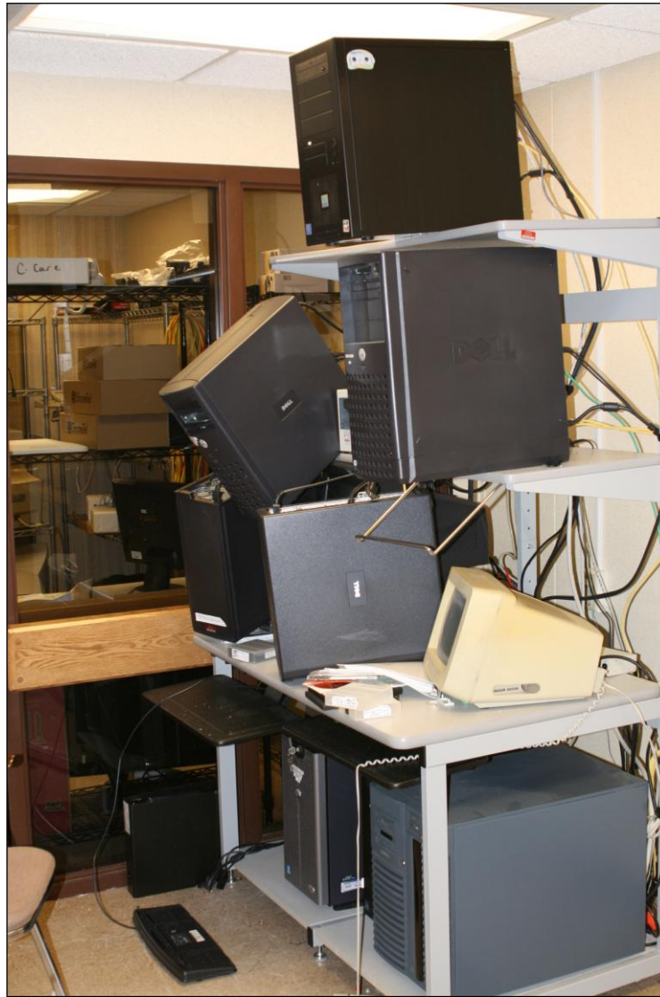
Figure 9. Remarkably resilient servers used by Wells Rural Electric. Although two servers fell onto the desk and others shifted, they remained connected and operating through the earthquake and afterwards (the fall was cushioned a little by books and papers on the table). The servers on the floor rack do not appear to have shifted at all. Photograph taken by Layla Walz of Wells Rural Electric Company.
