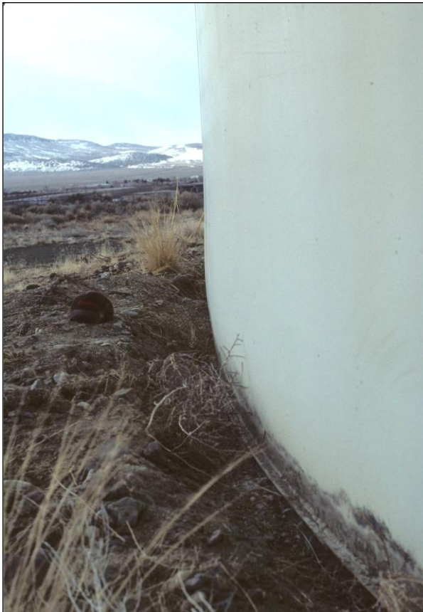
Figures 12, 13, and 14. Water tank has shifted and developed a bulge at its base (“elephant’s foot”) on one side (lower left). The shifted base is shown on the lower right with a baseball cap for scale.
