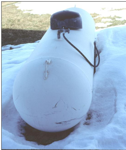
Figure 1. The tank has a flexible hose but is leaning on a rigid upright pipe feeder (left). Figure 2. Propane tank that shifted on its blocks by a few centimeters (about 1 inch) from the shaking (right).
