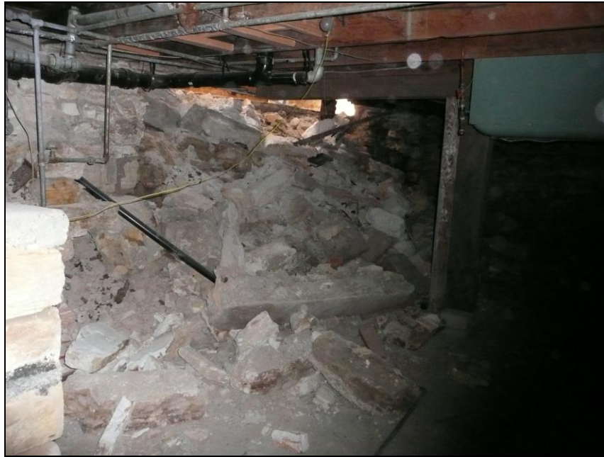
Figure 7. Collapse of the rubble-rock foundation and bottom of the rock wall into the basement of the rock house. Photo by Glen Palmer
