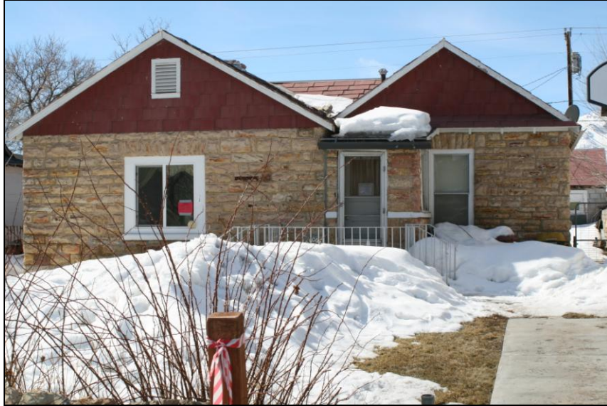
Figure 2. Rock wall house that was damaged beyond repair. The red “unsafe to occupy” posting can be seen in the window.
