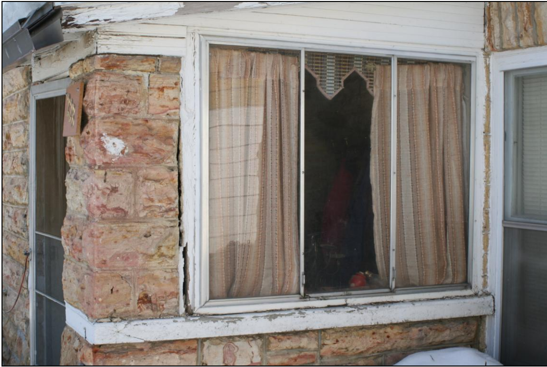
Figure 4. Shaking crack formed where the window frame was separated from the rock cladding in the rock-veneered house. Note the window was not broken.
