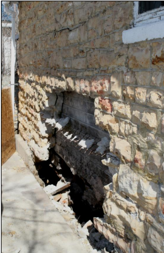
Figures 5 and 6. Figure 5 on the left shows an area where the rock house foundation collapsed sending rocks from the veneer into the basement. Figure 6 on the right shows a close-up view of the iron mesh used in the rock walls and some dry rot near the bottom of the wall.
