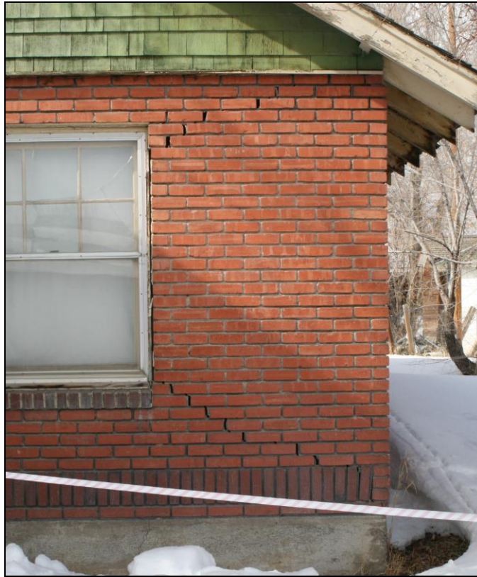
Figure 8. Damaged brick house. Large X-shaking fractures emanate from the corners of the window extending to the corners of the house; the window is broken with a partial X-fracture as well. The fate of this house was still unknown, but similar brick houses with cracking damage have been repaired and continue to be occupied.
