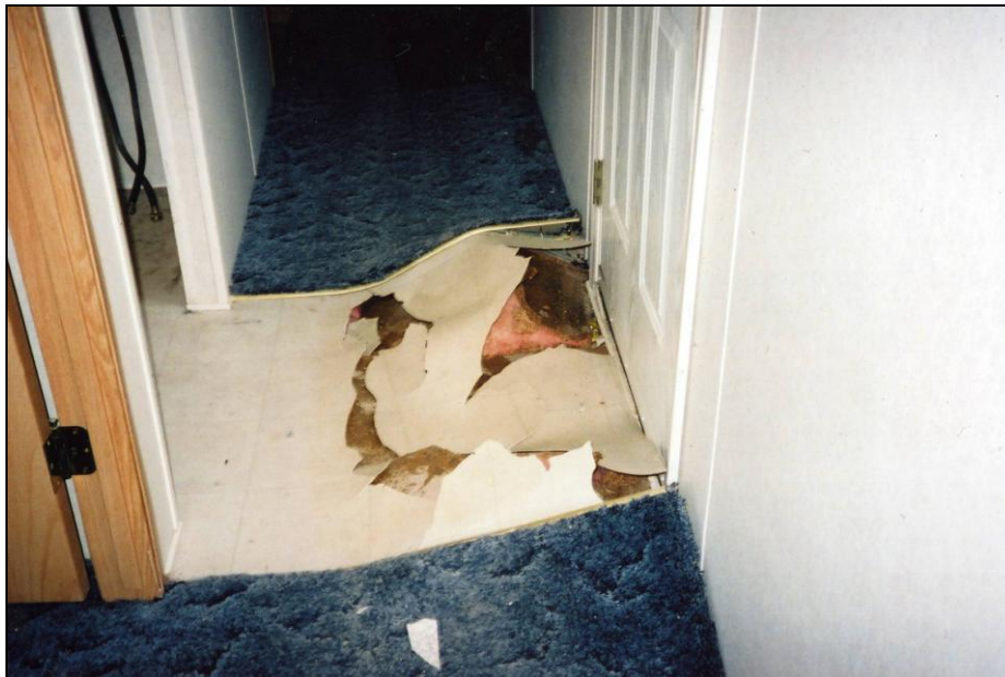
Figure 11. Support jack penetrating the floor after the home was knocked off its foundation. Photo by Bonnie Stark
