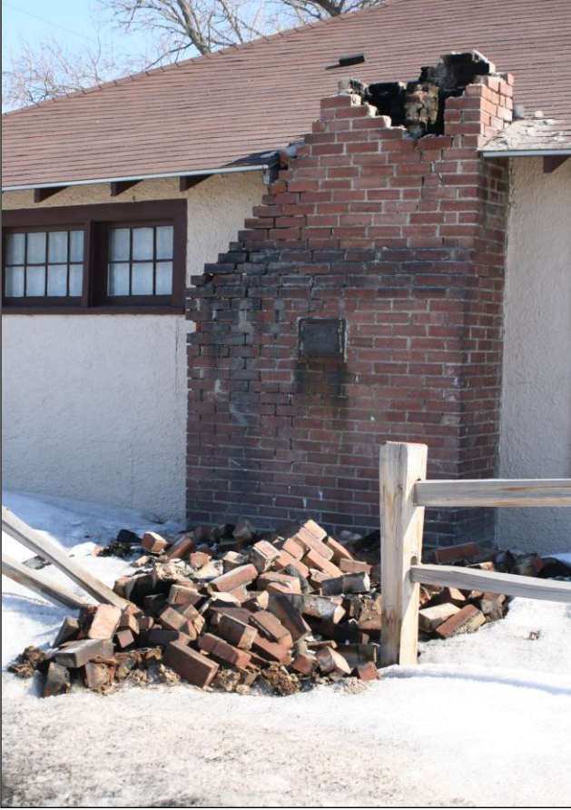
Figure 13. The fallen upper part of a chimney that broke near the roof line.
