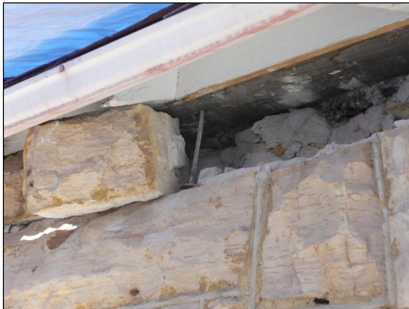
Figure 3. Upper part of rock wall where blocks were dislodged at the roof line. Photo by Glen Palmer
