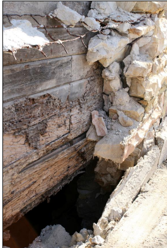
Figures 5 and 6. Figure 5 on the left shows an area where the rock house foundation collapsed sending rocks from the veneer into the basement. Figure 6 on the right shows a close-up view of the iron mesh used in the rock walls and some dry rot near the bottom of the wall.
