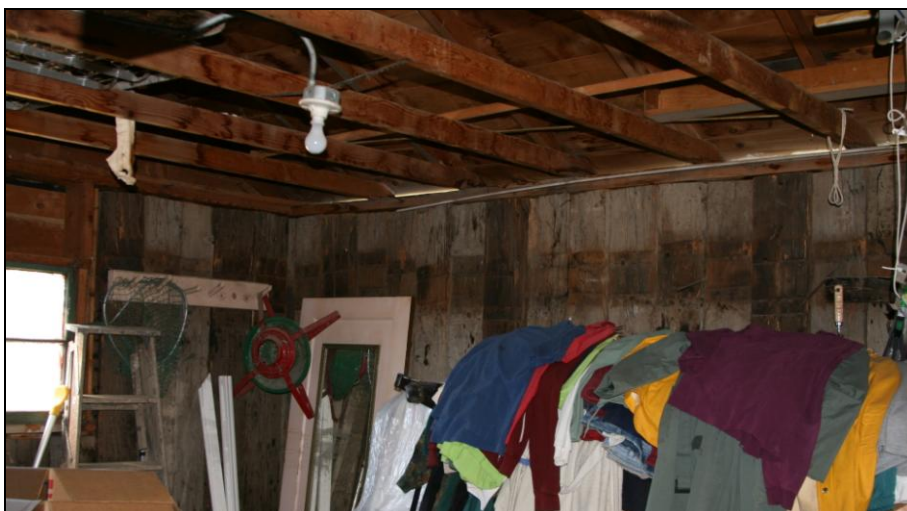
Figure 1. Railroad-tie house construction. The ties were placed vertically to make up the walls of this garage. This house was in the Modified Mercalli Intensity VII area but barely had a crack in it from the earthquake.
