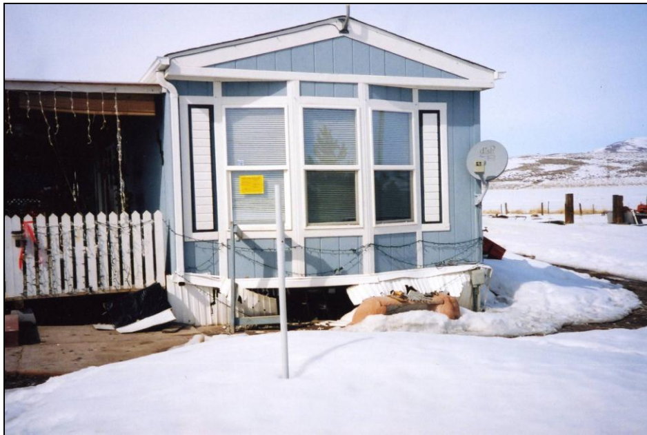
Figure 9. Manufactured home that was knocked off its jacks and destroyed. Photo by Bonnie Stark
