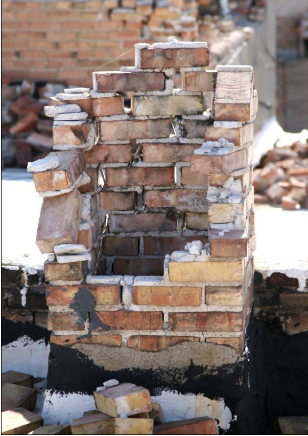
Figure 12. Shattered and fallen chimney from the Bargain Barn roof in old town; the chimney is disintegrating in place.
