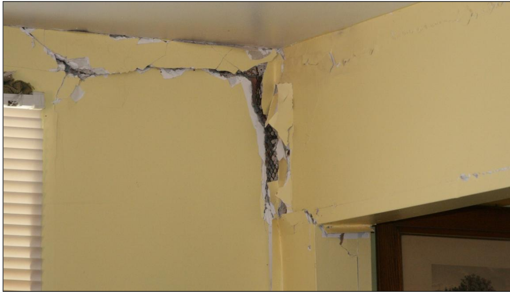
Figure 110. Severe cracking of sheetrock in the upper part of the second story of the El Rancho Hotel.
