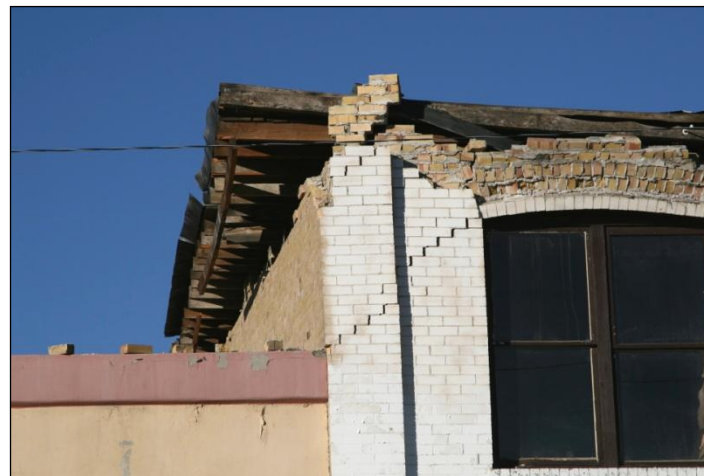
Figure 143. The brick arch over the upper window has lost the outer layer of bricks and is tilted out-of-plane. One of the major cracks comes up to its eastern base.
