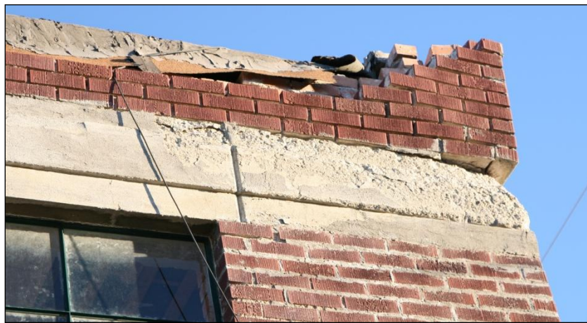
Figure 181. Upper southwest corner of the Wells Chalet. A short brick wall sat on top of the concrete beam and was capped by a two-rebar reinforced bond beam. This bond beam was thrown off the western side of the building by the earthquake, clearing the sidewalk, and fell on the car, crushing it.
