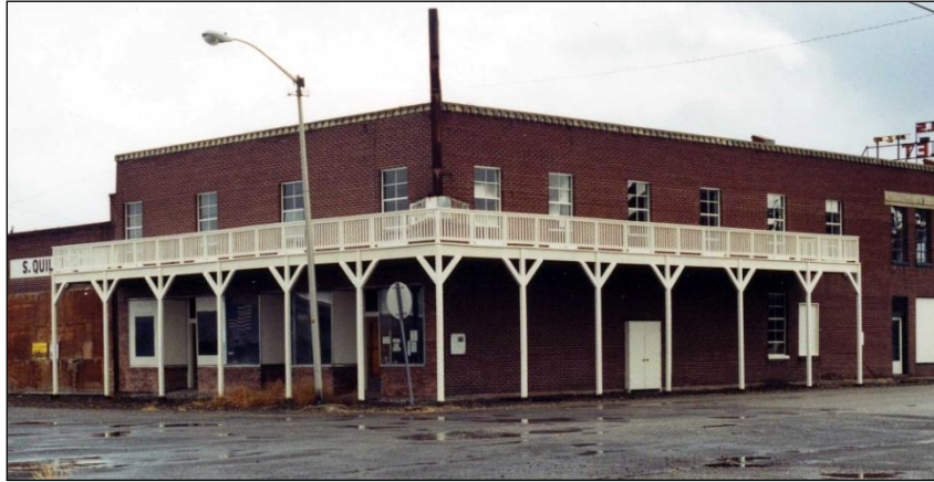
Figure 61. The Bullshead Saloon before the earthquake. The front is on the left side and the western side is on the right. The balcony surrounds the building and the bond beam can be seen on the top of the wall. Photograph by Sue Chapman.
