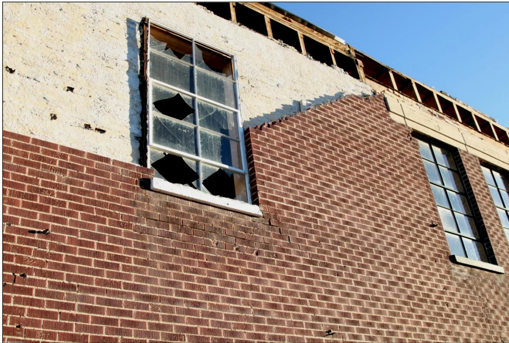
Figure 179. Southern part of the Bullshead Saloon (left) and northern part of the Wells Chalet (to right with the concrete beam near the top). The Wells Chalet appears to be a more rigid building (URM/concrete) versus the more flexible wood-framed Bullshead Saloon. The butted contact also apparently stiffened the edge of the Bullshead.
