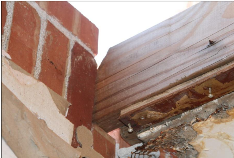
Figure 107. The diagonal cut is a “fire cut” made so the cut would burn faster if there was a fire and drop the interior of the building without damaging the walls. With a longer duration of shaking, these connections might have started to fail.
