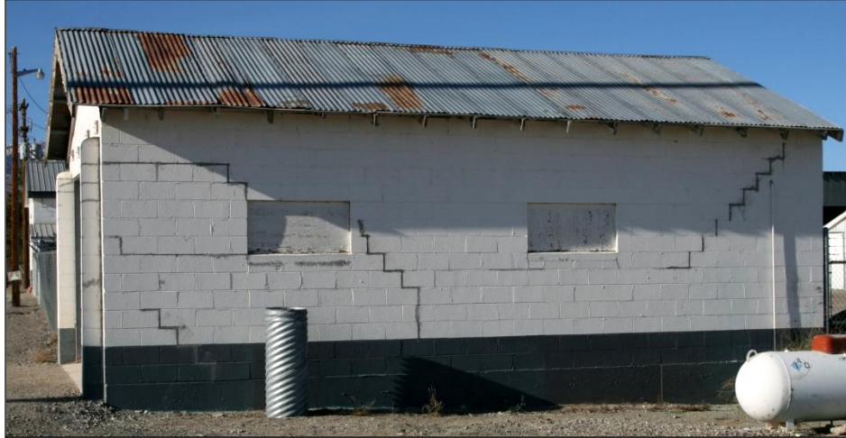
Figure 41. Patched cracks in another concrete block masonry building at the Elko County Highway Department compound; northern wall is shown.
