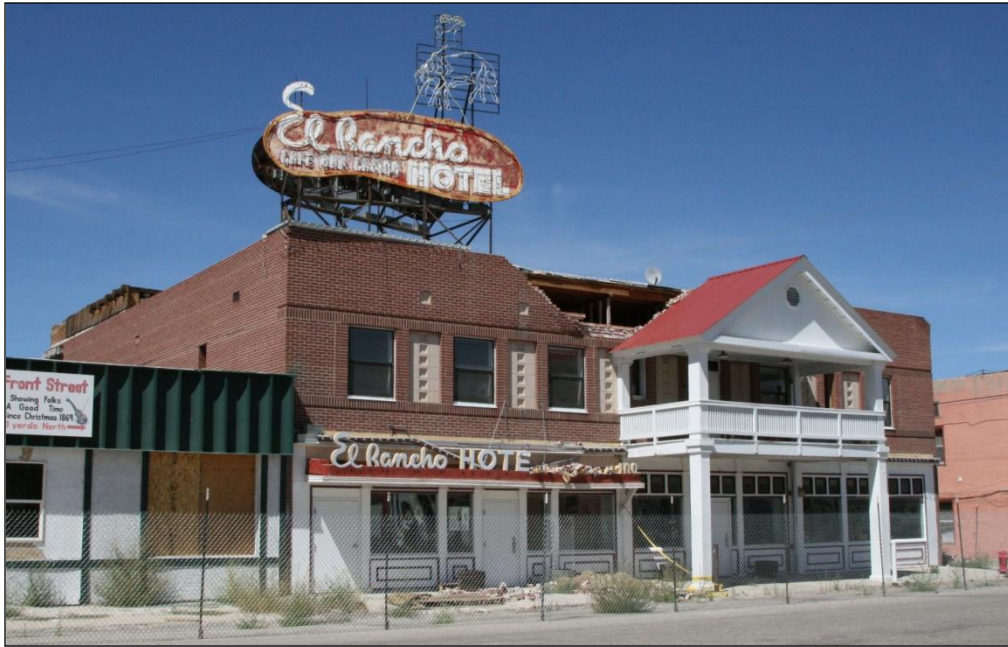
Figure 100. Earthquake-damaged front of the El Rancho Hotel.
