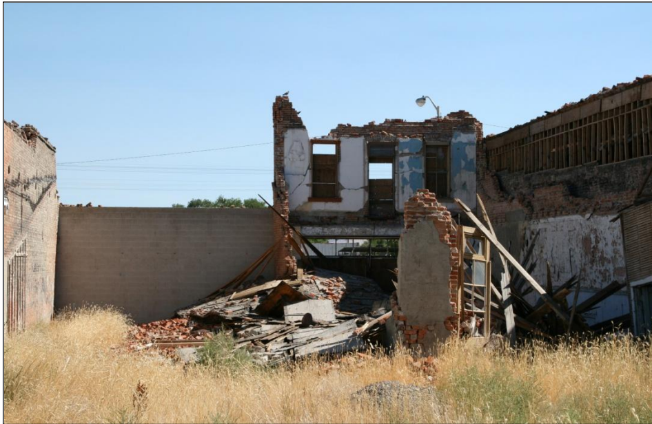
Figure 167. Collapsed San Marin Hotel viewed from the back. The western wall has collapsed bringing down the second story and roof. Only the lower corners remain of the western wall. Displacement may have been relatively limited at the more rigid front of the building, which is buttressed by the concrete block wall. The opposite remaining corner is badly cracked.
