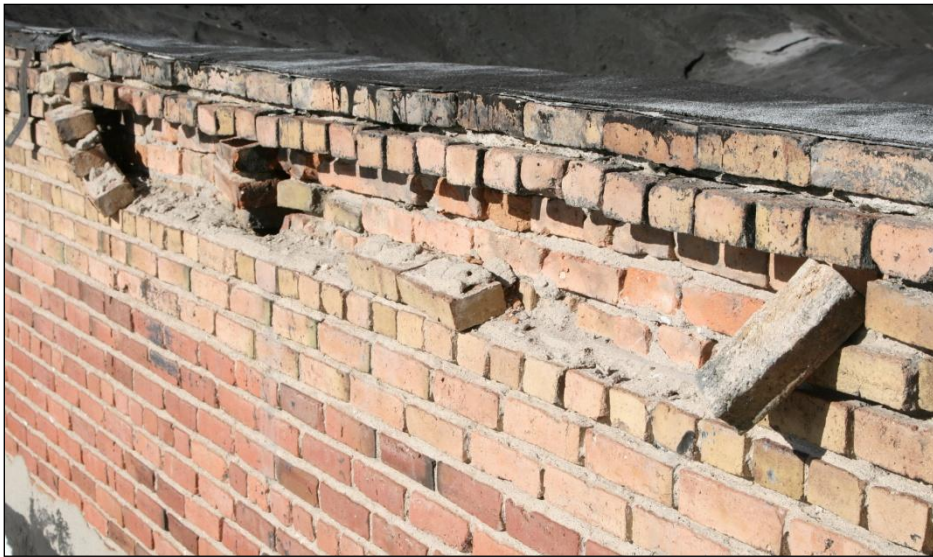
Figure 161. Area where bricks have fallen out near the roof on a side wall. The mortar lies pulverized around the remaining bricks.
