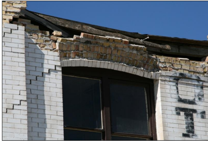
Figure 142. Eastern side of the front of the building showing fallen (and pushed off?) parapet on the eastern side of the building, the roof overhanging in the front, and a large crack coming up diagonally from the adjacent support of the Mint Saloon's false front.
