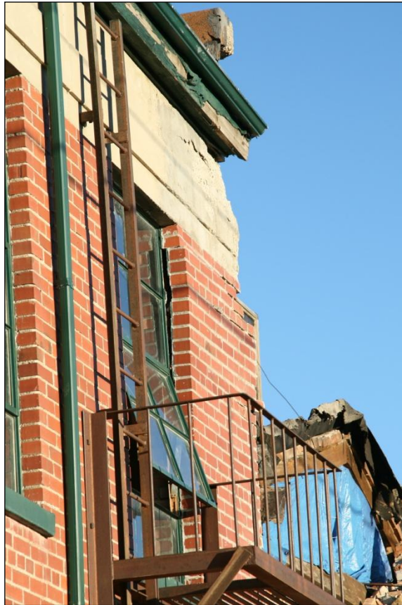
Figure 178. Delaminating brick wall below the eastern end of the concrete beam and next to the window.
