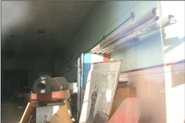
Figure 92. In the photograph to the right showing the inside of the Eagle Club, the pipes on the cabinet surprisingly stayed up during the earthquake even though they were free to roll around.
