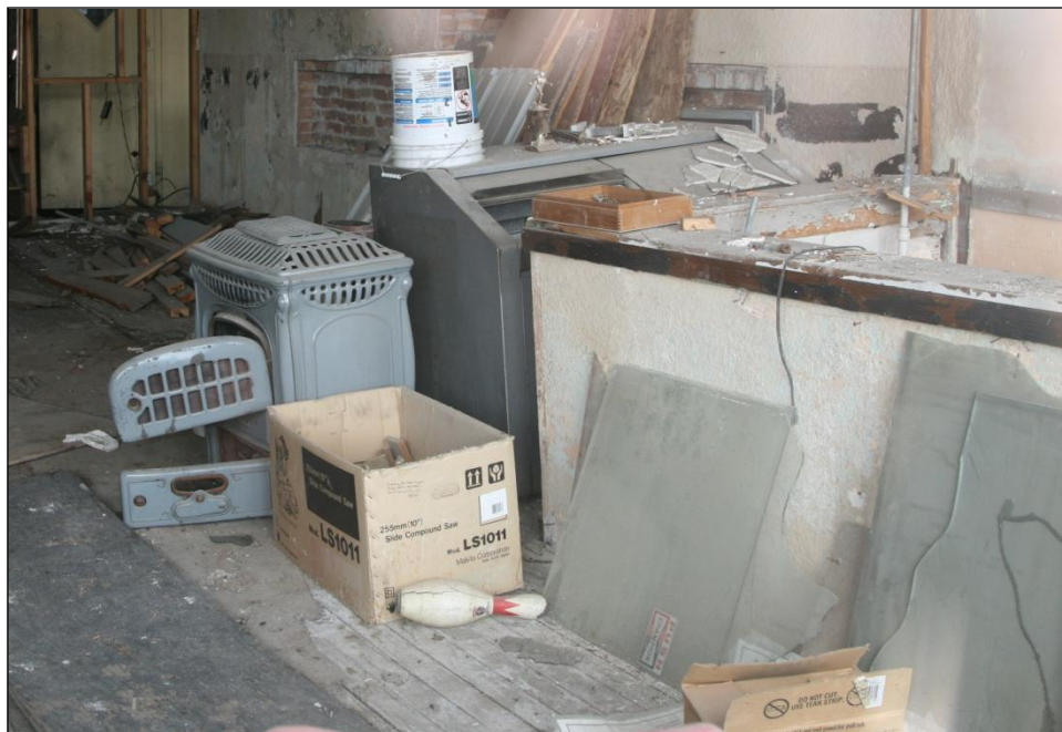
Figure 136. Interior of Murphy's Bar showing sheets of leaning glass that are unbroken by the earthquake. A cut in the wall in the background shows the unreinforced brick construction.
