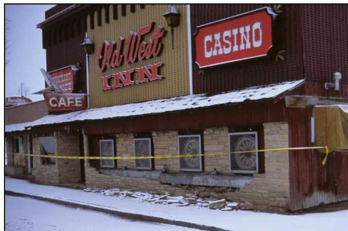
Figure 150. Front of the Old West Inn. Rocks forming a front façade were knocked down.
