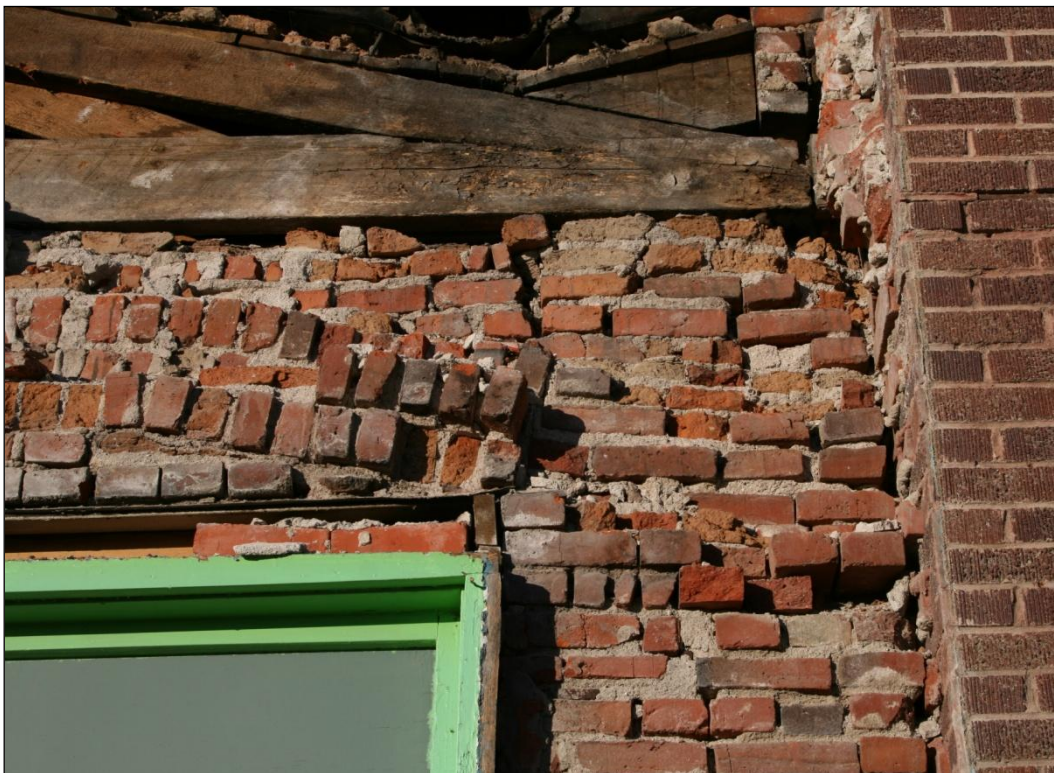
Figure 75. Detail of the front wall. Several of the vertical contacts between bricks lack mortar.
