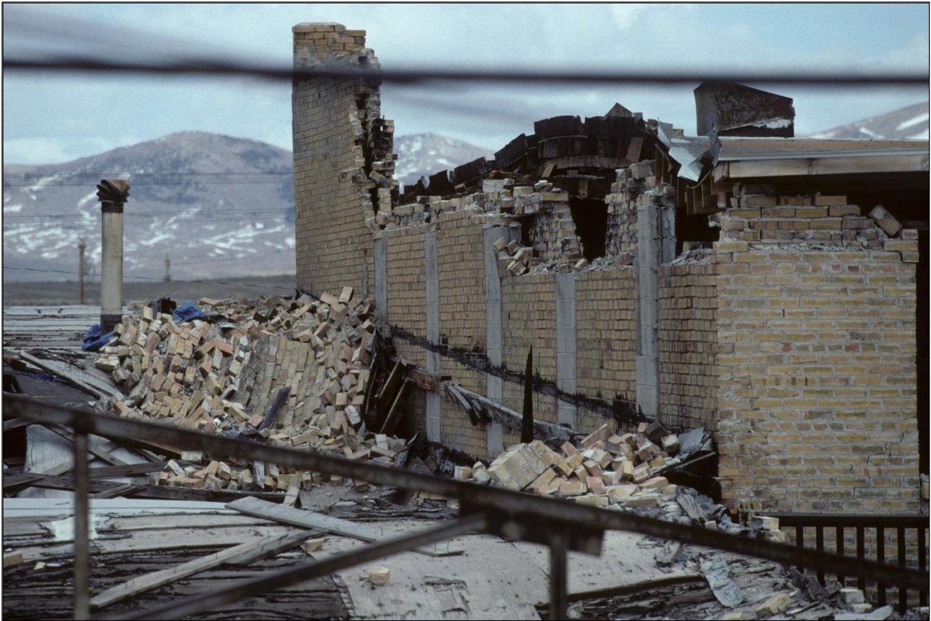
Figure 15. Failure of the parapet and upper wall of the eastern side of the Nevada Hotel. The roof failure of Murphy's Bar was pre-existing from snow damage. The wall is laid down on the roof as if it fell out en masse. Even though over 25 courses of bricks fell on Murphy's Bar, where the roof was in place, it stayed up. The bricks fell a distance of about half a story. The Nevada Hotel and Murphy's Bar share a common wall.
