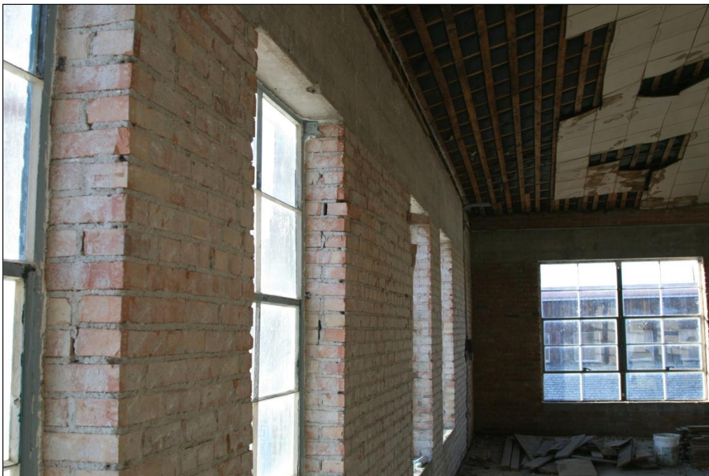
Figure 177. Damage to the second-story southern wall of the Wells Chalet below the concrete beam. Interior picture showing cracking and some displaced bricks of the wall in the center of the picture.
