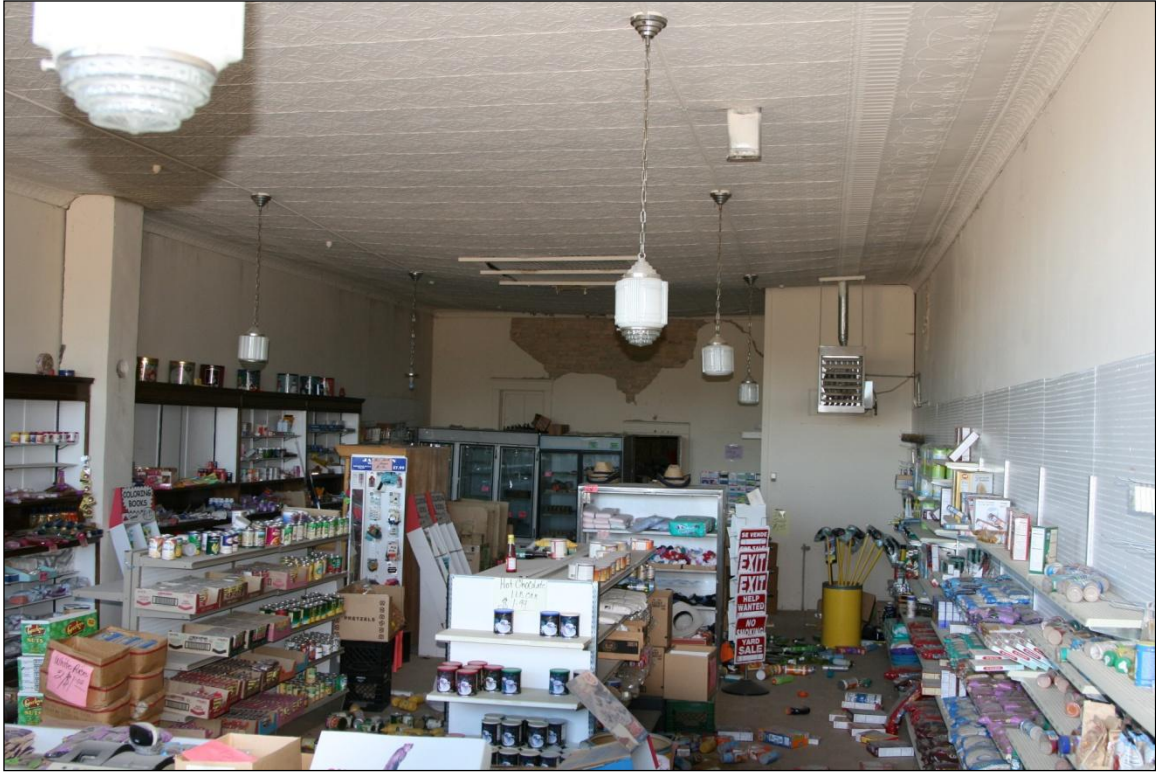
Figures 55. Interior nonstructural damage in the Bargain Barn. Although several items fell to the floor, most remained on the shelves. Ceiling tiles remain in place, hanging lamps and the suspended metal heating unit all are still in place.
