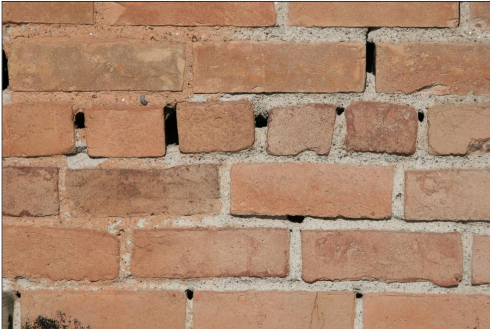
Figure 159. Weather-worn mortar on the top of the mercantile. This weaker mortar may have contributed to some of the dismemberment damage to the back corner.
