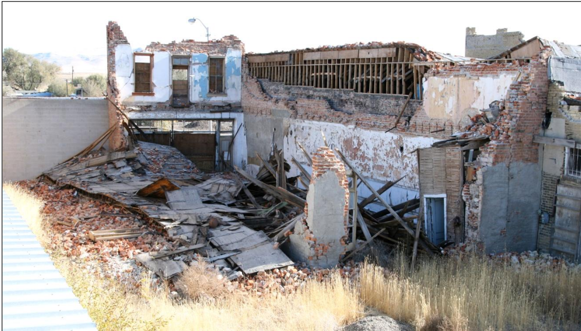
Figure 5. Collapsed San Marin Hotel, viewed from the back. The western wall (left side) has collapsed bringing down the second story floor and the roof. Only the lower corners remain of the western wall. Displacement may have been limited in the more rigid front of the building which buttressed by a concrete block wall and has a solid concrete header beam over the open window front. The opposite remaining corner is badly cracked and rear of the building is reported to have partially collapsed before the earthquake.
