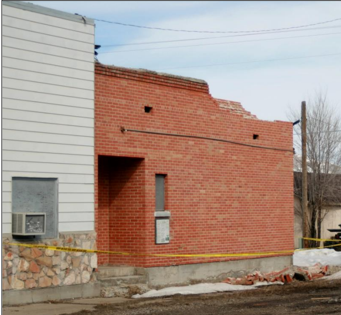
Figure 86. Fallen bricks and crowning bond beam from the parapet on the Constable Powers Building.
