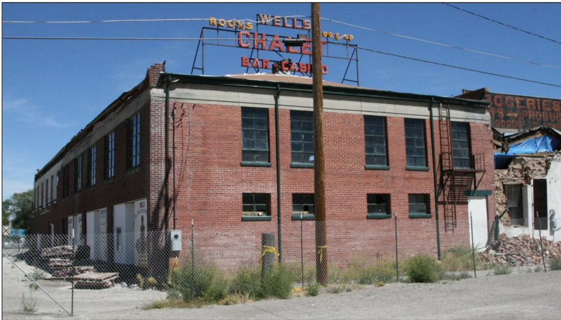
Figure 174. The Wells Chalet building, viewed towards the northeast showing the southern wall (center) and the shaded western wall (left). The building has unreinforced brick walls with large concrete beams at the top, partly to carry large steel trusses that hold up the roof over the second story dance floor. The Wells Chalet building appears to have shaken less than the adjacent Bullshead Saloon (seen farther down the block in the shadows with the fallen veneer) during the earthquake because the veneer on the west side of the chalet has not broken up and fallen away; this may be attributed to the stabilizing effect of the concrete beam, but note that nearly all of the windows are unbroken in the Wells Chalet as well.
