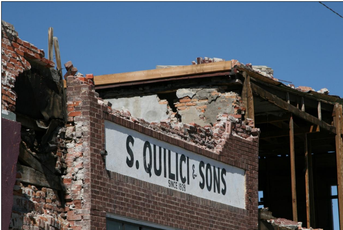
Figure 154. Failed parapet at the front of Quilici and Sons Mercantile.
