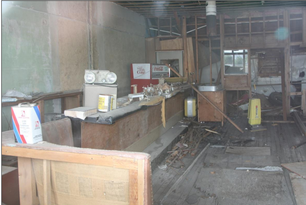
Figure 135. Inside the front of Murphy's Bar. Note the stovepipe hanging down just to the right of center near the top. This is the same stove pipe visible at the roof in figure 134 that is surrounded with bricks. No bricks penetrated and there was relatively little seismic disturbance to the interior.
