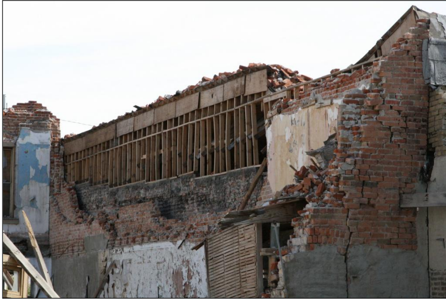
Figure 93. The western wall of the Eagle Club. Although the wall has not failed, the adjacent wall of the San Marin Hotel failed, exposing the top of the Eagle Club to the weather.
