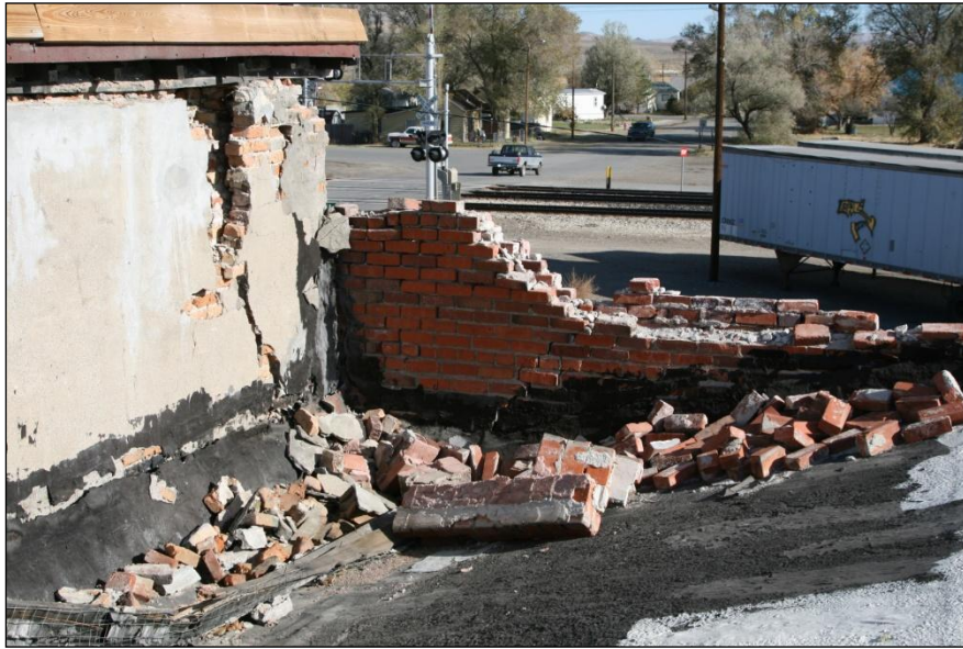
Figures 157a. Fallen bricks from the front of the mercantile and the Bullshead Saloon in the front corner of the store. This corner is where some of the roof and ceiling joist connections failed.
