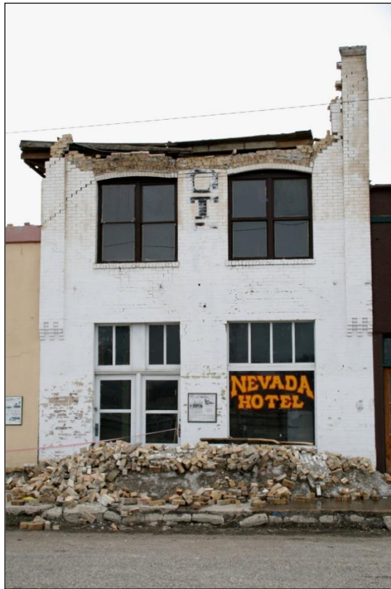
Figure 8. Earthquake damage to the Nevada Hotel. Fallen bricks from the front parapet and upper part of the wall are visible, as is the displaced roof. On the right (west) side of the Nevada Hotel is Murphy's Bar and on the left side is the Mint Saloon. Note that despite the damage to the hotel, the windows were not broken.
