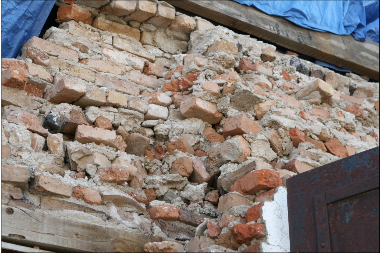
Figure 22. Rubble infill (basically unlaid brick) in the unreinforced masonry wall at the back of the Quilici Market. This was covered by laid bricks and stucco (lower right center).
