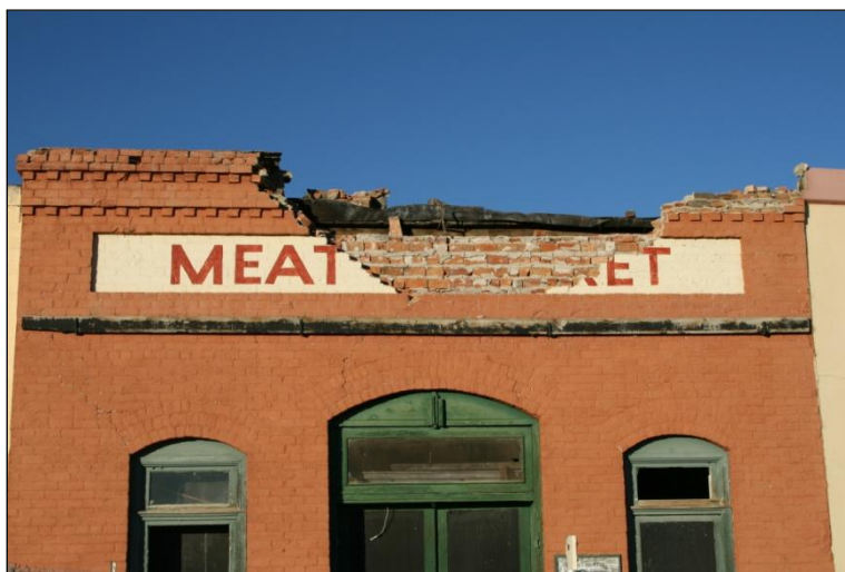
Figure 122. Area of fallen bricks from the upper wall and parapet of the Meat Market.
