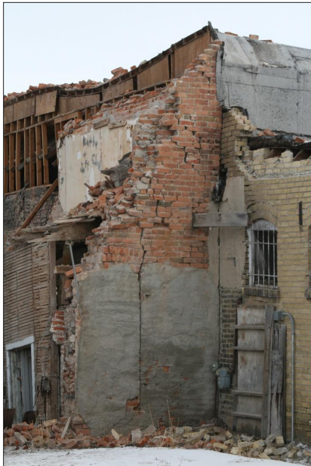
Figure 94. Corner between the back wall of the San Marin Hotel and the Eagle Club. An inactive gas regulator was threatened by falling bricks (shown to the right and below). Active utilities need to be protected from falling bricks around unreinforced brick/masonry buildings, possibly with a protective cage.
