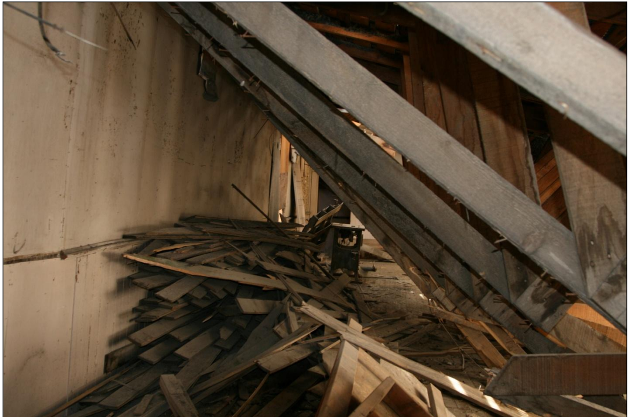
Figure 10. Inside the Mint Saloon with the collapsed roof system still hinged on the eastern wall.
