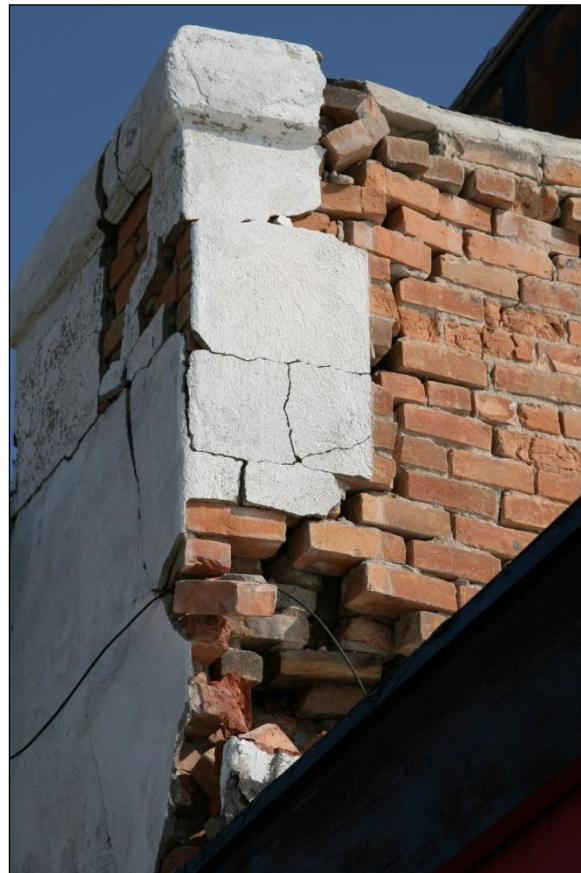
Figure 163. Damage to the southeastern corner of the store.
