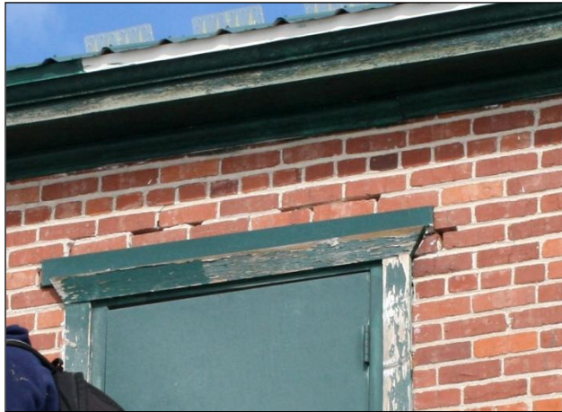
Figure 80. Disrupted bricks above the second-story fire escape of City Hall.
