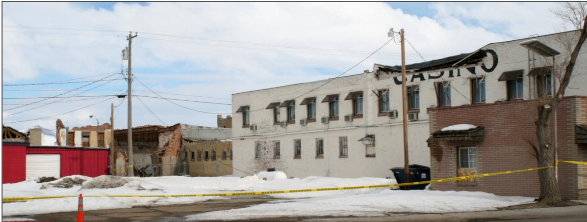
Figure 153. Contrast between the limited damage to the two-story Old West Inn (to the right) and the shell of the collapsed San Marin Hotel (next to the red building on the left). The view is to the northeast.
