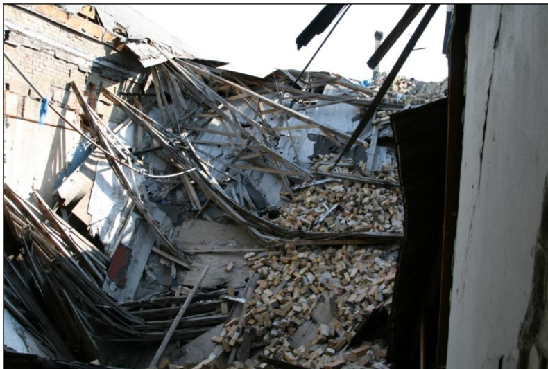
Figure 134. Bricks from the Nevada Hotel fell onto the roof of Murphy's Bar which had previously collapsed from snow. Bricks can be seen around the stove pipe on the uncollapsed part of the roof indicating that the roof was able to handle the weight of the bricks.
