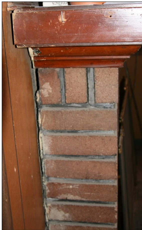
Figure 81. Displaced fireplace in Wells City Hall; this can be seen in the crack between the upper part of the fireplace and the wall.
