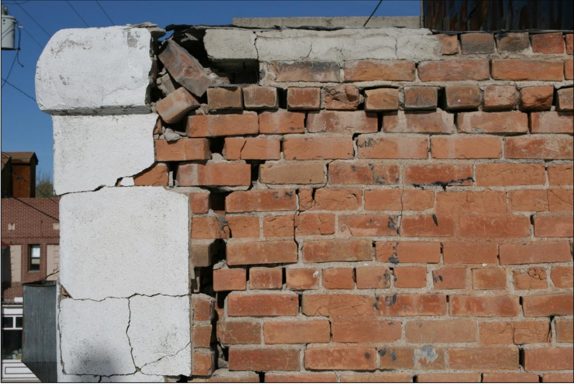
Figure 160. Rear of Quilici Market showing the façade breaking away from the building. Note eroded mortar.
