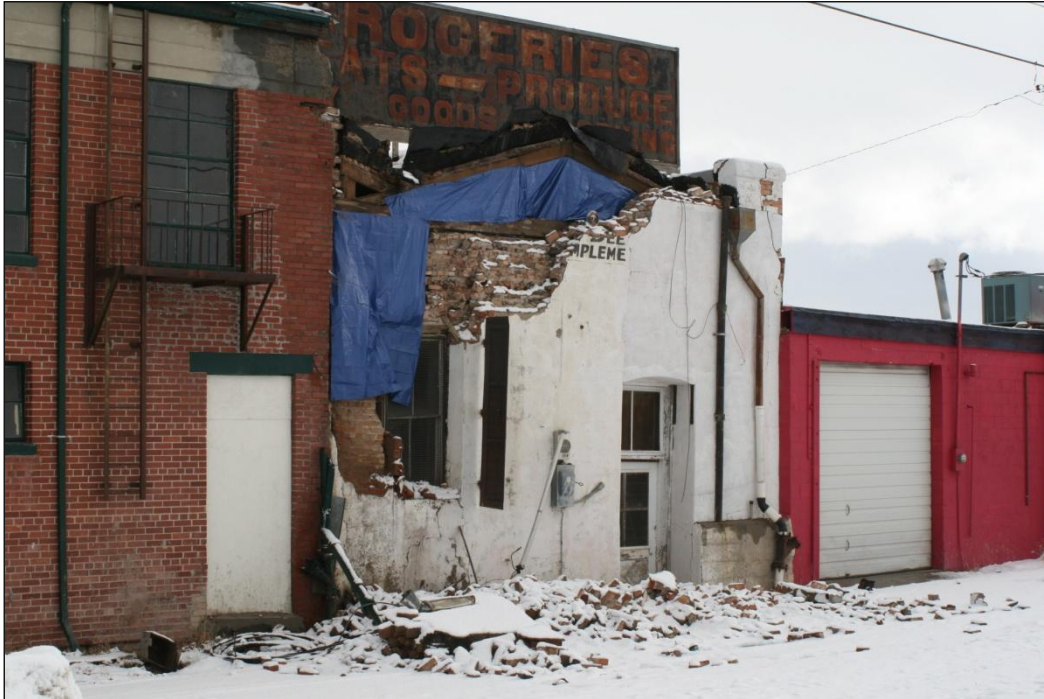
Figure 162. The Quilici and Sons Mercantile showing failed rear parapet, gable end, and wall. More bricks have fallen out of the western side of the back than the eastern side.
