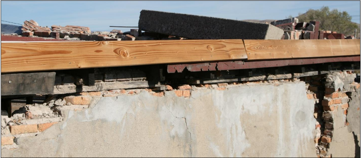
Figure 71. Eastern wall of the Bullshead Saloon. Contact between the roof and the wall. The roof is detached and is carried by the wood frame.
