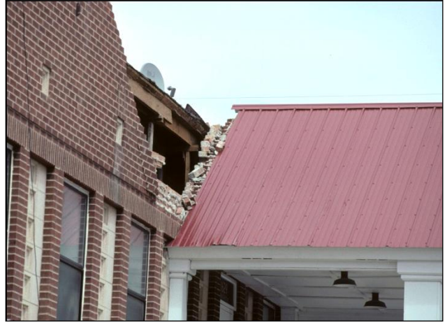
Figure 102. Close-up of upper wall shown in figure 101.
