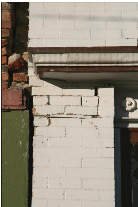
Figure 54. Closer view of the column in figure 53. This front column was pounded and displaced about 4 cm to the west over about four courses of bricks.
