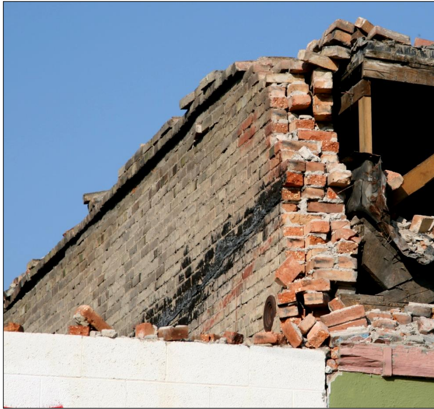
Figure 115. Damage to the eastern wall of the Goble Market has exposed its construction. A later study of the broken wall revealed the cross course bricks that tie the wall together. These appear to be on end along the side of the wall. This is a three-wythe-wide wall. There were also some widely spaced bolts holding the wall to the structure.
