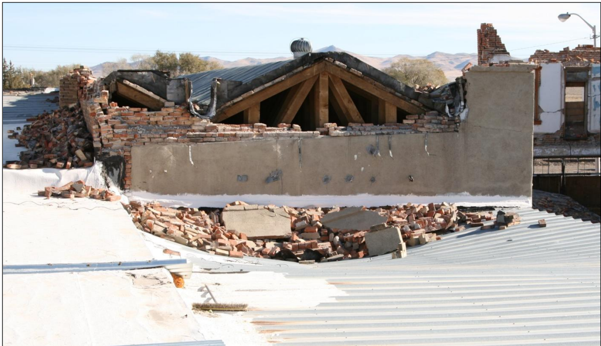
Figure 121. Failed rear gable and western parapet of the Goble Market. The brick wall was caught by the adjacent metal roof, which partially collapsed.
