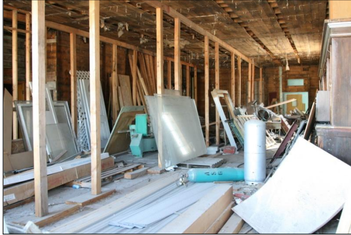
Figure 33. Interior of the Bullshead Bar showing the wood-frame structure. There are new wood braces (pre-earthquake) to help secure the building during construction. Note the leaning glass and other items on the first floor that did not topple or break. The wood reinforcing frame may have helped to keep the building from collapsing during the earthquake.
