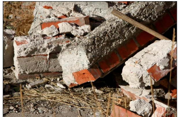
Figure 89. Part of the crowning bond beam that fell from the Constable Powers Building.
