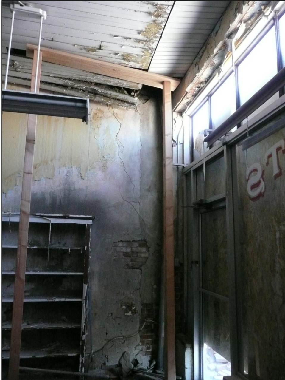
Figure 164. Interior of the Quilici and Sons Mercantile showing the temporary support where roof joists failed. This is directly below the corner shown in figure 157a and 157b. Photo by Glen Palmer.
