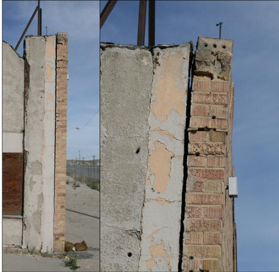
Figure 20. Separation and outward tilt of front wall of the Progress Building. This building has since been demolished.
