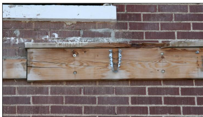
Figure 70. Hanger that held the building side of the balcony up.
