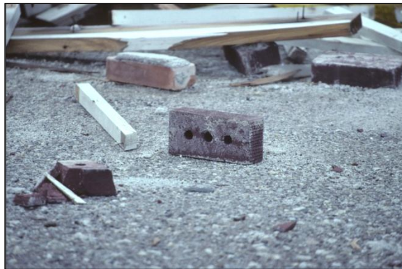
Figure 66. A brick from the upper part of the veneer on the Bullshead Saloon showing small holes for the mortar to stick into them and give the wall some lateral strength. Cracks seen in figure 65 that cross both types of bricks do not show distinct differences in character.
