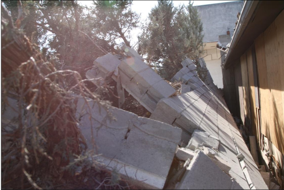
Figure 43. Failure of a concrete block wall away from the structure at the Ranch House Casino. There were a few vertical reinforcing pieces of rebar in the wall.
