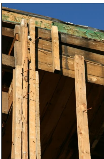
Figure 64. Detail of the upper part of the front of the Bullshead Saloon showing the wood-frame structure and nails that were used to tie the brick veneer to the building.
