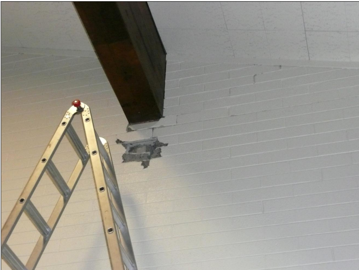
Figure 44. Damage to concrete blocks under a large glulam support beam in the Wells Ward LDS church. A column of concrete should have been poured under the beam, but the blocks were only partially filled with concrete. Photograph by Glen Palmer.
