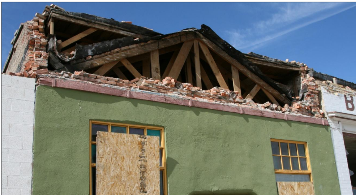
Figure 114. Damaged gable front of the Goble Market.
