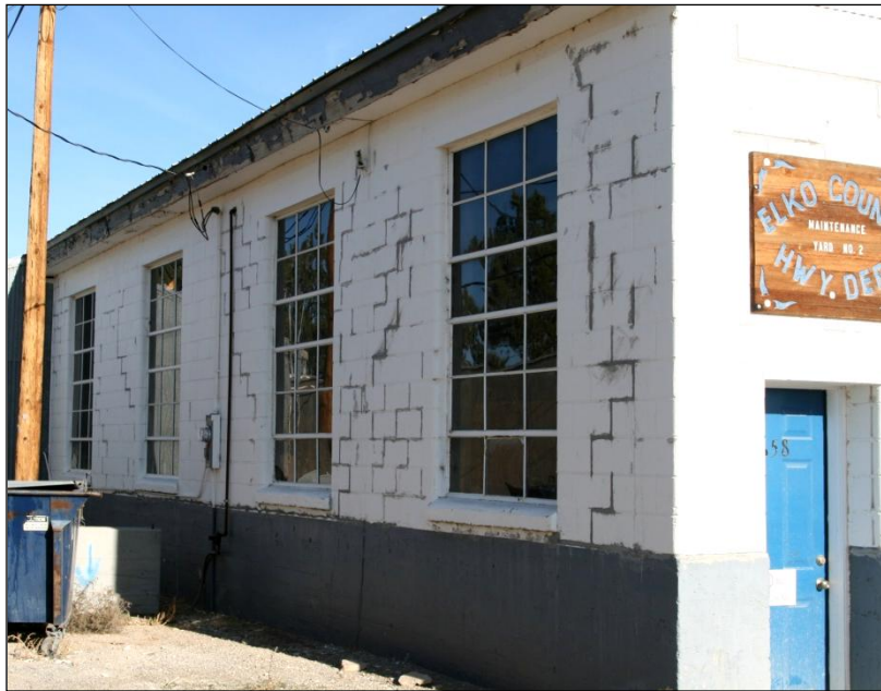
Figure 40. Southern side of the same building shown in figure 39, also showing patched cracks.
