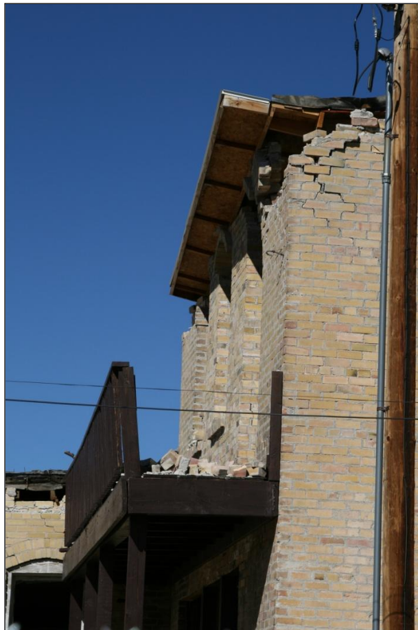
Figure 48. The rear Nevada Hotel balcony caught every brick falling from the back of this severely damaged building.
