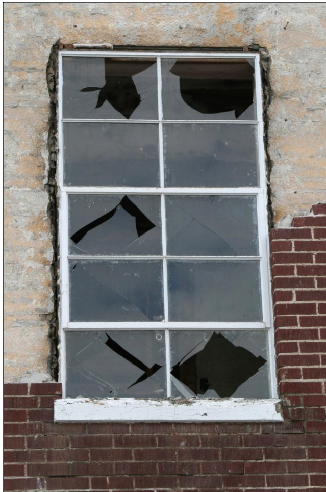
Figure 69. Broken window on the second story of the western wall that shows X-fractures from the back-and-forth distortion of the window.
