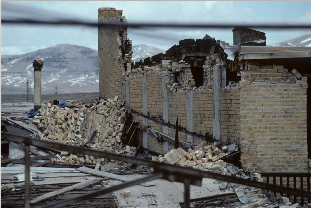
Figure 149. Collapsed western wall of the Nevada Hotel. Concrete block columns can be seen that extended up from the first story ceiling level half way up the wall in the front and relatively higher in the back part of the wall, where the parapet was lower. Many of the bricks that have fallen on Murphy's Bar around the stovepipe are in order and seem to have fallen out as a toppled unit.
