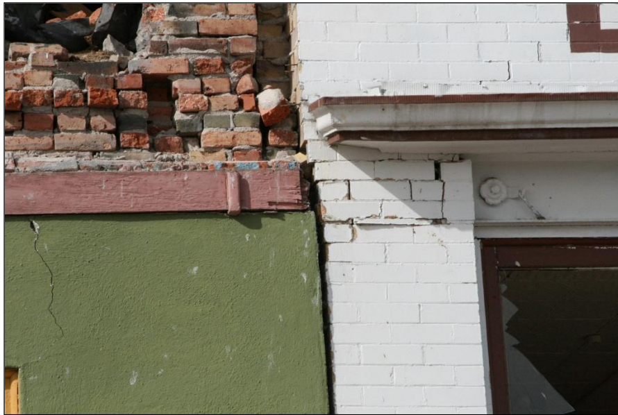
Figure 24. Building pounding damage between the Goble Market and the Bargain Barn. The white column of the Bargain Barn is displaced about 4 cm over four courses of bricks.
