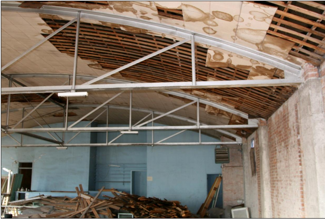
Figure 183. Interior of the second floor of the Wells Chalet showing roofing, steel roof trusses, concrete columns and in the back corner is the chimney shown in figures 184 and 185.
