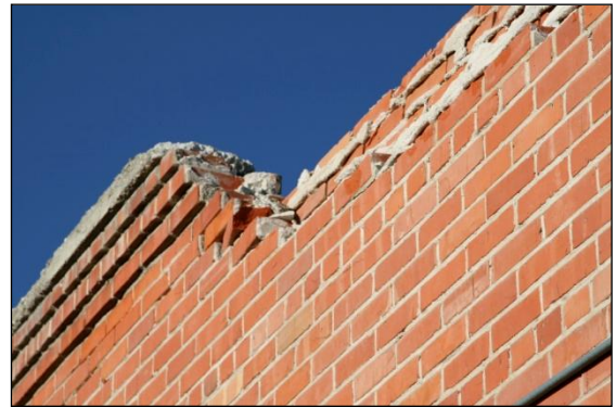
Figure 87. Parapet section that fell out of Constable Powers building.
