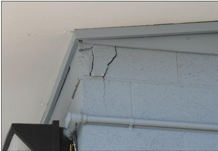
Figure 37. Broken concrete block brick and cracking in the upper corner of a Nevada Department of Transportation garage building in Wells.
