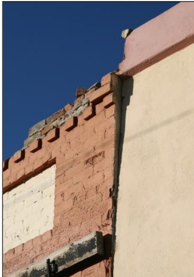
Figure 123. Leaning top of the wall of the Meat Market.
