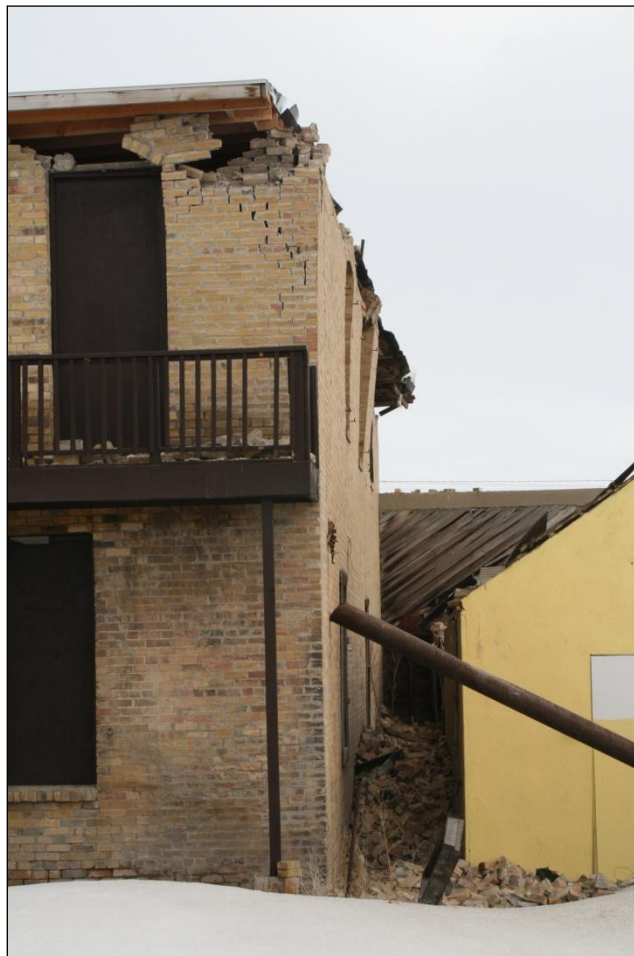
Figure 146. Eastern side of the Nevada Hotel showing rotated roof and out-of-plane parts. The balcony is on the back of the building and caught most of the bricks falling there.
