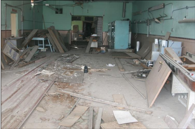
Figure 91. Interior of the Eagle Club showing little earthquake damage and washing machine units in the upper right that did not topple.
