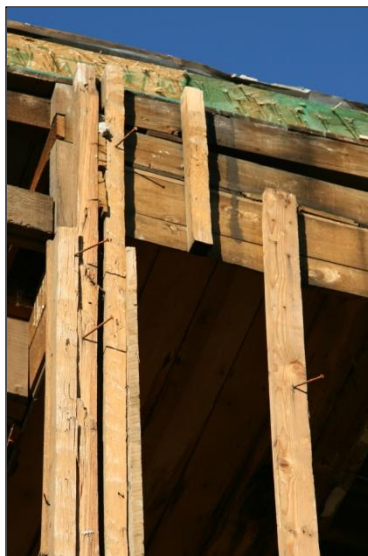
Figure 26. Detail of the upper part of the front of the Bullshead Bar showing the wood frame structure and nails that were used to tie the brick veneer to the building. There were more nails; some were pulled out.
