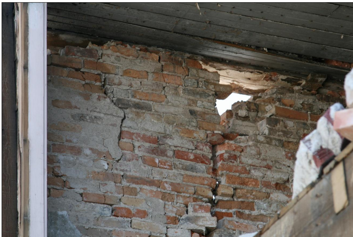
Figure 63. Close-up picture of damage to the eastern wall near the front corner. The wall is cracked, including a large crack that flowers into a hole near the top. The roof is detached from the wall and appears to have moved back-and-forth over it.
