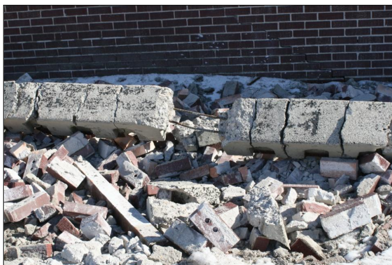
Figure 18. Crowning bond beam section that fell off the Wells Chalet and likely broke up from uneven impact. Rebar in the bond beam can be seen. This is the same bond beam that is shown in figures 17 and 19.
