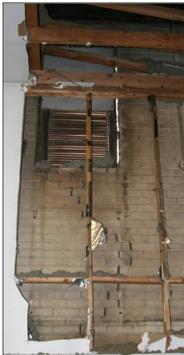
Figure 83. Wall crack shown in Figures 84 and 85 viewed from inside the city shop. There is a wood frame for the interior ceiling and walls.
