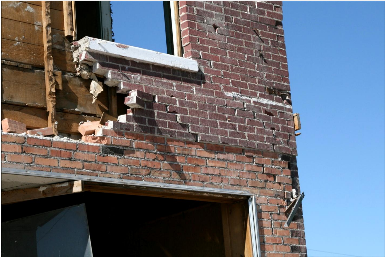
Figure 65. Large X-fractures in the remaining brick veneer on the front of the Bullshead Saloon show the break-up of the façade due to the back-and-forth rocking of the building. The lower, redder bricks are older and are solid, whereas the darker bricks above have small holes in them (figure 66). Both types of bricks fractured similarly.
