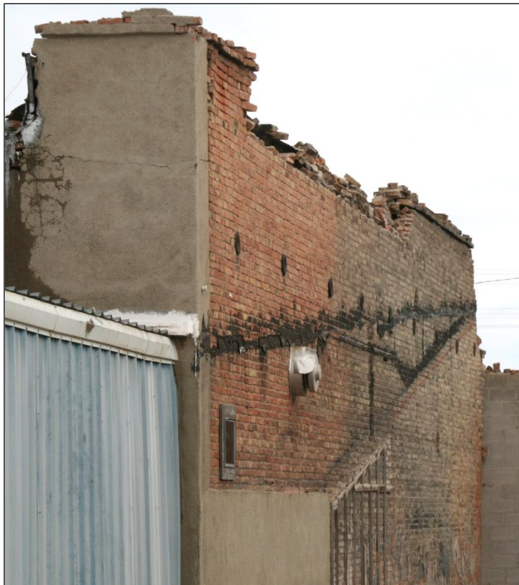
Figure 118. Eastern wall of the Goble Market. Parapet failure of wall and the ends of tie rod anchors are visible.
