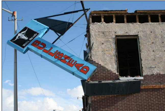
Figure 59. The northeast corner of the earthquake-damaged Bullshead Saloon with its dislodged sign.
