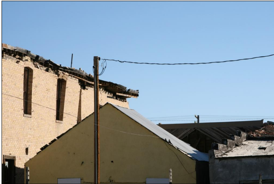
Figure 126. Back of the Mint Saloon showing the remaining part of the roof. A large gap can be seen between this remnant and the front where the roof has collapsed. Bricks from the Nevada Hotel, on the left, collapsed the roof.
