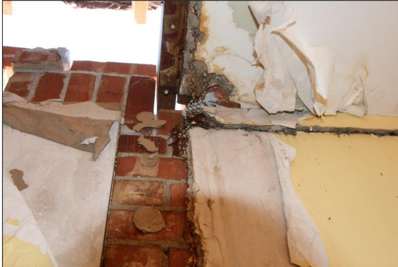
Figure 106. Ceiling joist connection exposed by water damage. The joist is unattached to the wall, but was found to have shifted only a few millimeters in this case, once the shaking had stopped.
