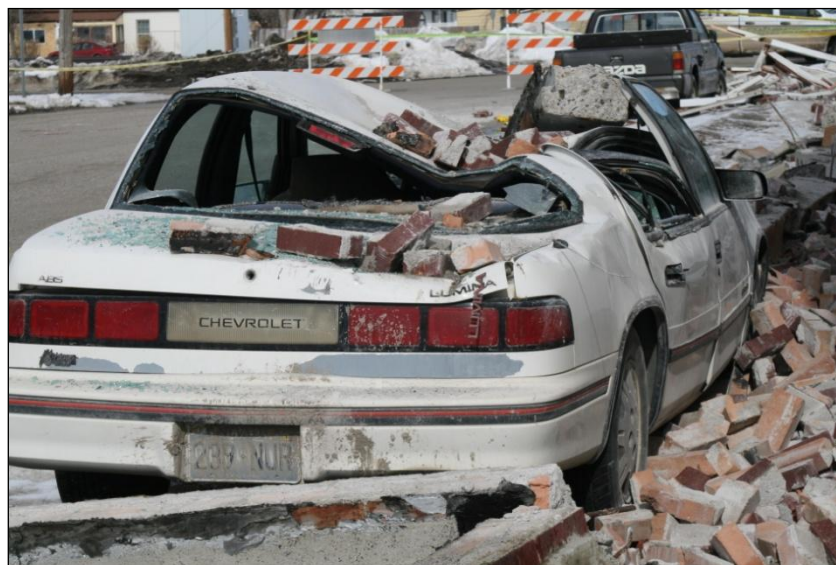
Figure 182. Car crushed by the crowning bond beam that fell from the Wells Chalet. The large bond beam cross section can be seen on the car.
