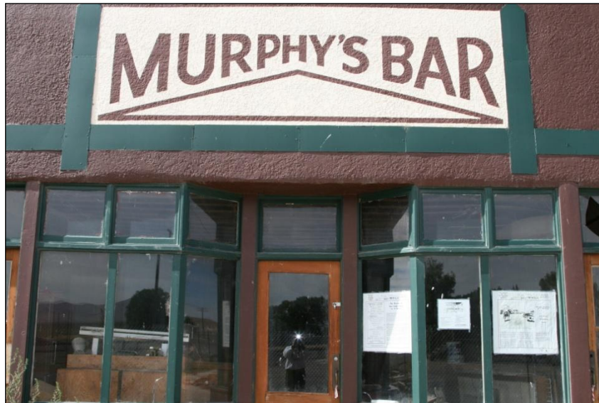
Figure 133. Front of Murphy's Bar. Only a couple of windows were cracked or broken.
