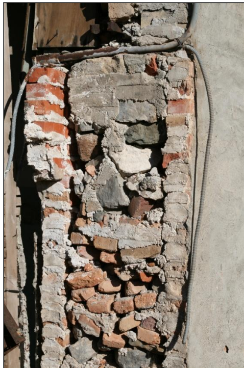
Figure 23. Rubble infill in the unreinforced masonry wall at the back of the San Marin Hotel. There were holes and gaps in this wall large enough to put a man's fist into, and several of the rocks were thrown in with no mortar in between them. The outer courses of laid bricks served as the forms for the rubble infill and hid this kind of construction from outside visual inspections.
