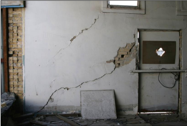
Figure 139a. Large crack inside the back door of Murphy's Bar.
