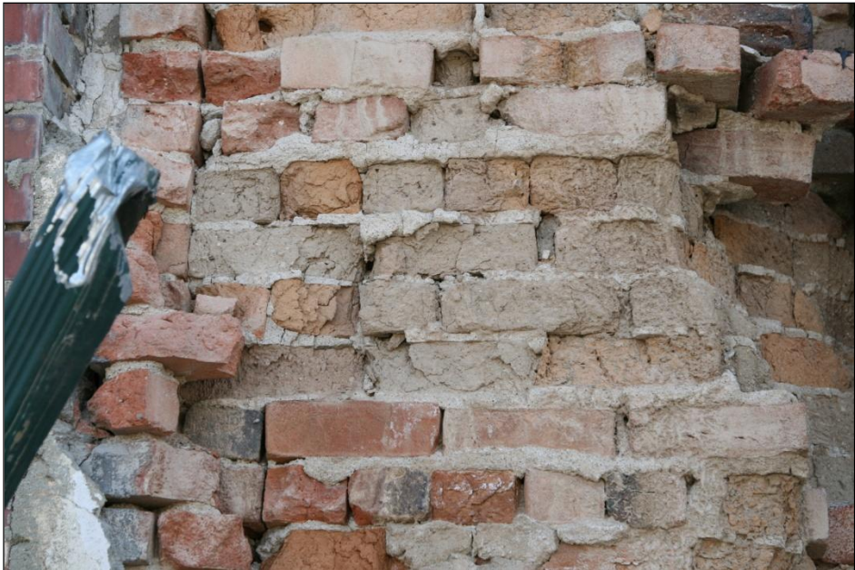
Figure 21. Adobe and unfired bricks in the back wall of the Quillici Market. These were weak elements and were reduced to a pile of dirt when wetted. Notice the course of fired bricks on the far left side of the photo that covered up the unfired bricks.
