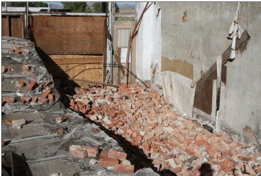
Figure 172. Part of the of the San Marin Hotel first floor not covered by the collapsed second floor and the roof, but completely covered with bricks. The front door (upper center of photo) has fallen bricks on both sides of it.
