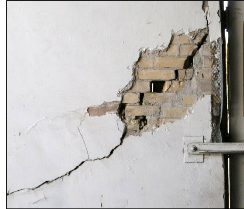
Figure 139b. Close-up view of the large crack inside the back door of Murphy's Bar.
