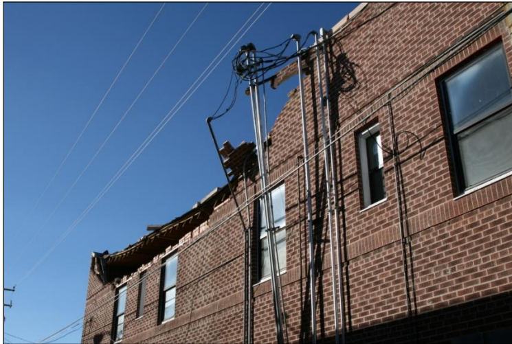
Figure 103. Failure of the upper part of the northern wall. A large section of the wall between the ceiling joists and the roof, including the parapet, fell out and damaged electrical masts to the building.
