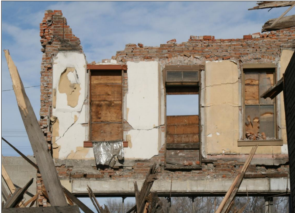
Figure 169. Remaining front of the second story of the San Marin Hotel. Note the concrete beam header for the front which was a relatively coherent part.
