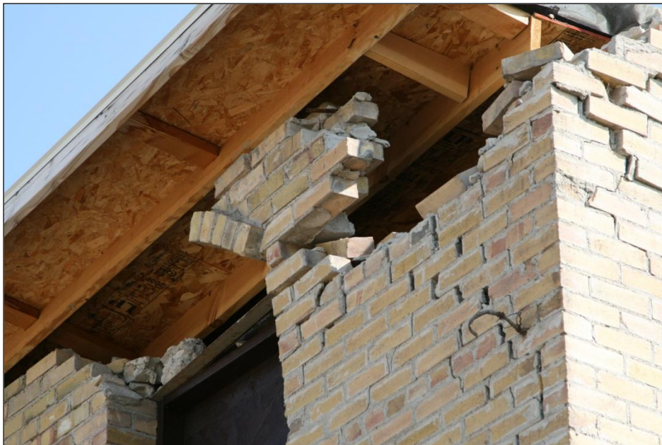
Figure 148. Southeast upper corner of the Nevada Hotel. The corner is badly cracked and is breaking up.
