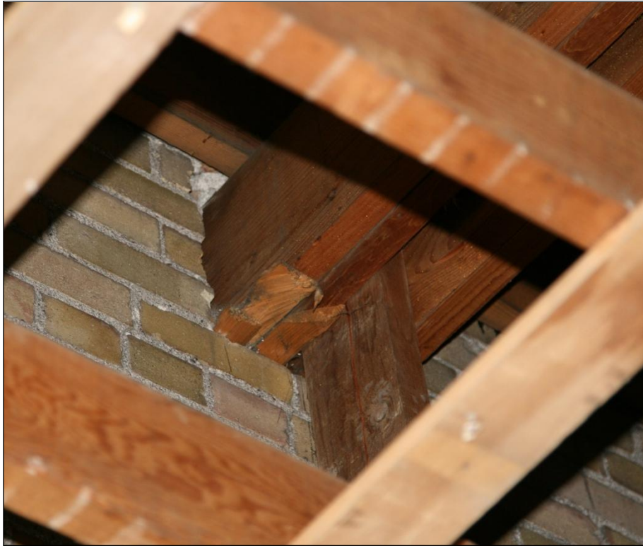
Figure 137. Detail of a roof rafter connection into the common wall of Murphy's Bar and the Nevada Hotel.
