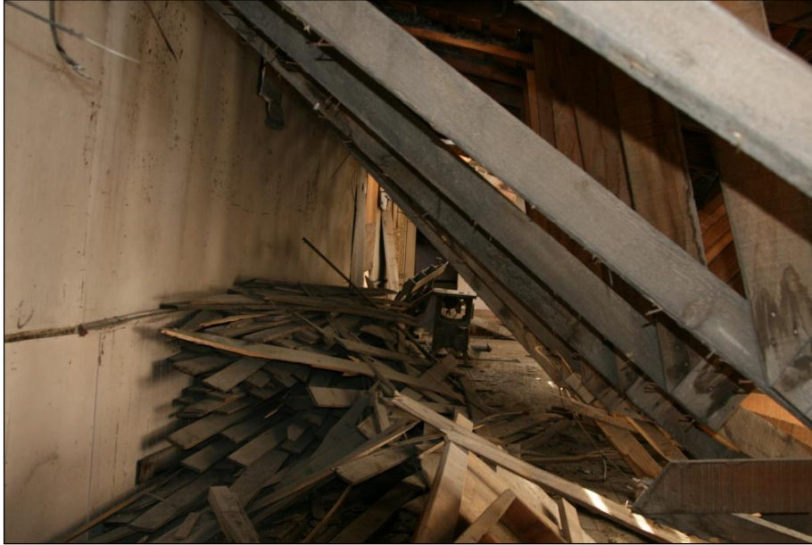
Figure 131. Eastern portion of the Mint Saloon. This area was survivable. The collapsed roof system is in the upper right.
