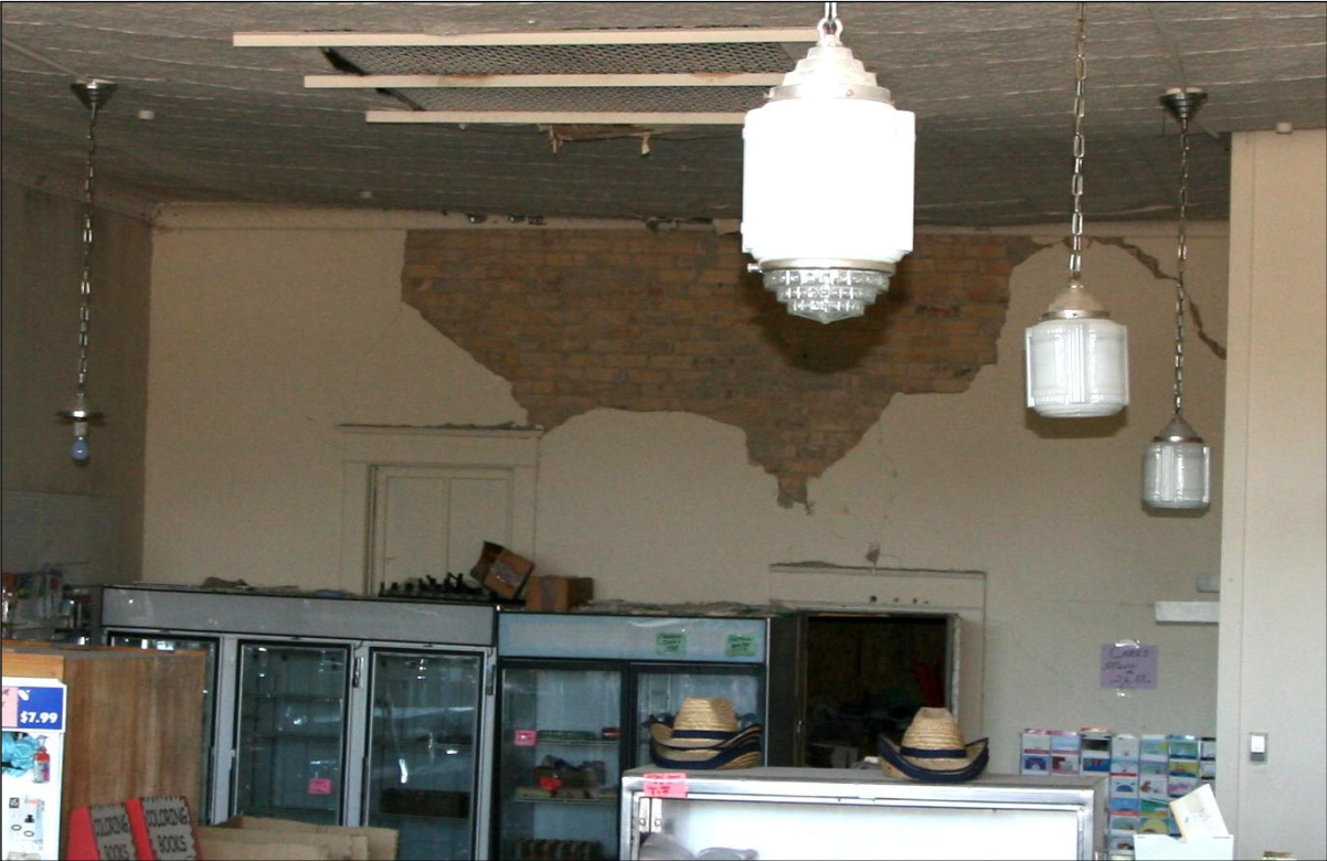
Figure 56. The back wall of the Bargain Barn shows broken Plaster, which reveals an unreinforced brick wall, probably an old back wall.
