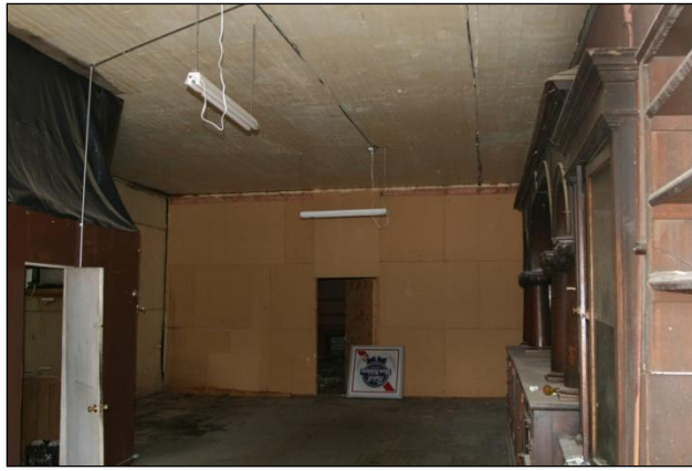
Figure 78. Interior of the Capitol Club showing few effects of the earthquake. The large bar back on the right is assumed to be unanchored to the wall. Note the fluorescent lights still hanging from the ceiling on relatively light-gauge chains.
