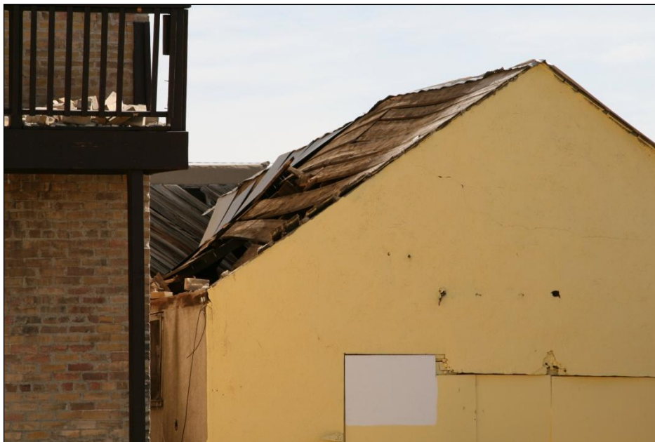
Figure 127. Back of the Mint Saloon. Holes can be seen in the roof where bricks have fallen through. The adjacent balcony that can be seen of the Nevada Hotel caught all the bricks that fell on that side.
