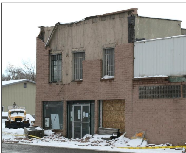
Figure 30. Failure of an unreinforced brick veneer on the Overland Hotel.
