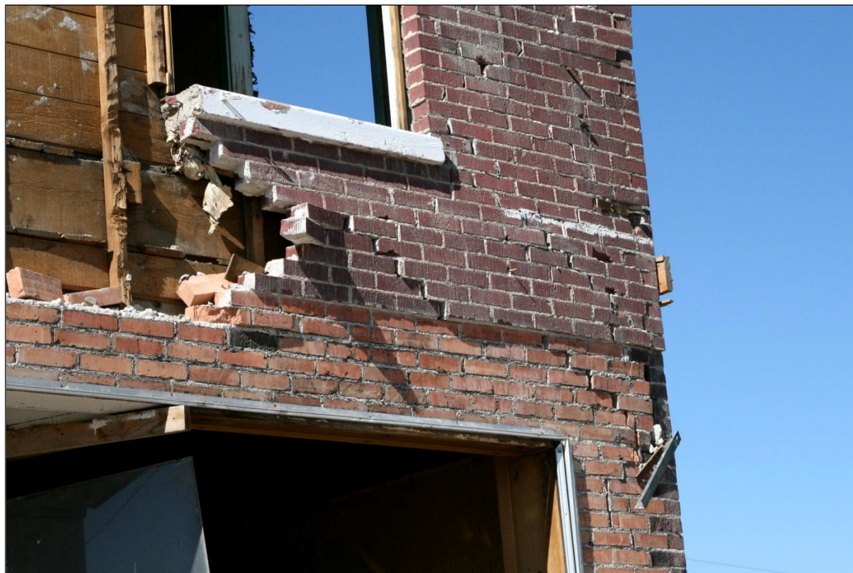
Figure 27. Large "X-fractures" in the remaining brick façade on the front of the Bullshead Bar show the break-up of the façade due to the rocking back-and-forth of the building. The lower, redder bricks are solid, older bricks. The darker bricks above have small holes in them (figure 28). The ledger for the balcony can be seen poking out on the right side of the building, just above the color change in the bricks.
