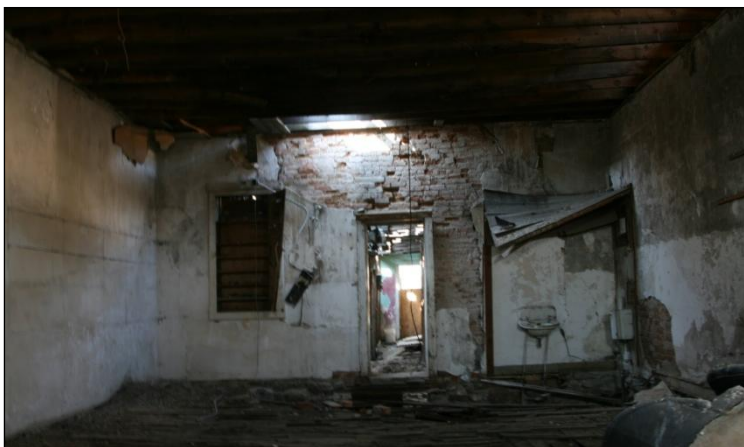
Figure 125. Inside of the Meat Market (an unused building) shows little damage, including ceiling to roof connections.
