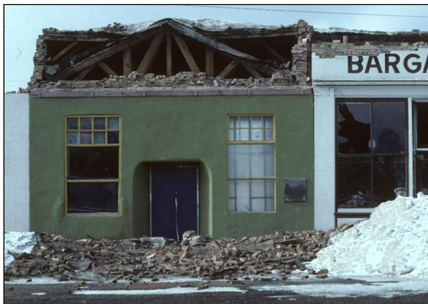
Figure 13. The gable ends of the Goble Market failed. The hole reveals two roofs on the Goble Market, with an earlier pitched roof on a truss system. Damage stopped near a horizontal wood board attached to the building (this supported a wood-covered sidewalk the past).
