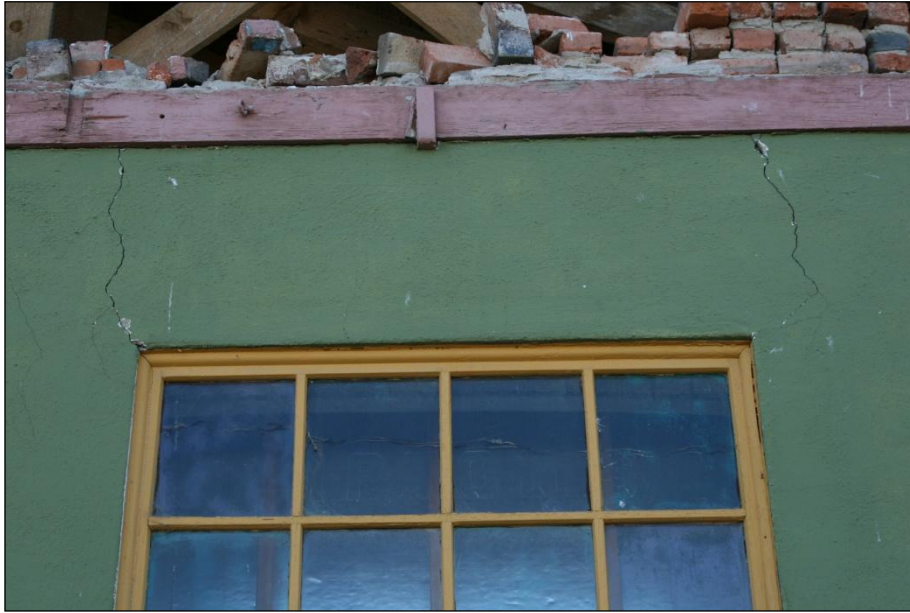
Figure 117. Cracks in the front of the Goble Market.
