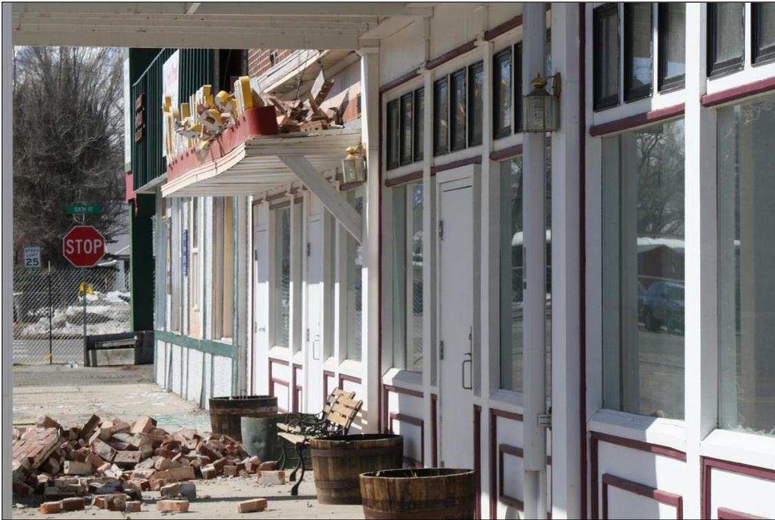
Figure 47. An El Rancho Hotel awning protected two benches from falling bricks, despite its rather meager support.
