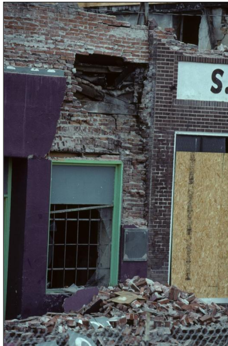
Figure 12. Failure of part of the front wall of the Capitol Club. The hole is in a wall that has three wythes of bricks. Above the hole the two outer wythes of bricks delaminated from the inner wythe, revealing a lack of cross-course bricks tying the upper wall together.
