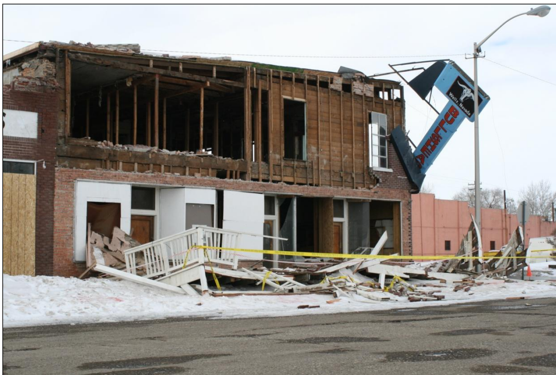
Figure 59. The northeast corner of the earthquake-damaged Bullshead Saloon with its dislodged sign.
