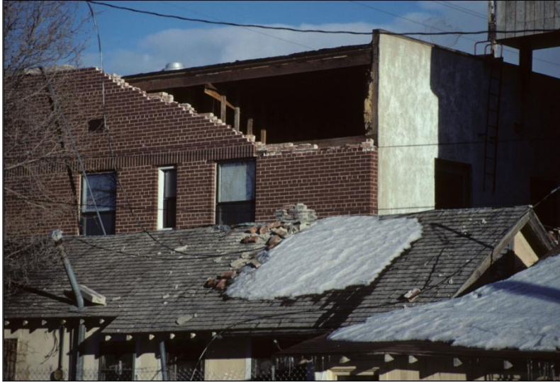
Figure 11. Parapet and wall failure of an unreinforced wall at the back of the El Rancho Hotel. Most of the bricks fell next to the building, but note the one piece of bond beam that fell far enough to clear the crest of the adjacent house; scrapes on the house roof indicate other pieces of brick cleared this crest as well and slid to the ground in front of the house.
