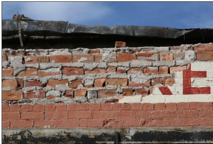
Figure 124. Detail of brickwork from the failed part of the wall. Note mortar is used on the horizontal contacts between bricks, but is missing from most of the vertical contacts between bricks.
