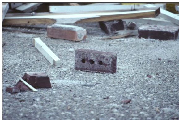
Figure 28. Brick from the upper part of the veneer of the Bullshead Bar showing small holes for the mortar to go into. Cracks seen in figure 25 that cross both types of bricks do not show distinct differences in character when they do so.
