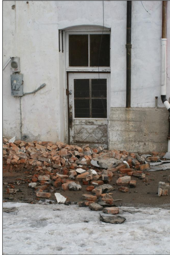
Figure 49. Bricks that fell across the back entrance of Quilici and Sons Market.
