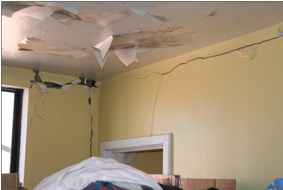
Figure 109. Severe cracking of sheetrock in the upper part of the second story of the El Rancho Hotel.
