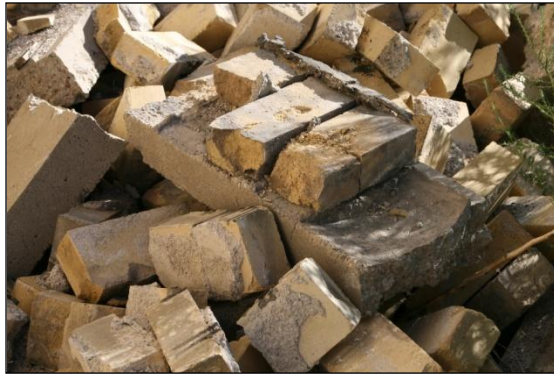
Figure 98. Bricks and a part of the concrete crowning bond beam that fell from the Eagle Club.
