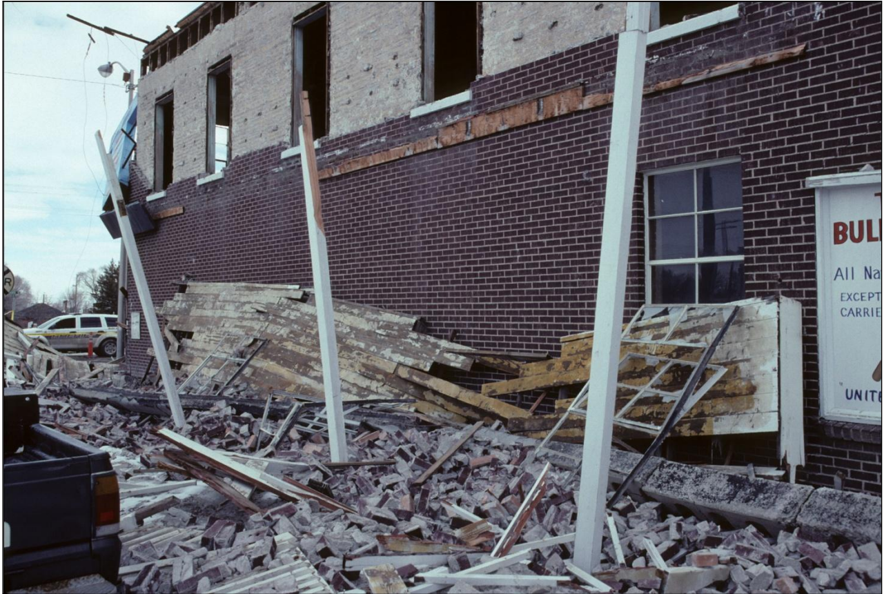
Figure 67. Western side of the Bullshead Saloon. The balcony was smashed to the ground abruptly by the crowning bond beam, breaking the column connections and leaving the columns standing. The large, nearly intact, bond beam can be seen in the central part of the photo and the lower right. This is the same beam that crushed a car to the right of the area shown in this photo.
