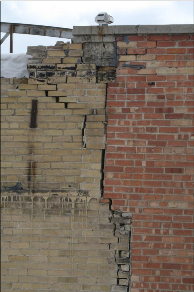
Figure 96. Damaged cold joint between two different added-on rear parts of the Eagle Club.
