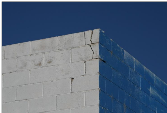
Figure 36. Damaged corner of the concrete block Supp Garage.
