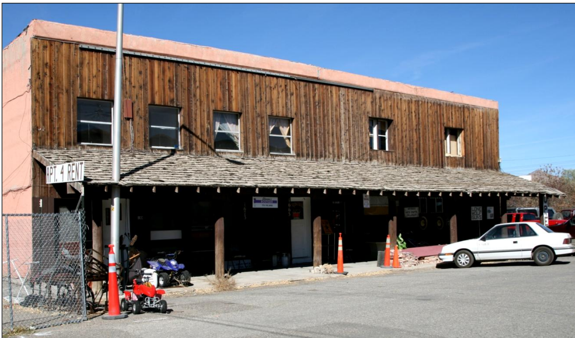
Figure 34. The Frontier Apartments are in a composite wood/railroad tie/concrete building in old town that survived the earthquake fairly well, although it had some nonstructural damage.
