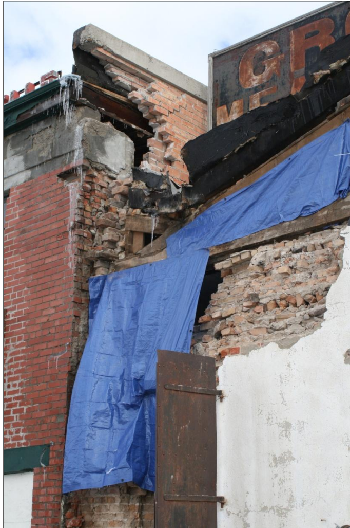
Figure 25. A hole has been pounded out of the eastern wall of the Wells Chalet. The upper part of this wall is two wythes wide. Note how the crowning concrete bond beam on top of the eastern wall and some bricks overhang the concrete beam on the southern wall, giving a hole-like appearance to the damage; this failure does not appear to have peeled down from the top as many of the other wall failures did. The concrete beam appears to have pounded this hole into the wall. This pounding and the resulting falling bricks may have contributed to damage in the upper corner of the back of the Quilici Market. The blue tarps were put up the day of the earthquake to cover holes to protect the interior from weather.
