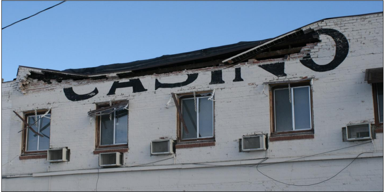
Figure 151. Failure of an upper section of the western wall of the Old West Inn. Most of the bricks fell outwards.
