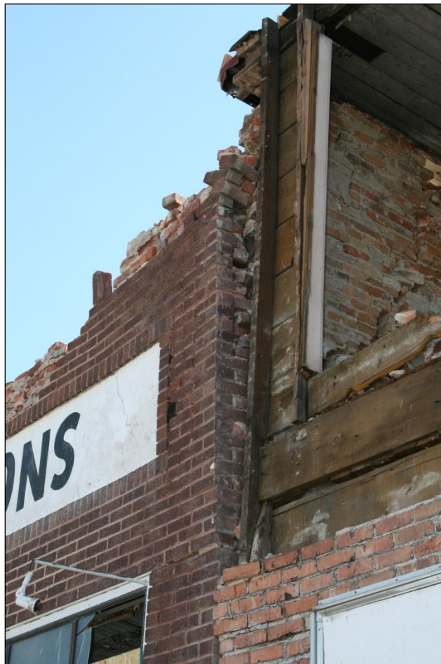
Figure 156. The front corner of the upper part of the front of the Quilici and Sons Mercantile is leaning outwards in a threatening way, despite the cross-course bricks on the end. There is a concentration of shaking damage at the corner of these two buildings.
