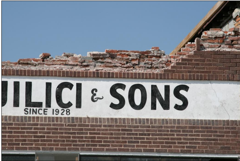
Figure 155. Fallen and delaminated bricks from the front parapet.
