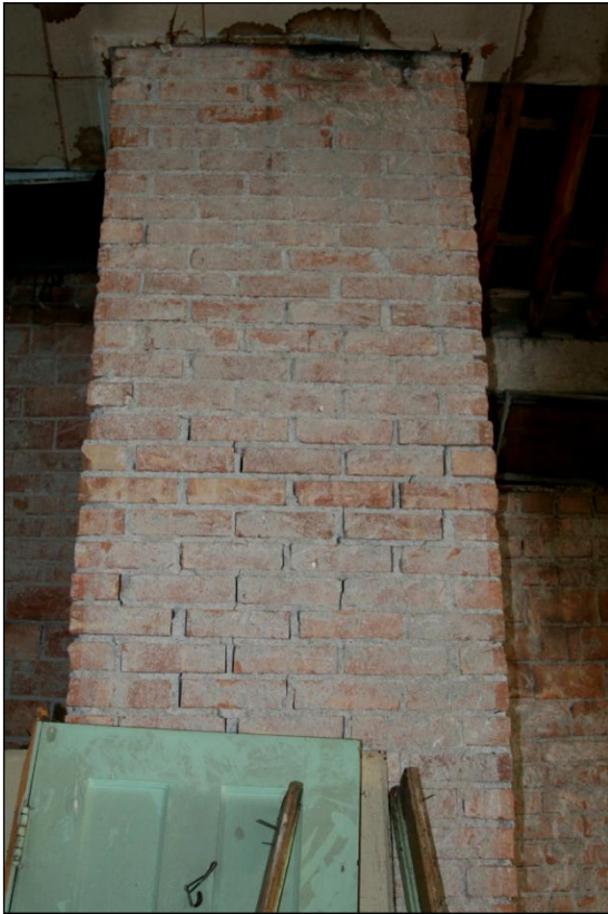
Figure 184. Chimney inside the Wells Chalet that shows cracking consistent with buckling out in the middle (see figure 185).
