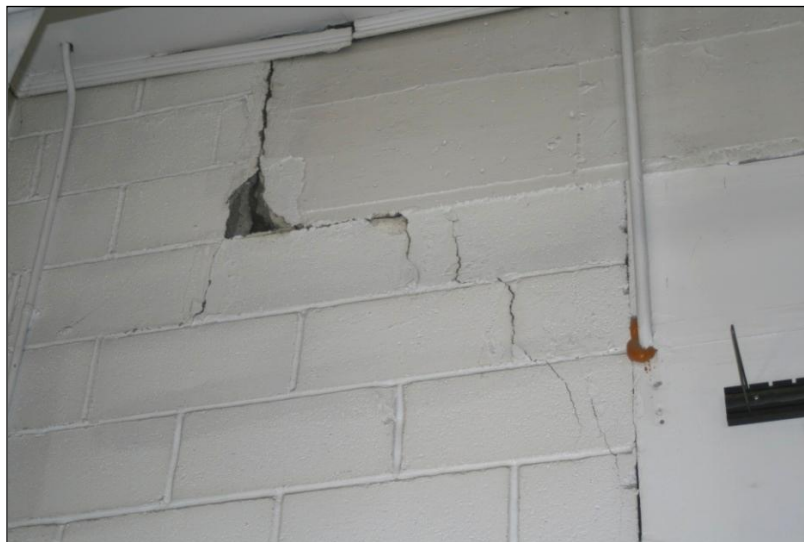
Figure 38b. Close-up view of the cracking shown in figure 38a.
