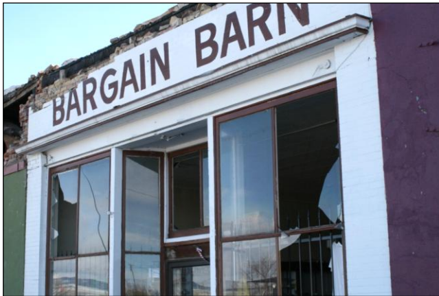
Figure 50. Front of the Bargain Barn store showing a couple of broken windows. The area above the sign is where the decorative cornice fell out. The broken windows on the left side of the store front in the picture are next to a column that was displaced at its top.
