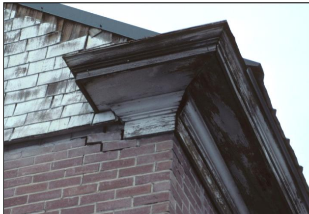
Figure 85. Cracking in the upper corner of the City Shop building, just below a wooden cornice.
