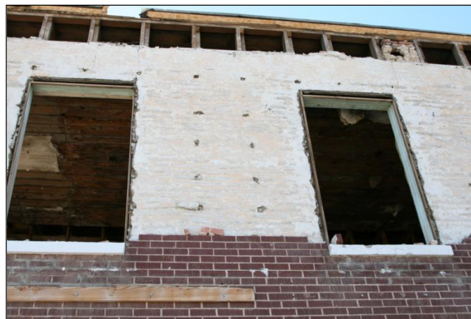
Figure 68. Part of the western wall that shows where the brick veneer has peeled away. The dark areas in the wall are where the nails tied the veneer to the building (many still have the nails in them that weren't pulled out – the veneer probably broke up around them). The window frames and glass fell out with the bricks.
