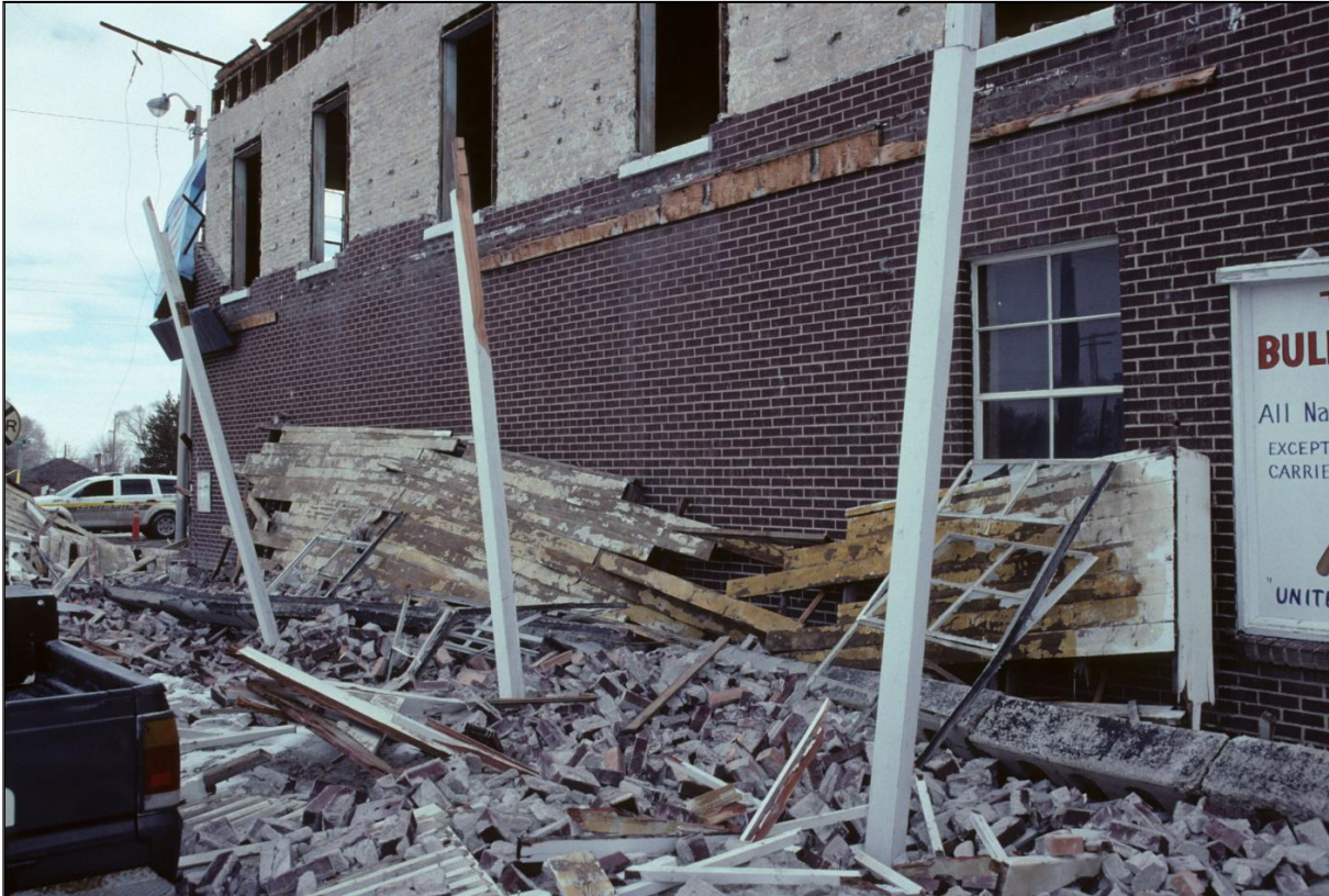
Figure 19. Western side of the Bullshead Bar. The balcony has been smashed to the ground abruptly breaking the column connections and leaving the columns still standing. This likely happened because the balcony was rapidly impacted by the large, nearly intact crowning bond beam that can be seen in the photo. This is the same beam that crushed a car to the right of the area shown here (figure 17).
