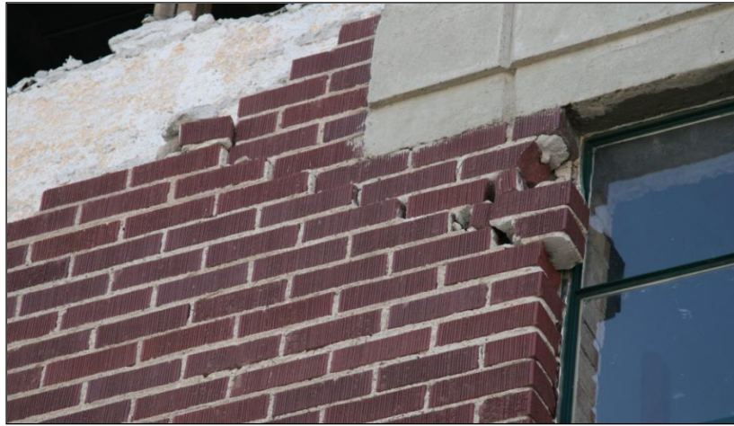
Figure 180. Broken bricks under and near the end of the concrete beam shown above.
