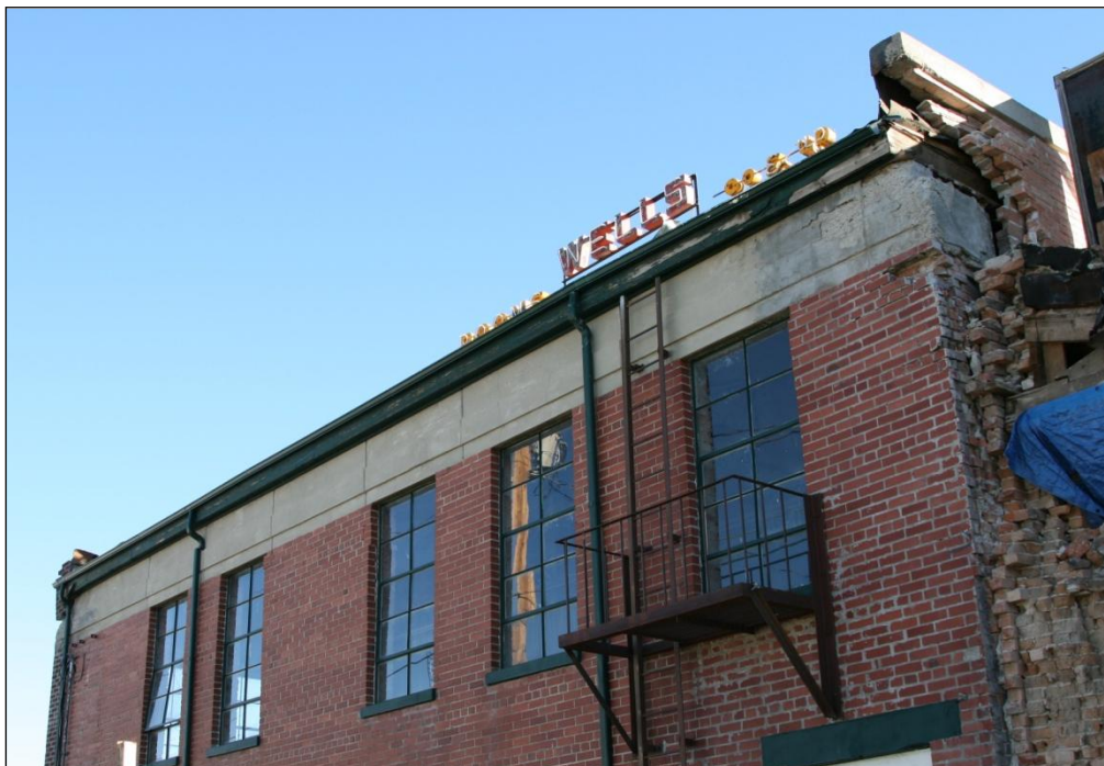
Figure 175. Close-up of the second story concrete beam that apparently moved back-and-forth in an east-west direction. In several places between the windows, the wall is delaminating.
