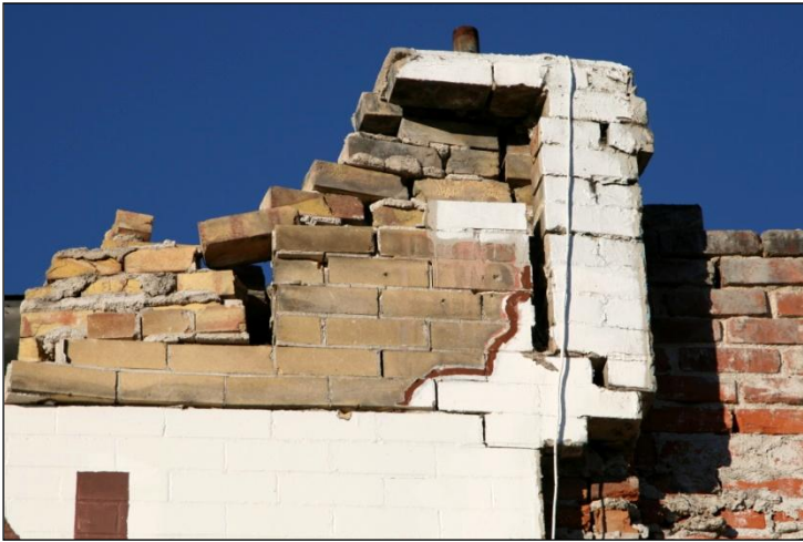
Figure 52. Top of front wall of the Bargain Barn where the cornice pulled out. Note the paint outline. This western side of the parapet didn't fail but was badly damaged.
