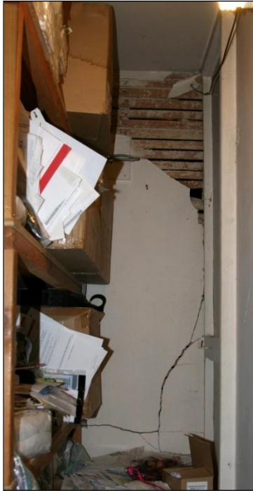
Figure 35. The eastern portion of the building had racked and fallen plaster.
