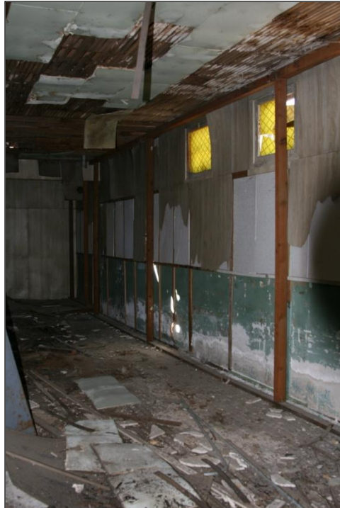
Figure 45. Bracing under the ceiling joist connections and roof. This example is from the Eagle Club.
