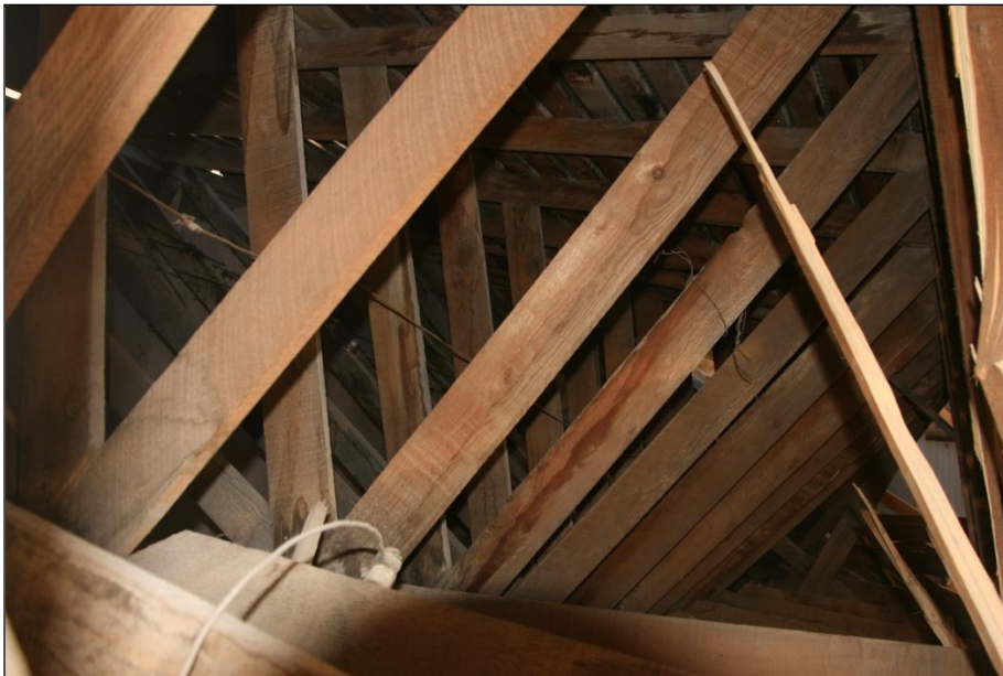
Figure 132. Tilted truss roof system showing it mostly collapsed as a unit.
