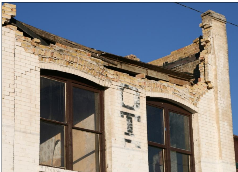
Figure 141. Upper part of the Nevada Hotel. The roof collapsed down to the second-story ceiling level. The upper part of the front parapet and wall has completely fallen out and several parts were left out-of-plane.
