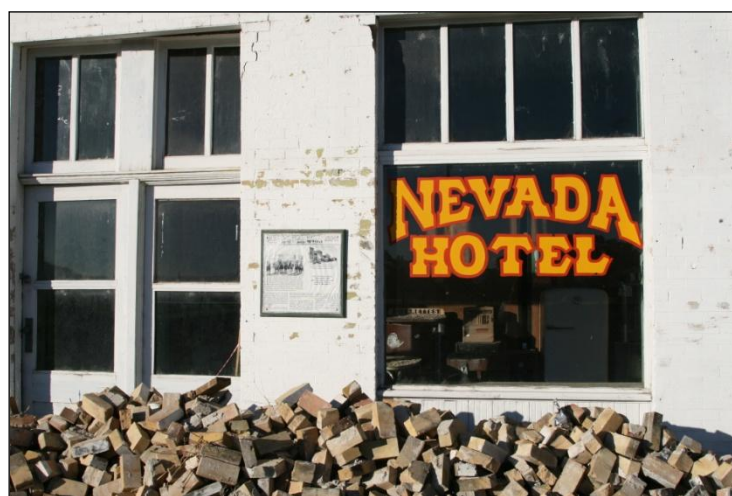
Figure 144. Bottom of the front of the Nevada Hotel showing bricks fallen from above. No windows were broken, but the frame for the windows and doors on the left is coming out of its opening.
