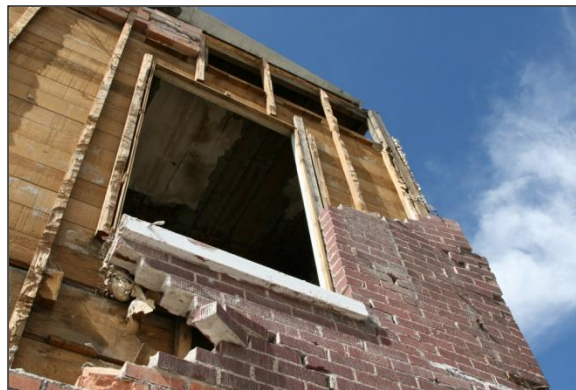
Figure 32. Wood frame of the Bullshead Bar exposed at the northwest corner of the building where the brick cladding has come off. The remaining cladding is damaged and ready to fail, which would also allow the concrete window sill to fall.
