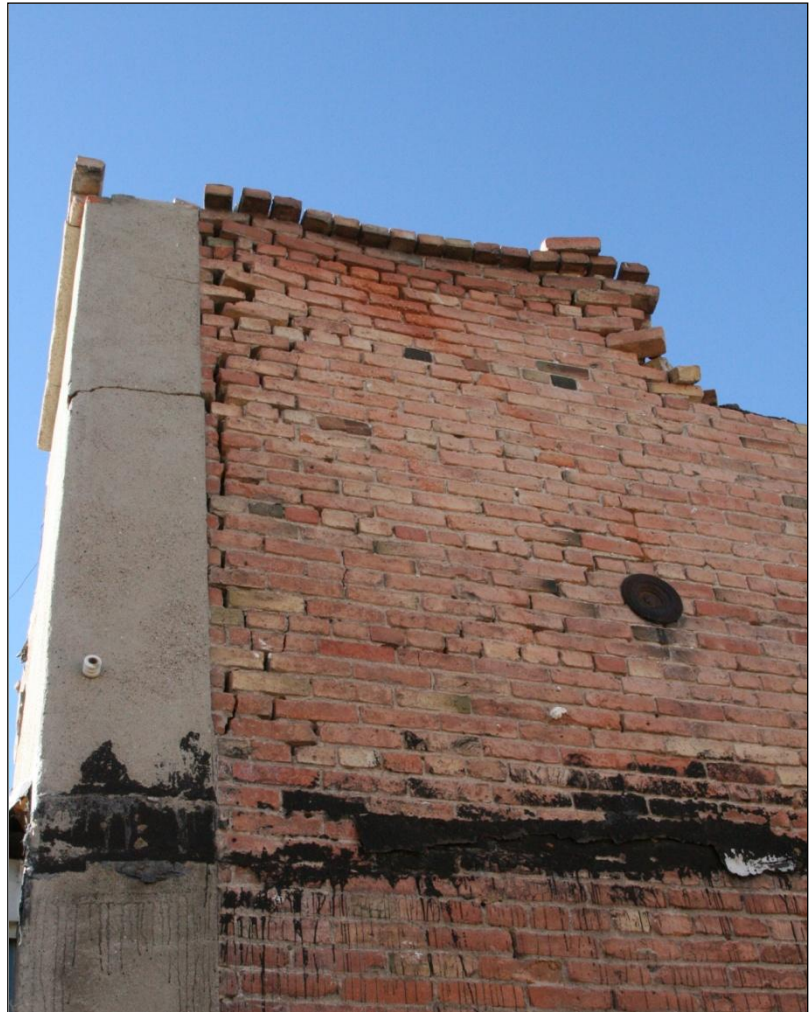
Figure 120. Damaged southeastern corner of the Goble Market.
