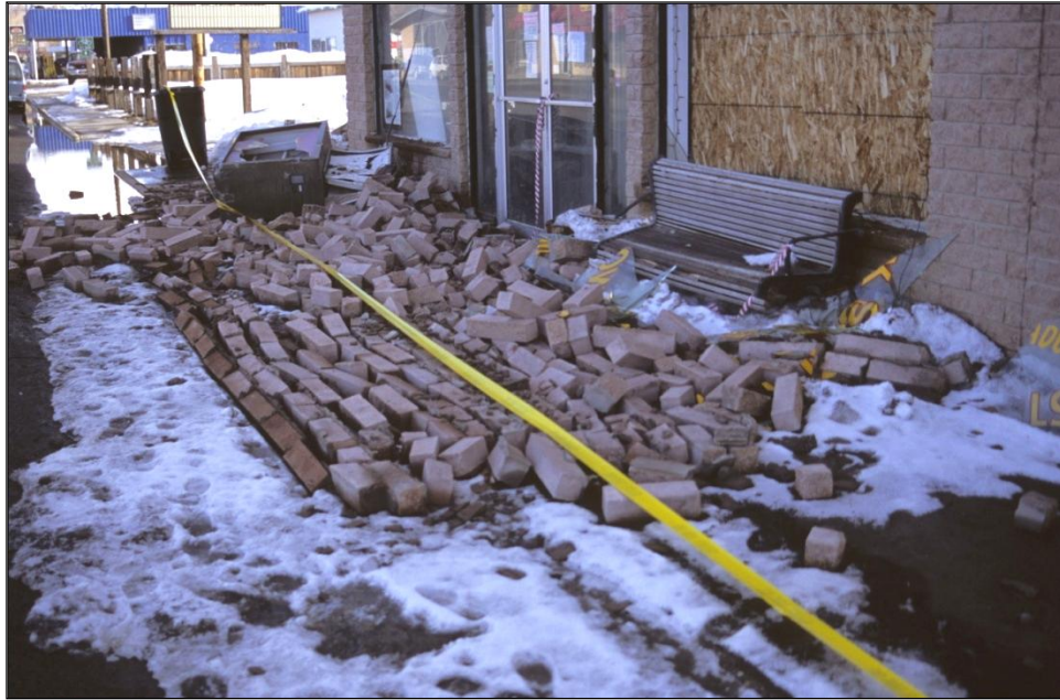
Figure 31. Failure of an unreinforced brick veneer on the Overland Hotel. The ordered nature of the bricks indicates much of the veneer fell out en masse .
