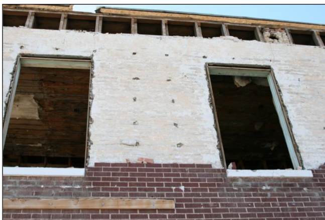
Figure 29. The second story of the western wall of the Bullshead Bar where the unreinforced brick veneer has fallen off. The darker areas on the white wall are where nails, either single or clusters of nails up to three in number, were driven into the wall studs. This was how this one-wythe-wide veneer was attached to the building.
