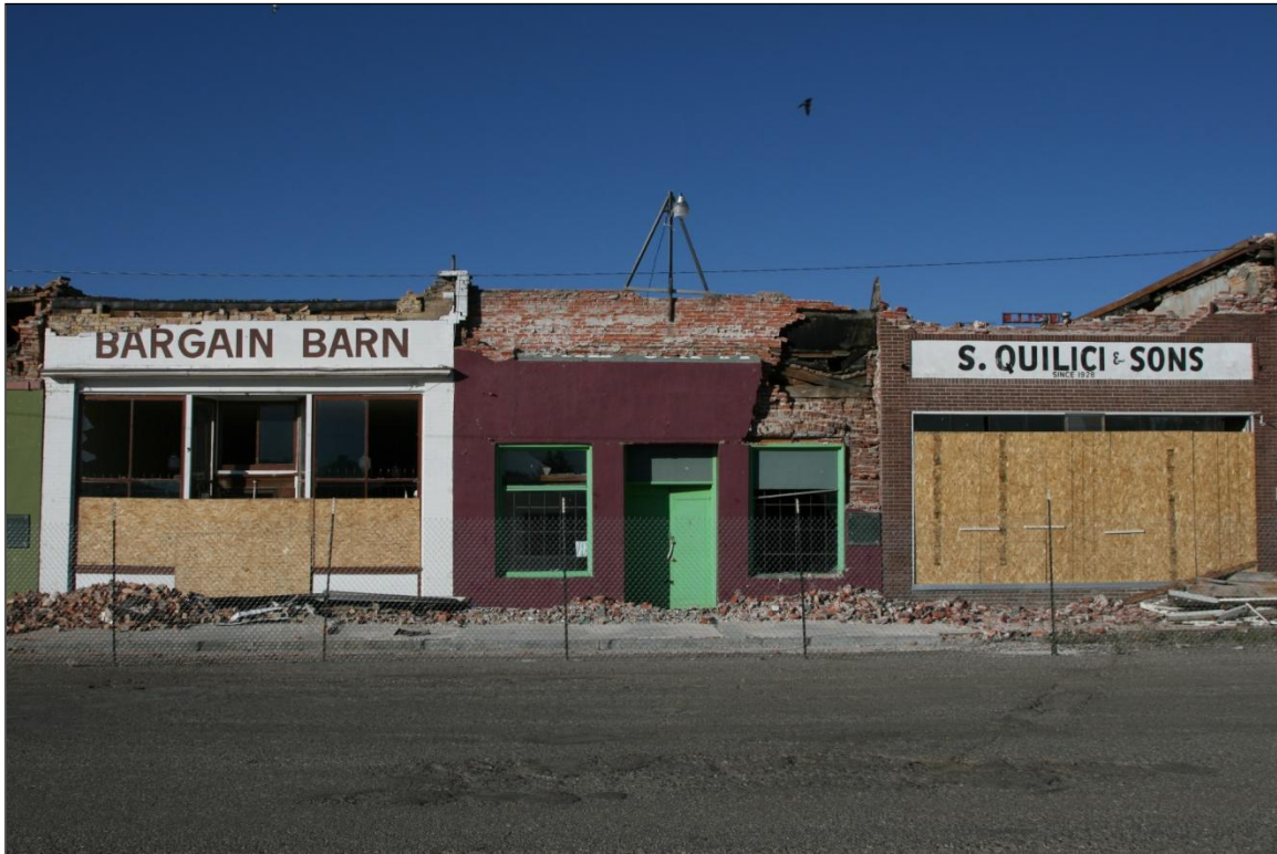
Figure 73. The front of the Capitol Club (purple building in the center with green trim and doors). The upper parts of the parapet and wall have failed and thrown bricks onto the front sidewalk, across the entrance.
