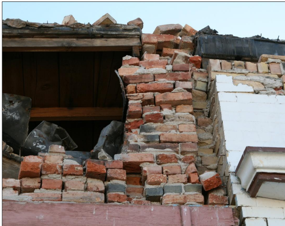
Figure 116. Detail of the bricks of the front of the western wall of the Goble Market. Several vertical contacts between bricks are missing mortar.
