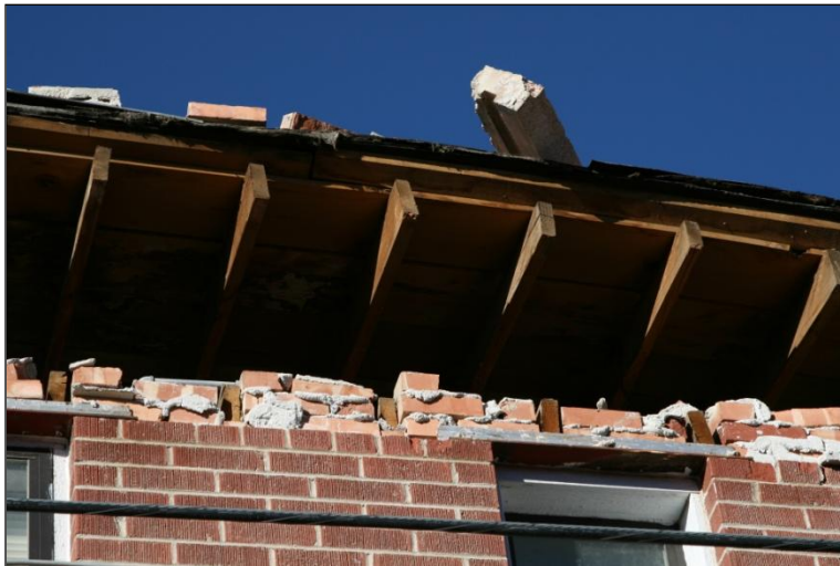
Figure 104. Close-up of the wall failure showing hanging roof joists, a section of bond beam on the roof, and the exposed ceiling joist connections.
