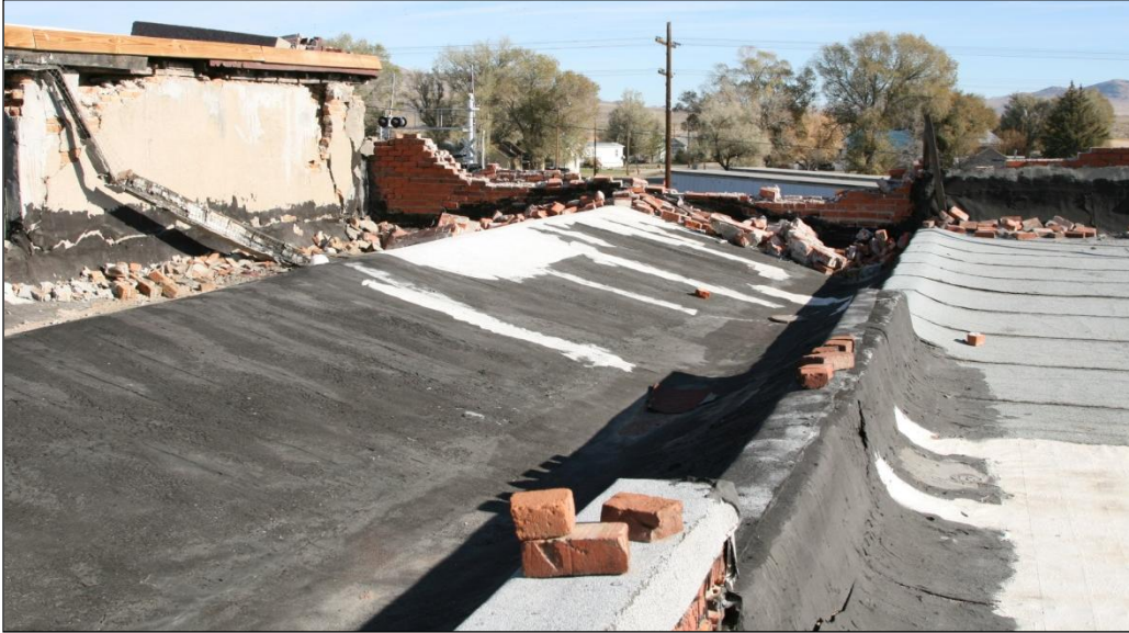
Figure 158. View to the north (front) of the Quilici and Sons Mercantile showing failed parapet from the back.
