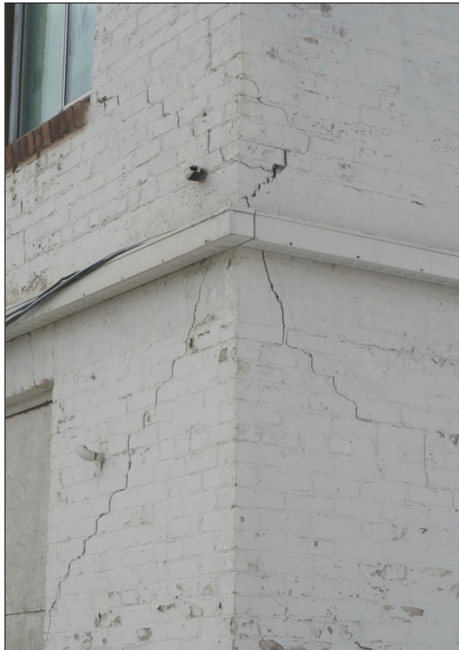
Figure 152. Cracked northwest corner of the Old West Inn.
