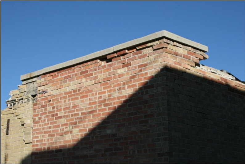
Figure 97. Remaining part of the crowning bond beam and upper wall near the back southwest corner of the Eagle Club.
