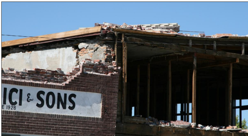
Figure 62. Upper eastern corner area of the front of the Bullshead Saloon. The open area of the second story can be seen, along with part of the eastern unreinforced brick wall, badly cracked near the corner. A section of the bond beam can be seen on the roof.
