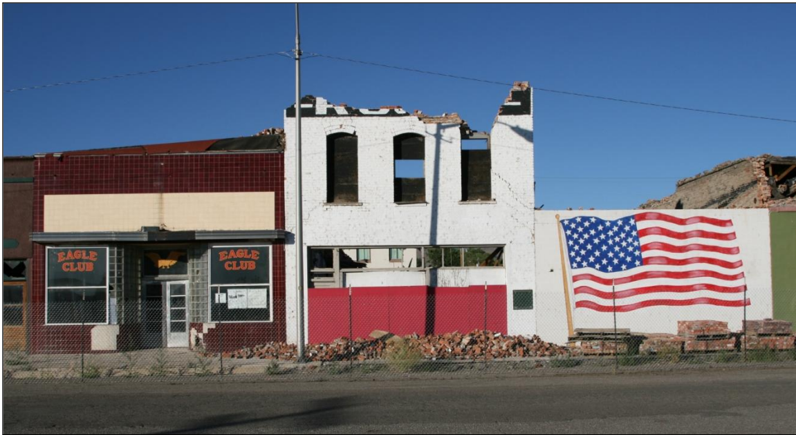
Figure 166. Remaining front of the San Marin Hotel after the earthquake.
