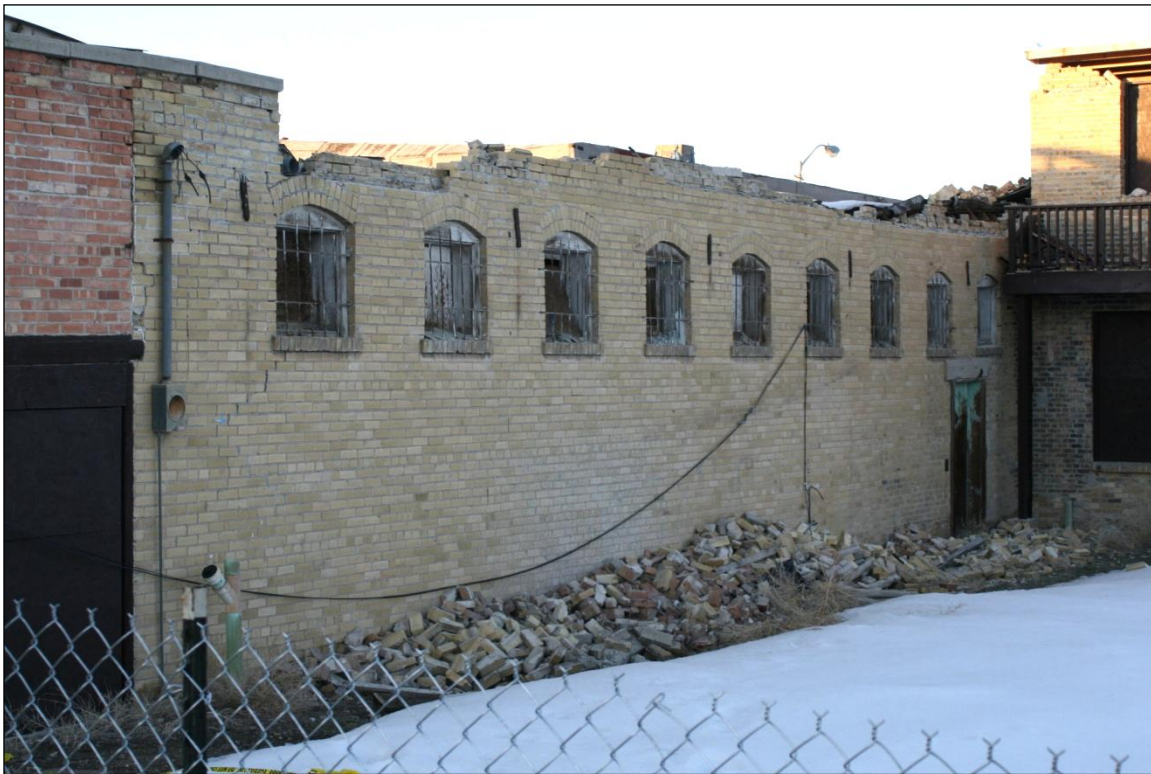
Figure 138. Fallen parapet at the back of the Murphy's Bar.
