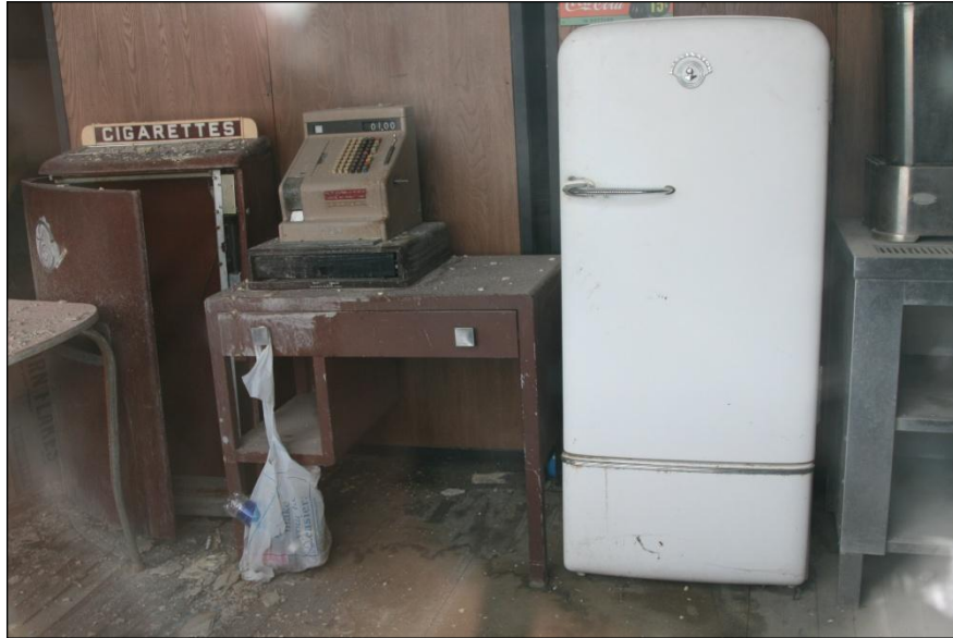
Figure 145. First floor interior of the Nevada Hotel. The refrigerator and cash register did not fall. Most of the interior of the Nevada Hotel was not damaged although the second story could not be inspected.
