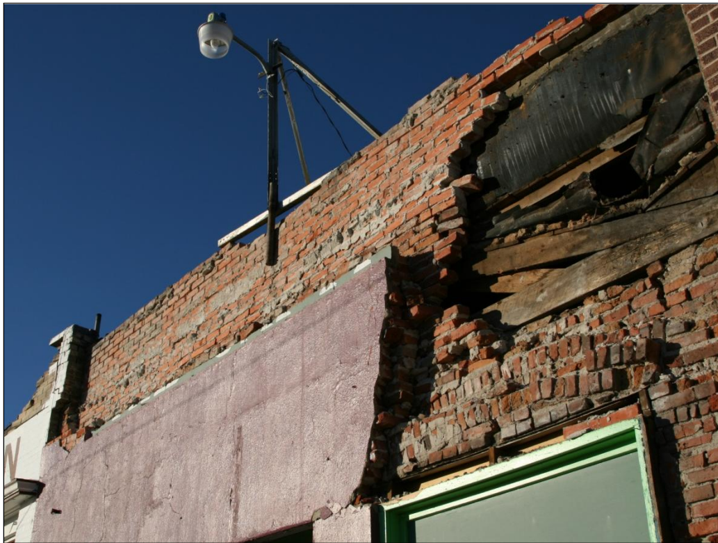
Figure 74. The front of Capitol Club where bricks fell out. Note the even face of the upper part of the remaining wythe of bricks indicating a lack of cross-course bricks to tie the wall together.
