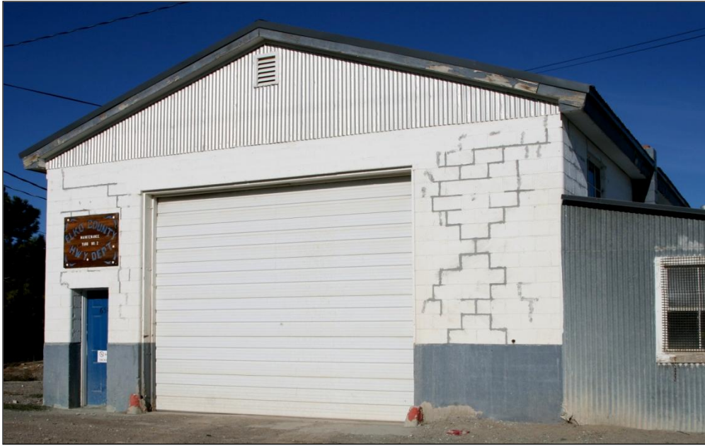
Figure 39. Patched cracks in the eastern wall of the Elko County Highway Department building. Cracks are between the blocks and show some crude "X" patterns.
