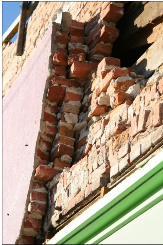
Figure 76. Detail of bricks in the front wall of the Capitol Club. Some widely spaced cross-course bricks can be seen.
