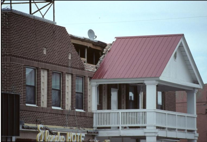
Figure 101. Upper part of the front unreinforced failure brick wall that fell out.
