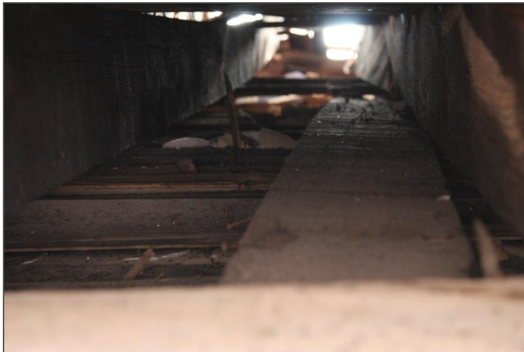
Figure 6. Roof rafters from the San Marin Hotel lying directly on the second story floor. There was very little survival space in this collapse.
