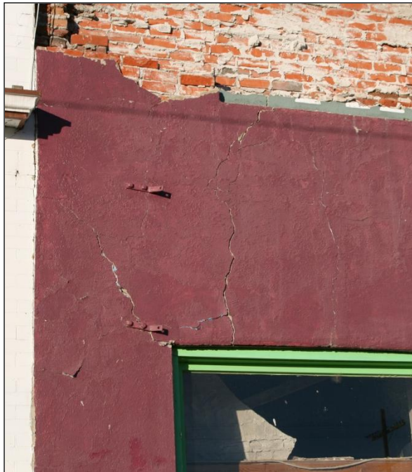
Figure 77. Part of the front wall of the Capitol Club that has not failed but is badly cracked. Note in the window that a part of an interior plaster ceiling has failed.
