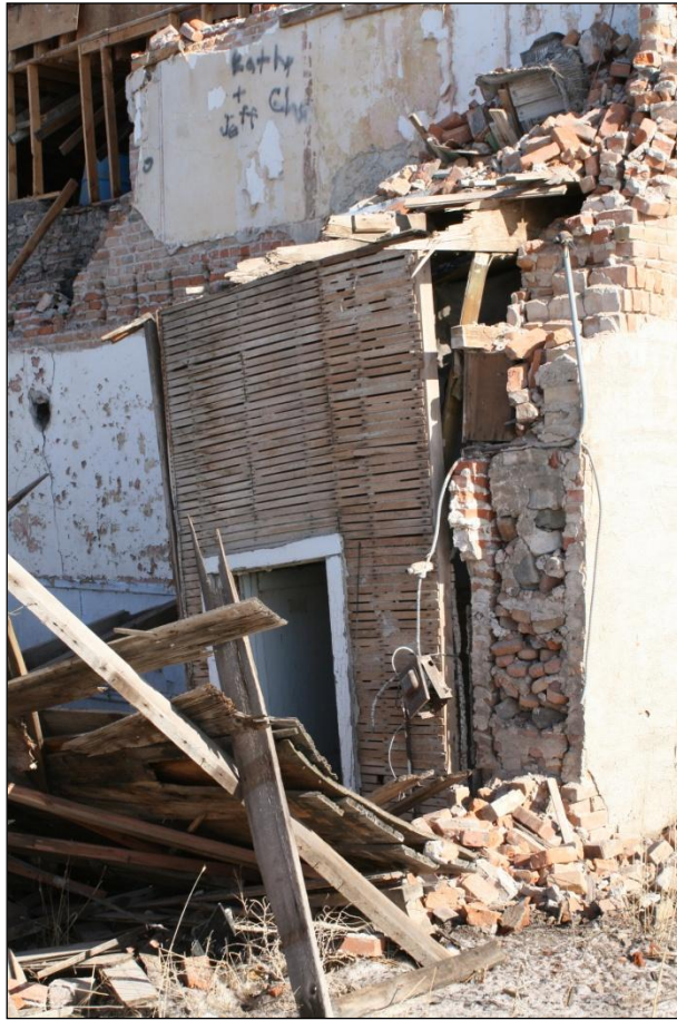
Figure 171. The small room in the back of the San Marin Hotel appears to have been one of the few interior rooms in the hotel. This one of the few potentially survivable spaces in the collapsed building.
