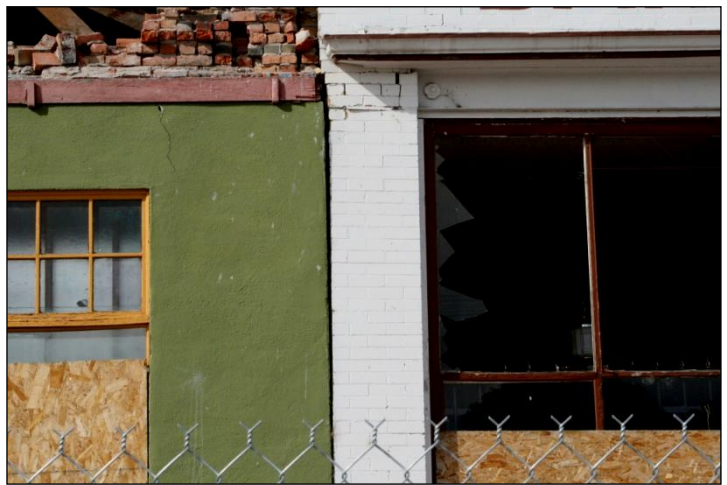
Figures 53. Pounding damage to the eastern wall of the Bargain Barn.
