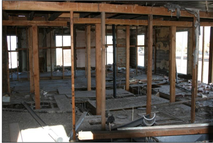
Figure 46. Interior wood bracing in the second story of the Bullshead Bar; the first story had bracing as well (figure 33).
