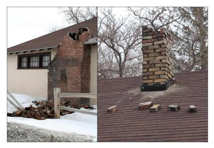
Figures 9 and 10. Two damaged chimneys at the same house from the earthquake. This is evidence of intensity MMI VII.
