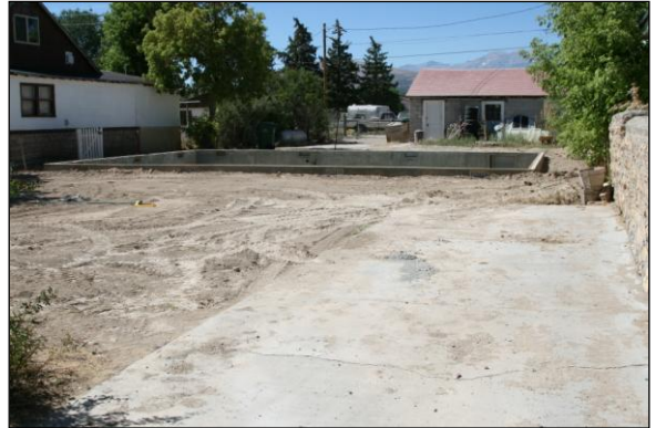
Figure 27. The removal of the badly damaged rock house and the new foundation were funded by the relief fund from donations and recovery rally.
