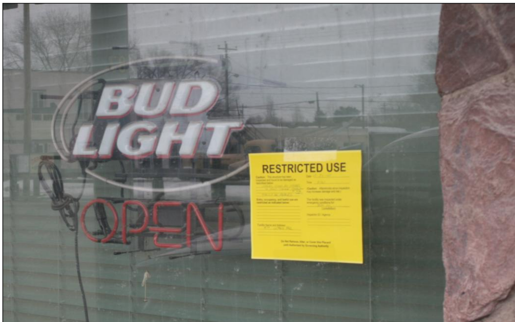
Figure 3. The local bar was in use by day three, but the open sign was not lit because of the yellow tag (cracking in side parapets and walls). This was an important social place for many people to gather and talk about the earthquake. Several people who hadn't been downtown in years dropped by, partly to have some company.
