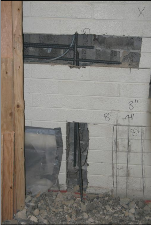
Figure 17. The above photograph shows a detail of the rebar in the slots prior to being tied together.
