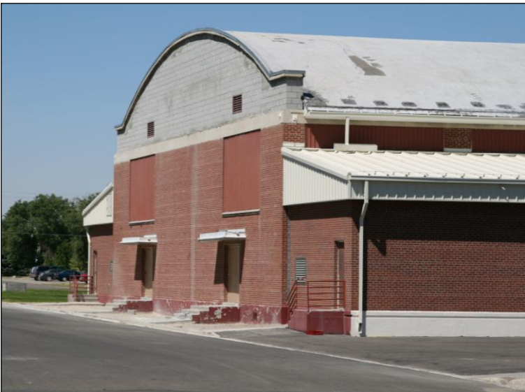
Figure 15. Completed reconstruction of the rear wall of the Wells High School gymnasium.
