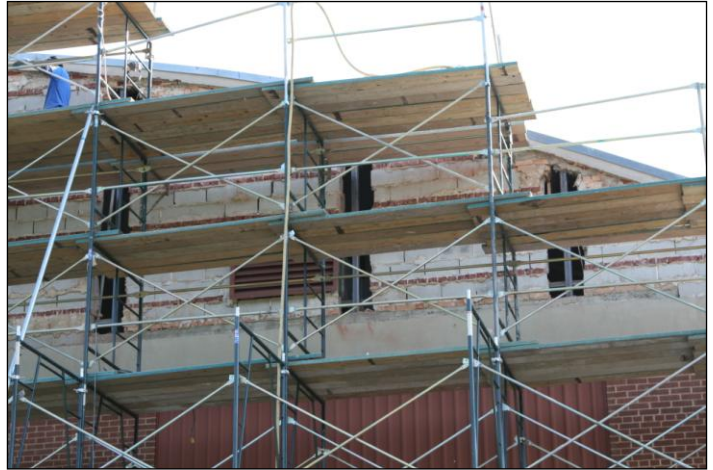
Figure 14. Close-up of the reconstruction of the rear wall of the high school gymnasium.
