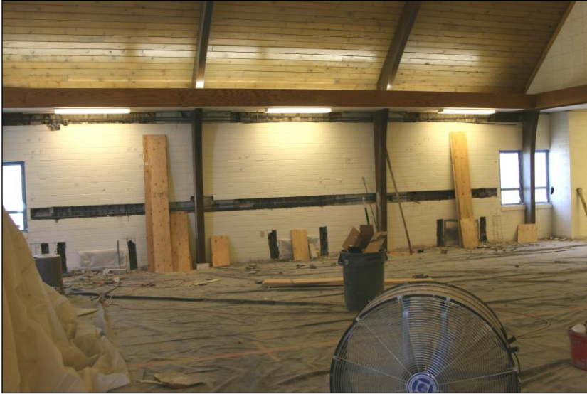
Figure 16. Reconstruction of the LDS Church which had severe cracking and some column damage. The building was only partially reinforced, so during reconstruction the building was rehabilitated to be seismically resistant. This photograph shows the removal of sections of the front of hollow concrete blocks to place rebar and concrete in these and create reinforced columns and reinforced beams in the LDS Church reconstruction.
