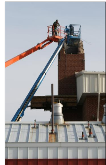
Figure 11. More of the careful demolition work on the chimney the day after the earthquake).
