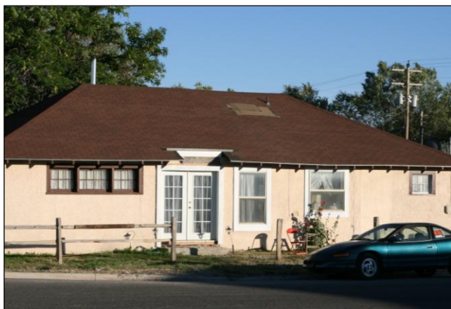
Figure 25. This part of the house was later remodeled to have a new set of French doors.
