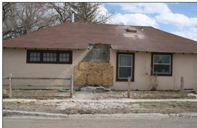
Figure 24. Volunteers tore the rest of the chimney down, stacked the bricks (since removed in photo), and boarded up the hole left by the fireplace.
