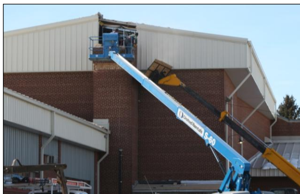
Figure 12. The chimney nearly entirely taken down to its damaged level.
