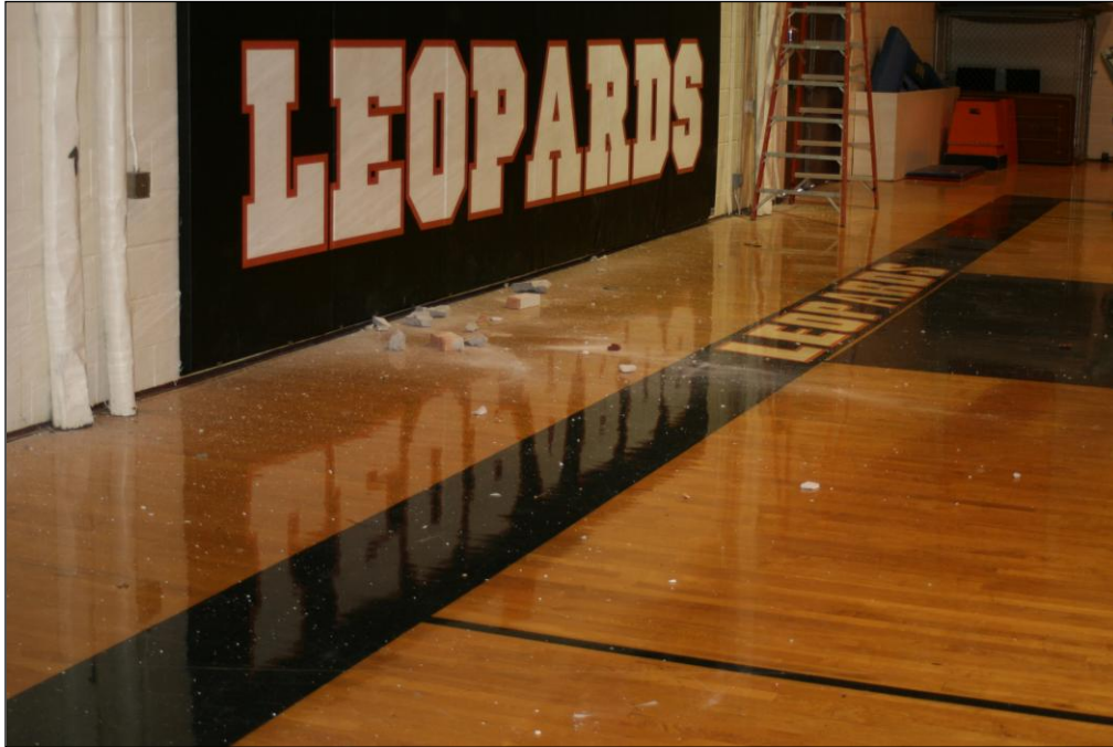
Figure 1. Bricks thrown down inside the high school gymnasium from an upper, unreinforced masonry wall that was starting to breaking up during the 2008 Wells earthquake. The high school buildings sustained $2.48 million in damage. These buildings were restored and back in use within six months.
