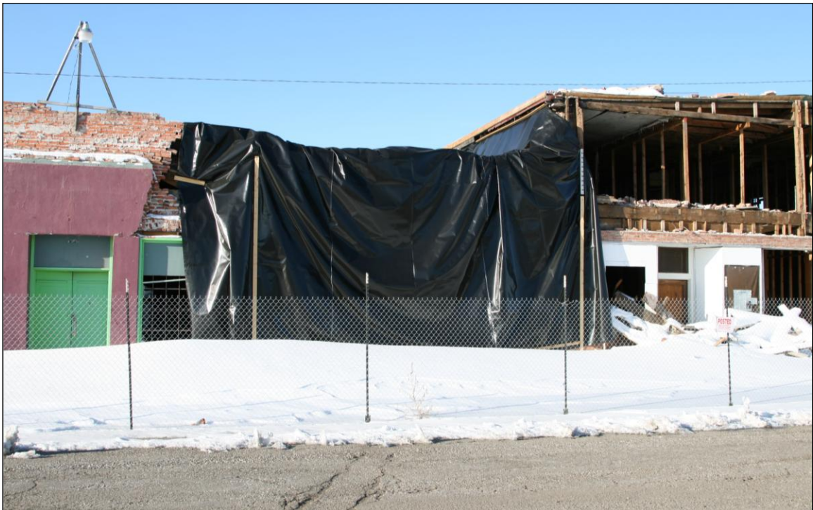
Figure 30. Quilici Market was also covered with black plastic used as weather-proofing until it could be reconstructed.
