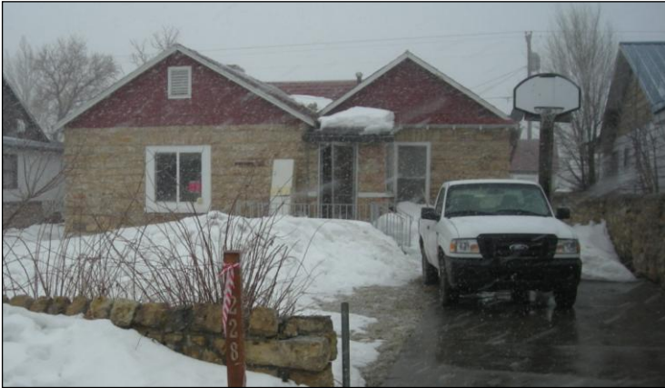
Figure 26. Rock house that was damaged beyond repair from the earthquake with a failed rubble-wall foundation, failed lower part of a wall, and failed wall-roof connection. Photo by Wells resident.
