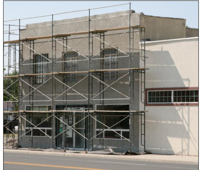
Figure 20. The Overland Hotel after the bricks were peeled off the front and sides of the building and it received a stucco treatment.
