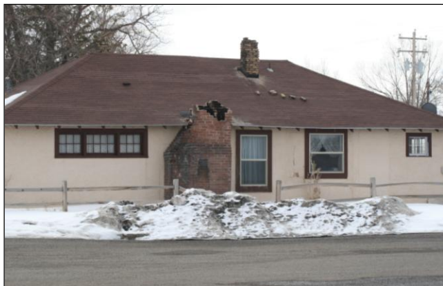
Figure 23. Earthquake-damaged chimneys.
