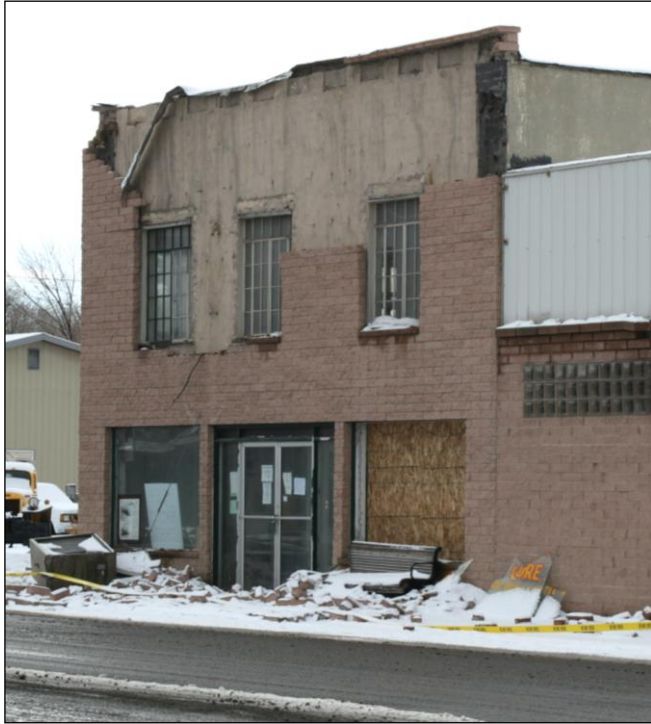
Figure 19. The earthquake-damaged Overland Hotel where bricks and window glass rained down over the entrance and bench in a potentially deadly fashion.
