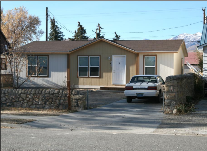
Figure 28. The new home that replaced the badly damaged one was partly funded by the Nevada Homeowners Disaster Assistance Fund.
