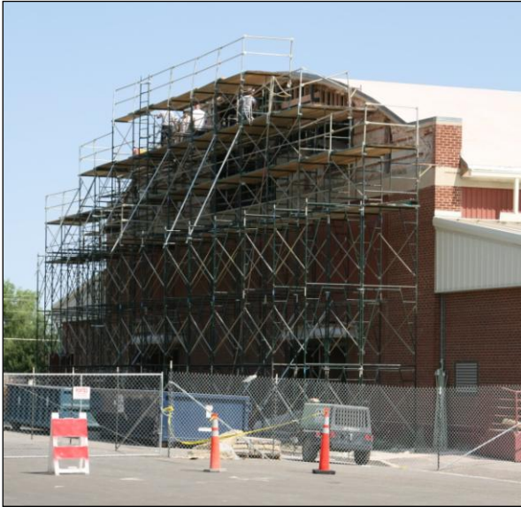
Figure 13. Reconstruction of the rear wall of the high school gymnasium.
