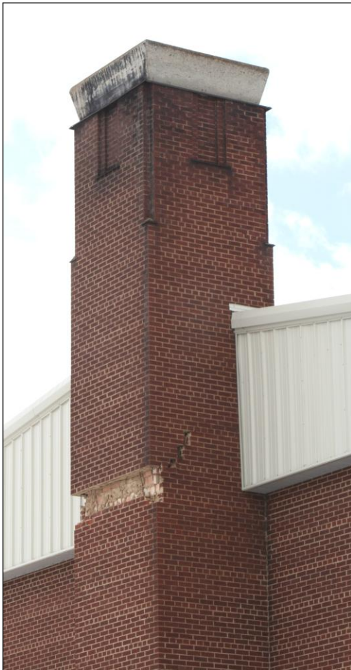
Figure 9. The earthquake-damaged chimney of the Wells High School auditorium.
