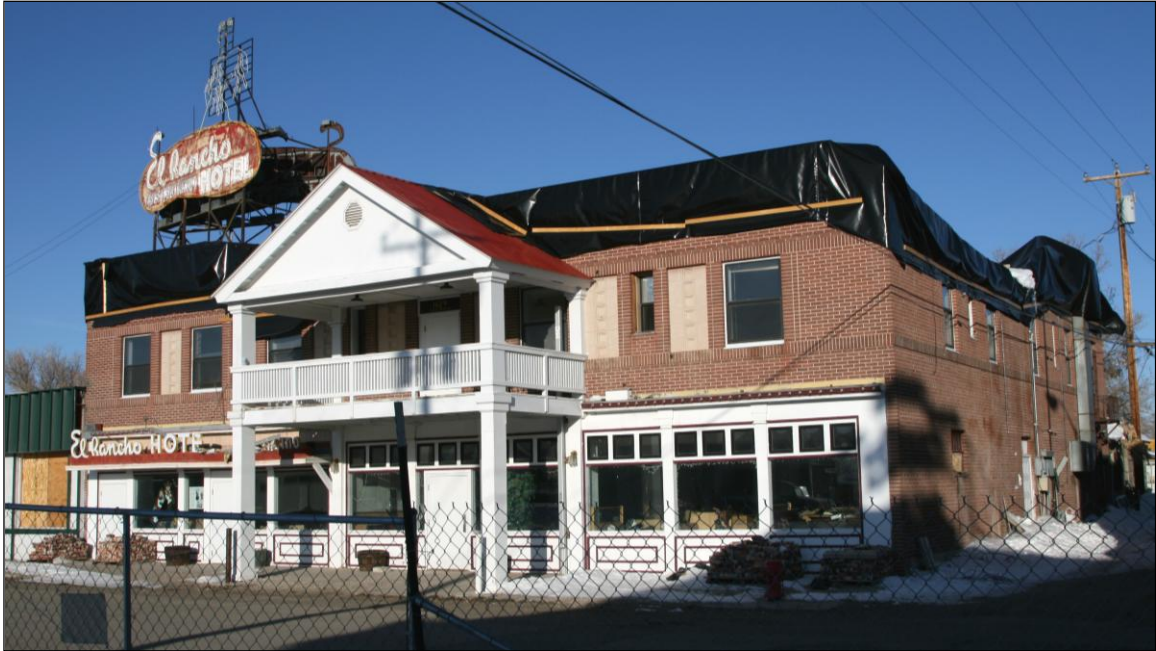
Figure 29. Temporary protection of buildings from weather; a large plastic tarp covers the top of the El Rancho Hotel where collapsed walls allowed the rain and snow into the building.
