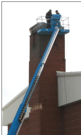
Figure 10. Careful demolition of the chimney that began the day after the earthquake.
