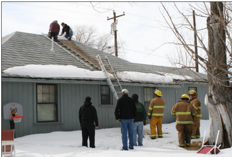
Figure 22. Recovery began immediately following the emergency response. Here some available response personnel are helping take down a damaged chimney and cover the hole for a single mother. Caution was used because large aftershocks were still occurring.
