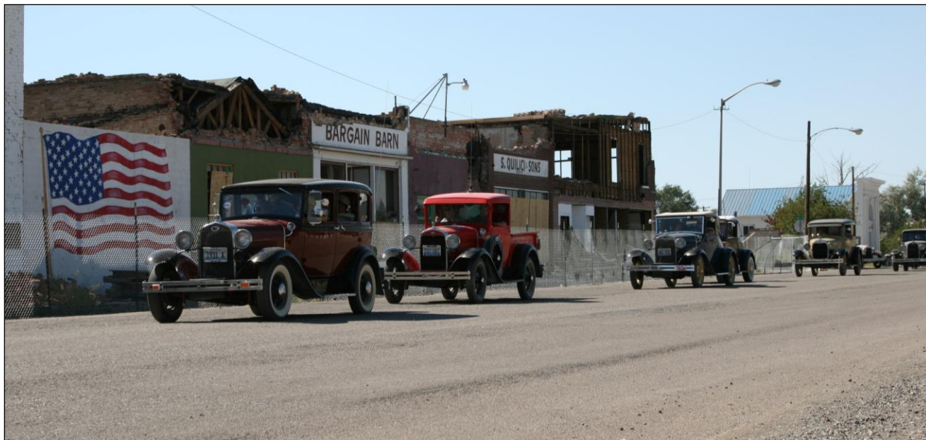
Figure 4. A chain-link fence surrounds the damaged historical district. A caravan of old cars was passing this day as if to pay homage to old friends.
