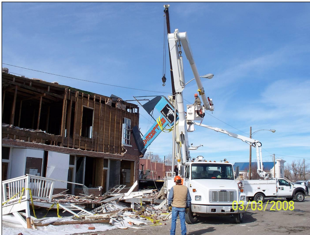
Figure 32. Removing the unstable Bullshead Bar sign that was leaning against a lamppost, in danger of falling from aftershocks. Photograph by Wells resident.
