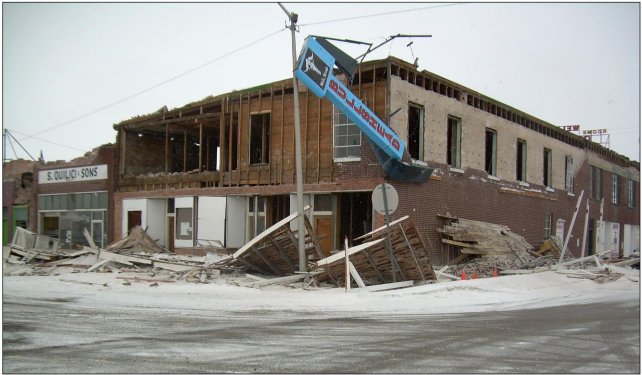
Figure 7. Damage to the Bullshead Bar from the 2008 Wells earthquake. Brick veneer fell from the second story along with a crowning concrete bond beam, which both smashed the balcony to the ground. Photograph by Nick Stake.
