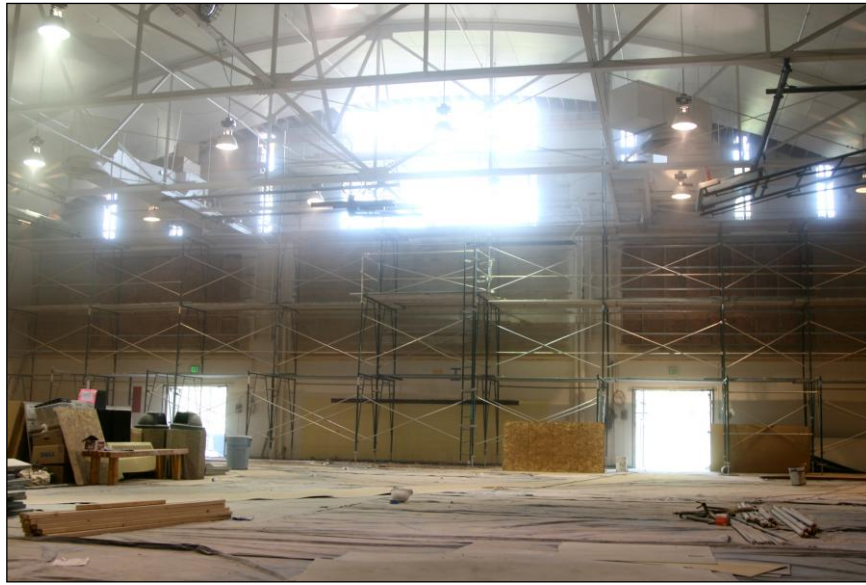
Figure 21. Reconstruction of the Wells High School gymnasium. This will be a safer building for the high occupancy the gym occasionally has during any future earthquakes.
