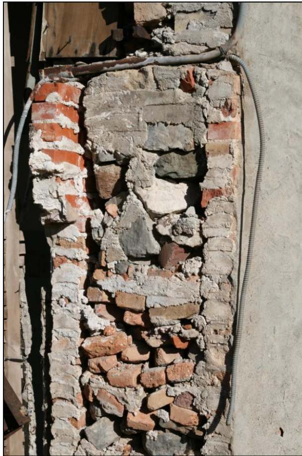
Figure 26. A damaged wall exposed a rubble infill of broken bricks and rocks with intermittent mortar dumped in, all hidden behind a single thickness of laid brick wall. This kind of construction offers an uncertain performance during an earthquake.
