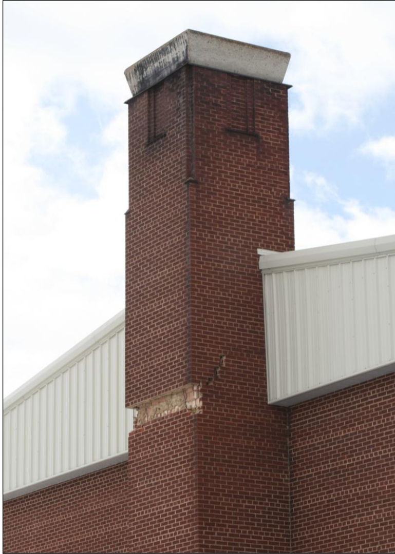
Figure 11. Large chimney on side of the Wells High School auditorium that was cracked from the earthquake. Note the bricks that were thrown out as the top of the chimney was cocked back towards the building from the shaking.
