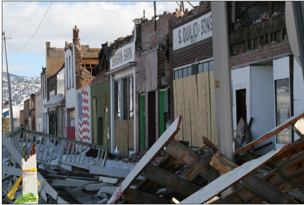
Figure 2. Wells historical district, where several unreinforced masonry buildings were damaged by the 2008 earthquake.
