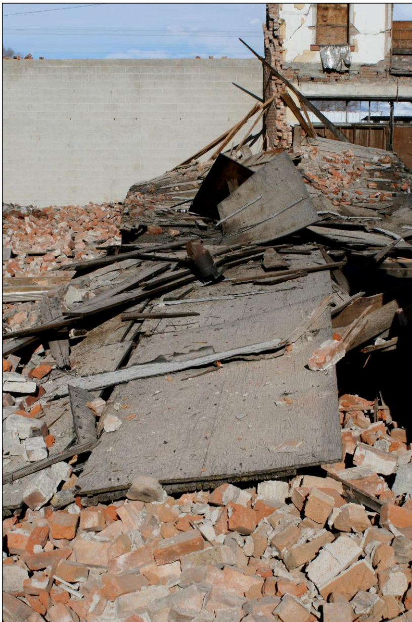
Figure 25. The roof of the unreinforced masonry San Marin Hotel lies on top of the second story floor and the collapsed and disintegrated two-story western wall.
