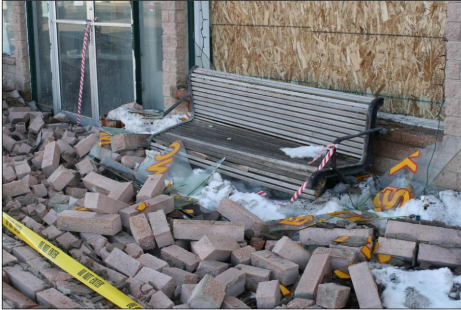
Figure 9. Bricks from an unreinforced veneer and broken glass from the front plate glass window are strewn about a bench on the sidewalk and the building's exit in front of the Overland Hotel. The early morning time of the earthquake helped prevent more injuries and possible deaths.
