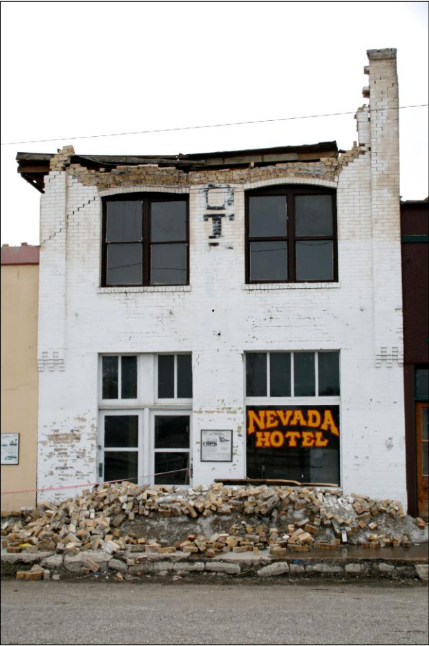
Figure 10. Partial collapse of the Nevada Hotel. Nearly all of the upper parts of the walls and parapets failed, dropping the roof down on the second story ceiling. Many bricks fell across the front exit of the hotel. Remarkably, for all this damage caused by shaking, none of the windows are broken.
