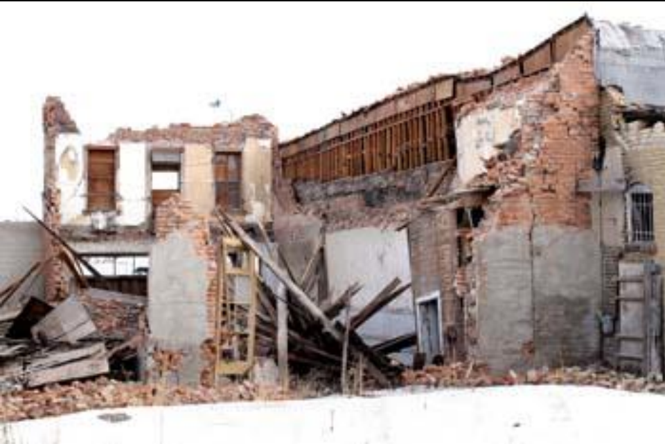
Collapse of unreinforced masonry building, Wells, 21 February 2008, magnitude 5.0 earthquake
