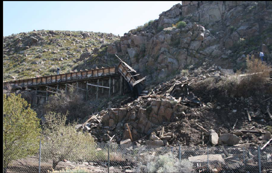
Damage to water flume, Mogul, 25 April 2008, magnitude 5.0 earthquake
