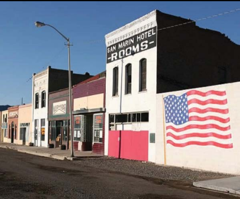
San Marin Hotel, Wells, Nevada before the 21 February 2008 M_w 6.0 earthquake
