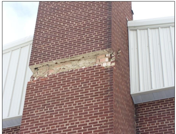
Figure 5. North wall of chimney.
