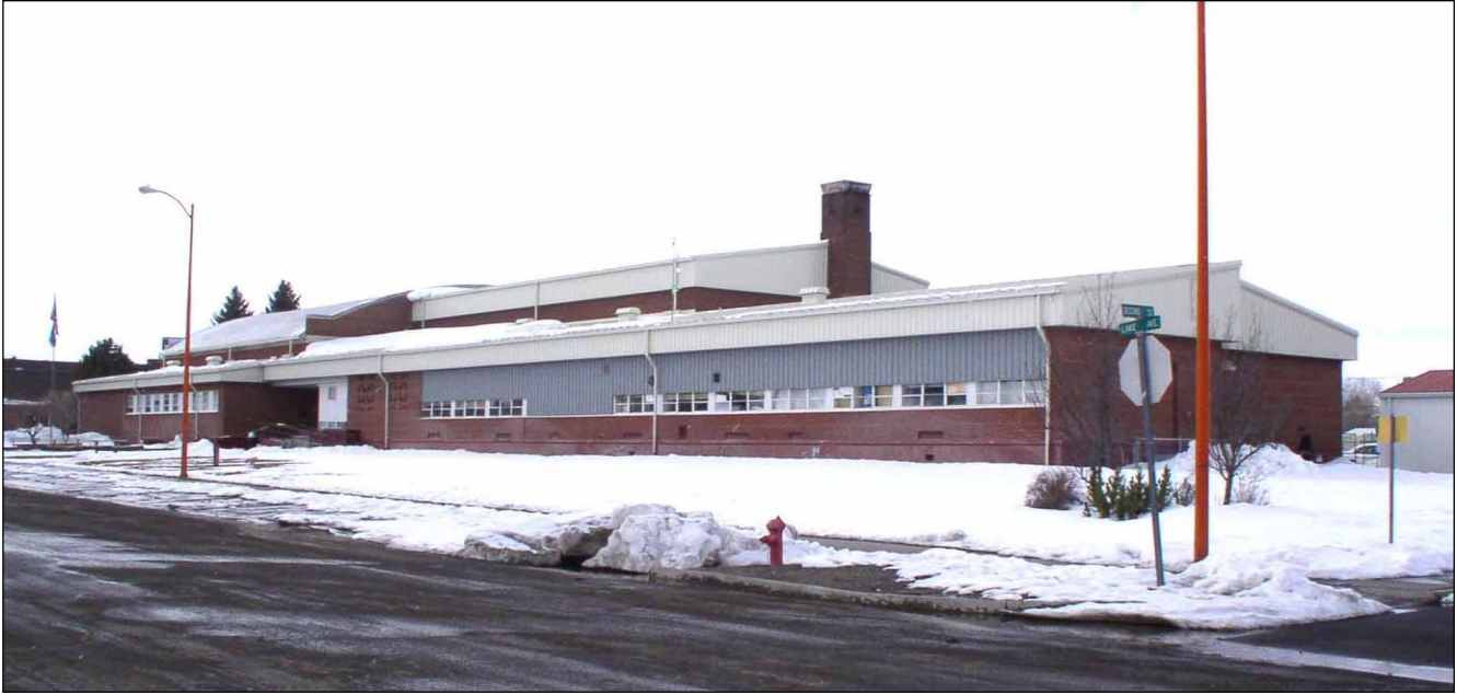
Figure 2. Wells High School, February 21, 2008.
