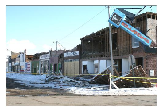
Figure 8. Wells historical district showing partial collapse of buildings and facades; this was an area of intensity MMI VIII.
