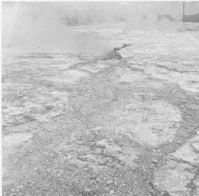
FIGURE 19.—Closed fissures near vent 39 on the crest of the Main Terrace. Fractures in sinter have controlled condensation of steam and oxidation of H_2S resulting in disintegration of opaline sinter adjacent to the fractures.
