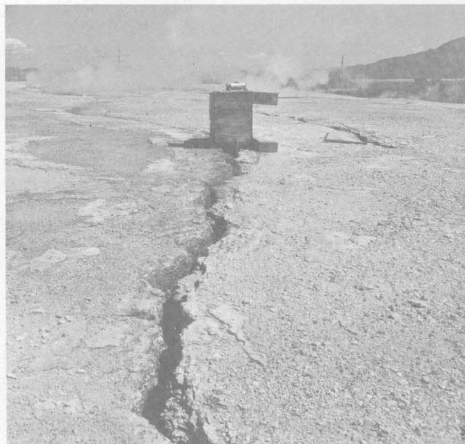
FIGURE 22.—An open fissure near the crest of the Main Terrace; view north toward a water-stage recorder installed at vent 35. The average width of the fissure is about 5 inches.
