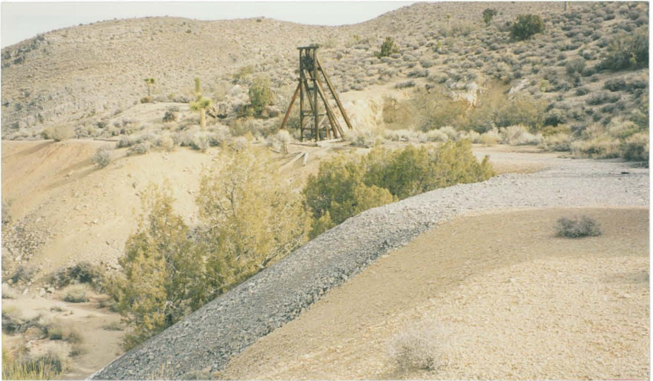
Photo 7-43 Headframe remaining over the main shaft of the Arrowhead Mine, Southeastern district ( R. Nicholson photo ).
