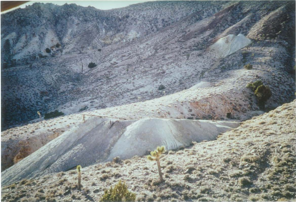
Photo 7-13 Mine dumps at the Urania Mine, Cactus Springs district. Lower dump is in the foreground, and upper dump is at upper right. The small dump between the two marks an air shaft connecting to the lower adit ( J. Tingley photo ).
