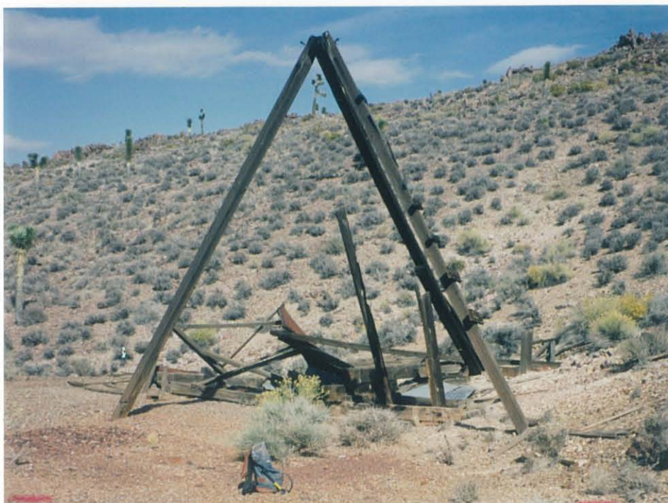
Photo 7-46 Headframe remaining over the Kelly Shaft, Papoose district ( R. Nicholson photo ).
