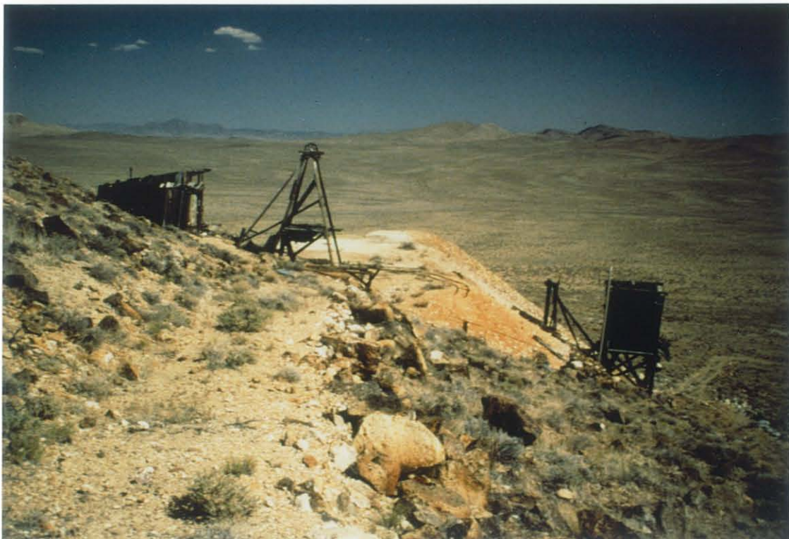
Photo 7-22 Headframe, hoist house, and orebin remaining at the Mellan Incline, Mellan Mountain district ( C. Henry photo ).
