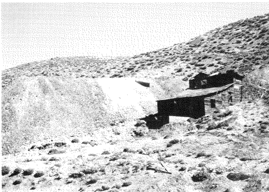
Main dump and mill remains, Twin Buttes mine, Staggs area. J. Quade photo.
