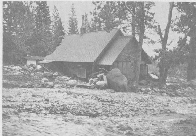
FIGURE 19. House destroyed by a flash flood on Galena Creek, in the summer of 1952. Four-foot boulders covered highway.
