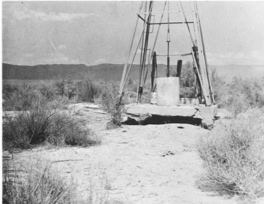
Well 5/37-20 bd. Note ground subsidence of about one foot beneath the concrete platform.
