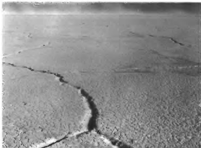
FIGURE 37.—Polygonal earthquake cracks in southern Carson Sink. Such cracks occur locally in clay of Seho formation east of the mouth of the Carson River. Two generations can be seen. The younger (fresher) was formed by tremors from the earthquake of January 1949, whose epicenter was near Verdi, Nev. Largest crack in foreground is about 8 inches wide. Sec. 33, T. 22 N., R. 30 E.
