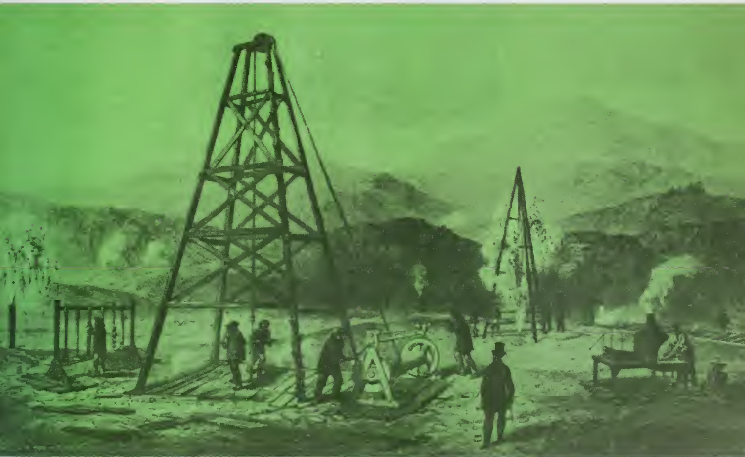
Photo 11. Early system of drilling wells in thermal areas at Larderello, Italy. From an old print.
