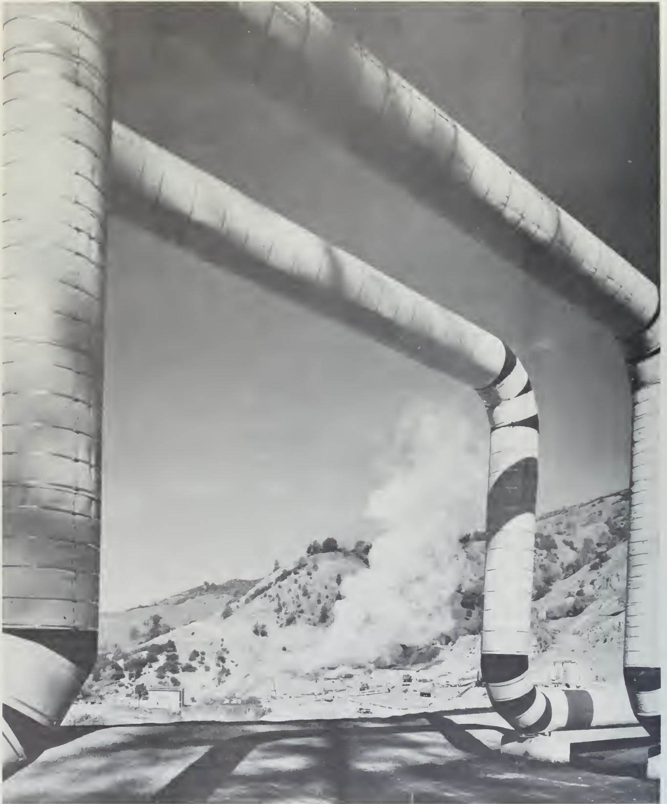
Geyser steam field seen through expansion bend in 2,000-foot steam line which transports steam from the field to the plant. Photo courtesy Pacific Gas and Electric Company.
