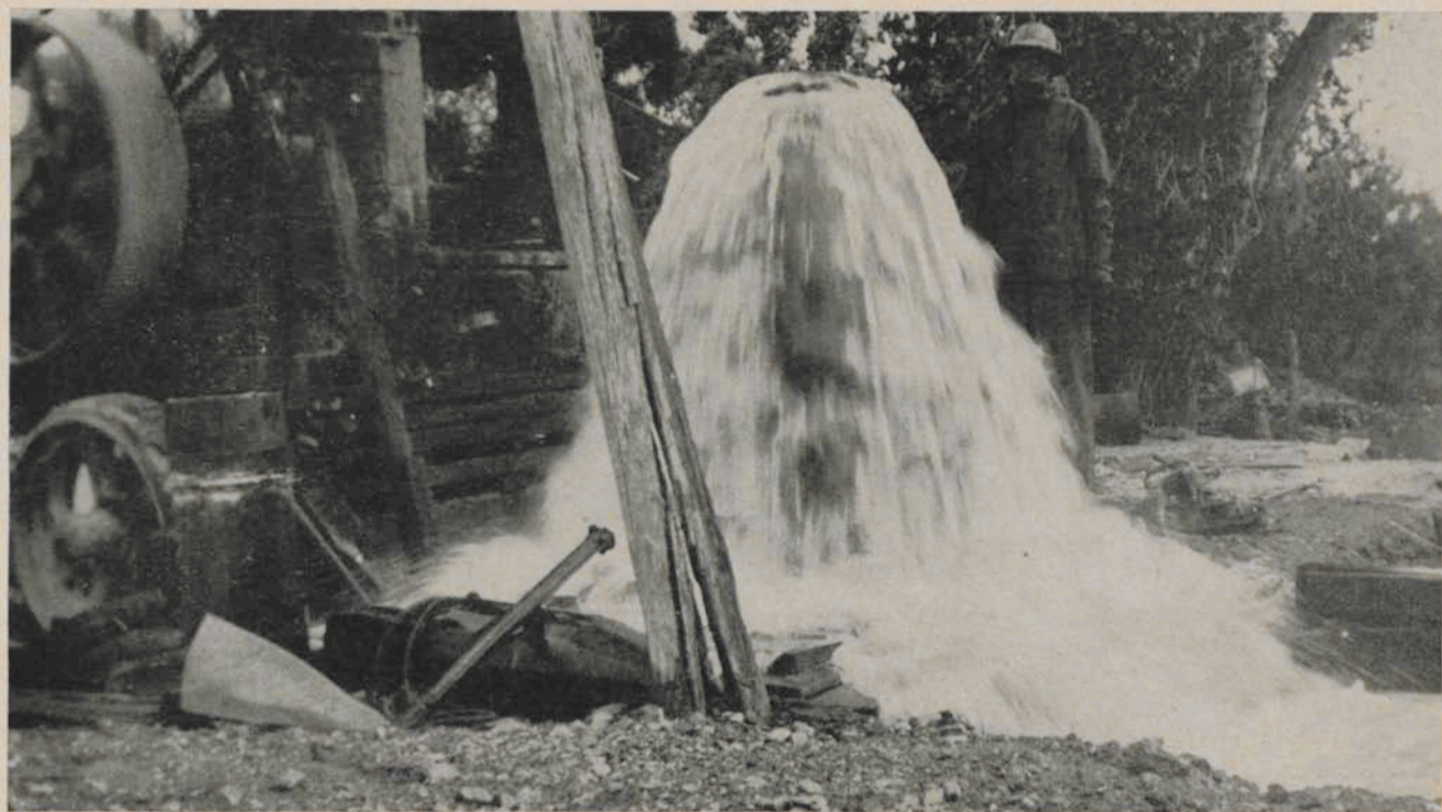
PLATE 3—Well (S-21-54) 3cad1. Manse Ranch, Pahrump Valley, Nevada. Flowing 3,450 gallons per minute in February 1941
