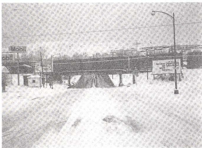
Figure 7. State highway snow melt system heated by a downhole heat exchanger (DHE).
