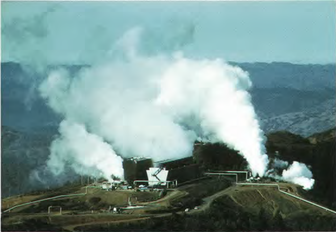
Geothermal powerplant at The Geysers near Santa Rosa, California. Photograph courtesy of Pacific Gas and Electric Company.
