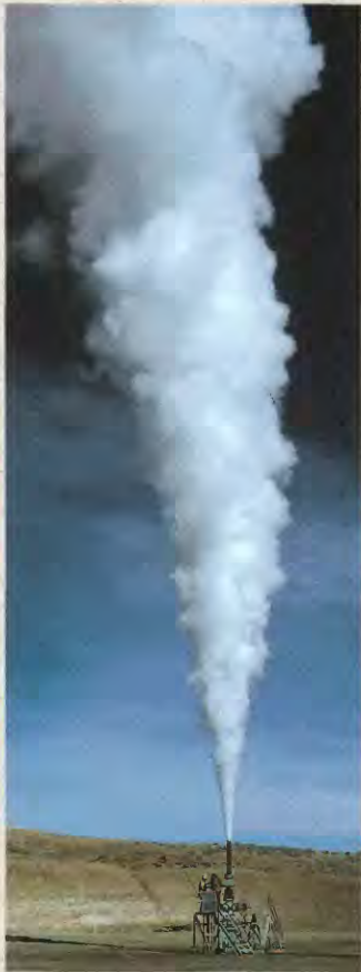
First geothermal well drilled at Coso geothermal area, south-central California, by private industry. It, together with a few other wells, has been developed to feed steam into the initial powerplant.
