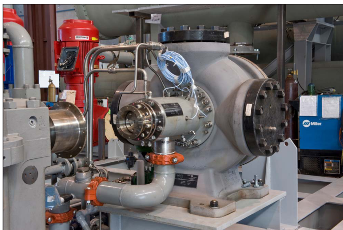
Figure 3. Manufactured Turbine in the TAS Shop.
