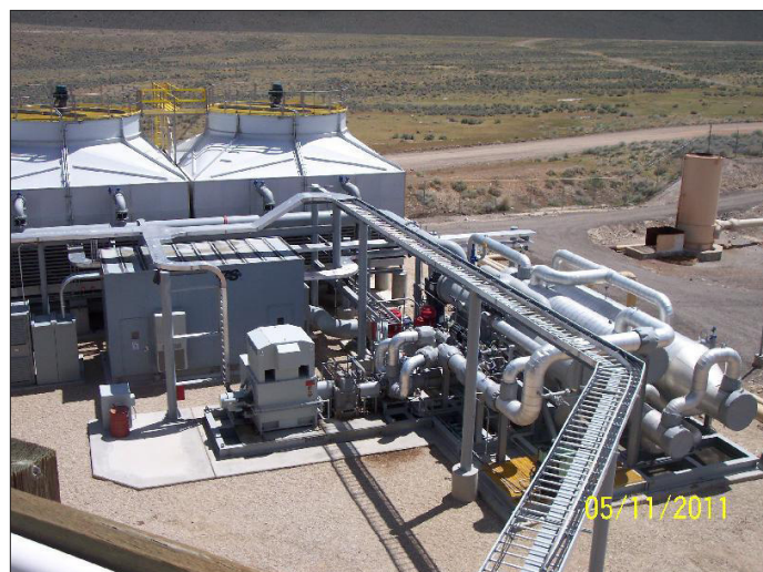
Figure 6. Beowawe Modular Bottoming Plant operating in field.
