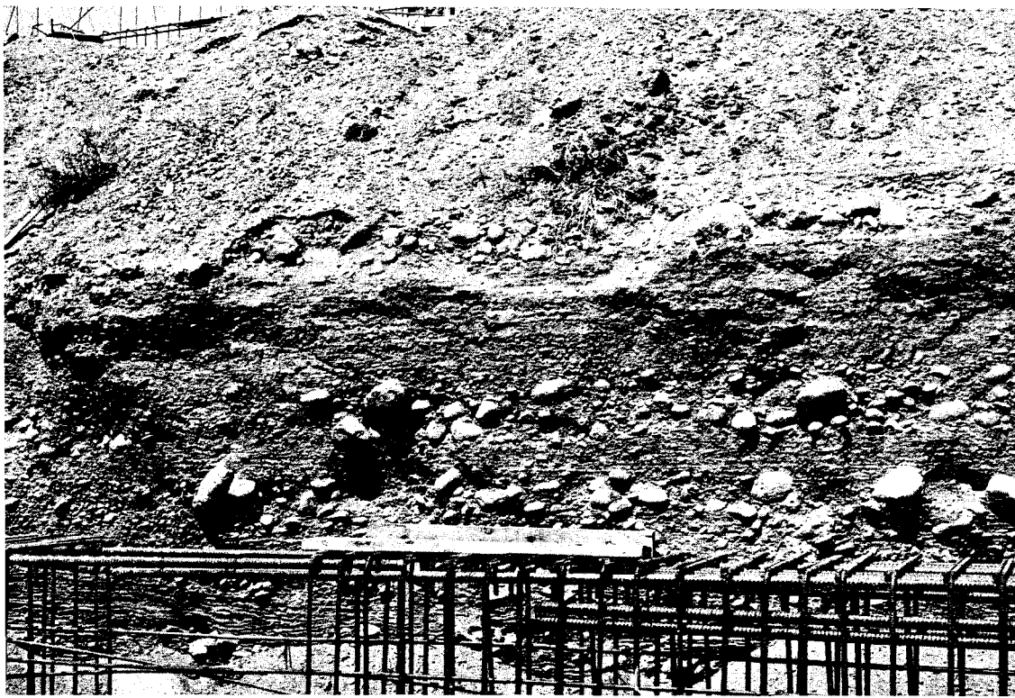
Bouldery Tahoe outwash overlain by a thin veneer of Holocene gravely sand reworked locally from the alluvial fan deposits of Peavine Mountain. Excavation for Interstate 80
