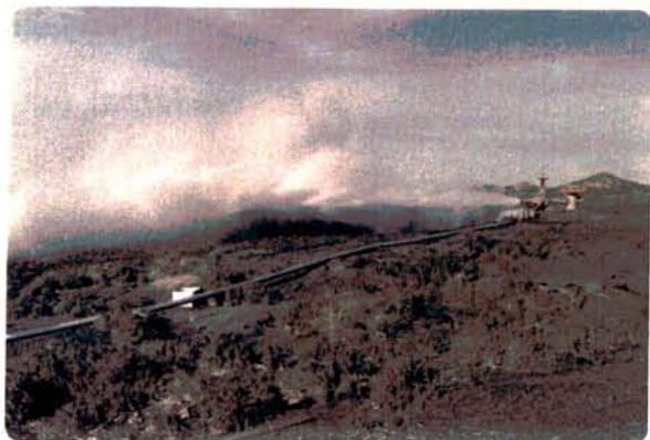
Figure 10. - Bradys Hot Springs. View northwest at most active of 6 Magma Power Co. steam wells. Twenty-in. conductor pipe and 13 3/8-in. casing are cemented to surface. Eight-in. valve and flow line. Steam jet is about 50 ft., with reported pressure 50 psi at well head. Aggregate water discharge is 25 GPM (est.). Catchment trough and pipe for local domestic heat and washing use.
