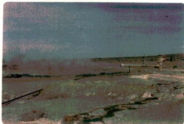
Figure 11. - Bradys Hot Springs. View north at second active Magma Power Co. steam well. Completion and equipment same as well shown in fig. 10. Flow is by heads, aggregate water 15 GPM. Water temperature 204°F at well head.
