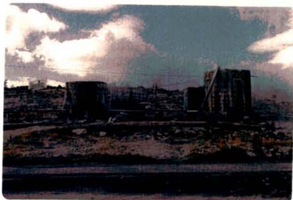
Figure 16. - Steamboat Springs. Wells at spa for arthritics. Note heavy deposits on catchment and cooling tanks. Water temperature 193°F. This Steamboat-Reno spring area is geologically well known because waters are depositing gold and silver.
