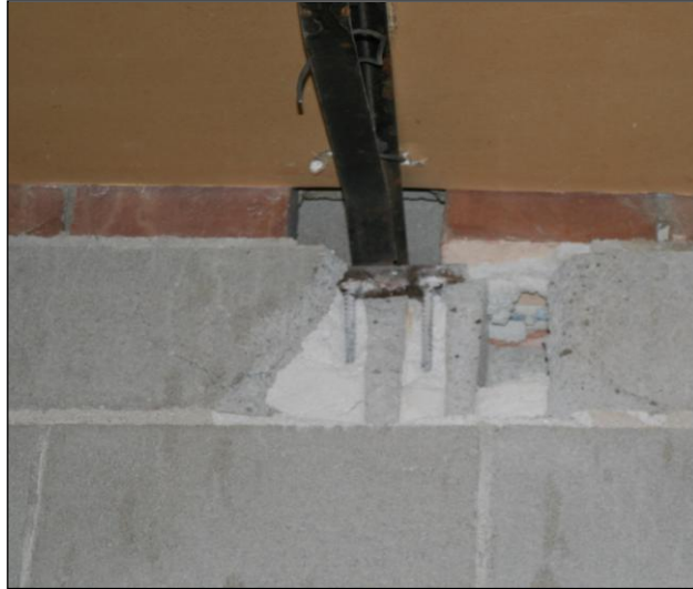
Figure 17. Interior damage to ceiling beam in the Wells High School. Photograph by C.M. dePolo.
