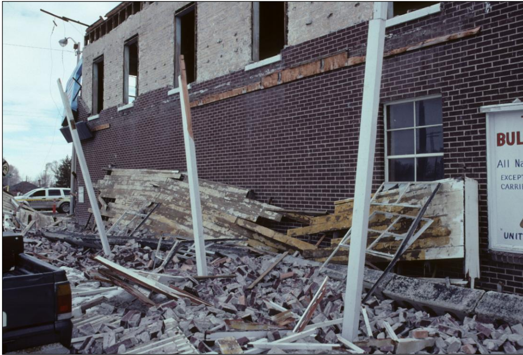
Figure 4. Western side of the Bullshead Bar. The balcony has been smashed to the ground abruptly breaking the column connections and leaving the columns still standing. Wells ReMi Line 3 was laid out along the avenue this balcony was along. Photograph by C.M. dePolo.
