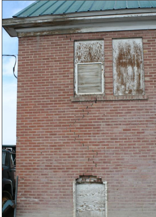
Figure 21. Damage to the City Shop wall.
