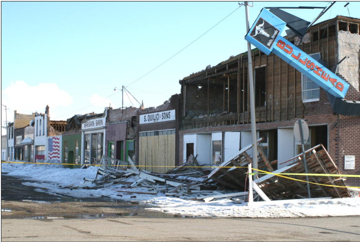
Figure 12. Damage along 7 th Street from the Wells earthquake. Line 2 was laid out along the edge of the street in front of these damaged buildings. The Bullshead Bar is on the corner of the street, near the intersection of Lines 2 and 3. Photograph by C.M. dePolo.
