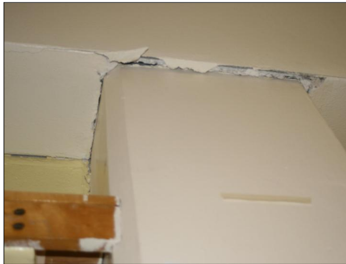
Figure 18. Interior damage in hallway at the high school. Photograph by C.M. dePolo.
