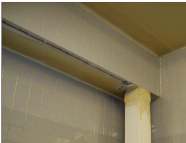
Figure 24. Earthquake damage at the 4-Way Casino, Nevada. Interior cracking near a column and beam. Photograph by 4-Way employee.
