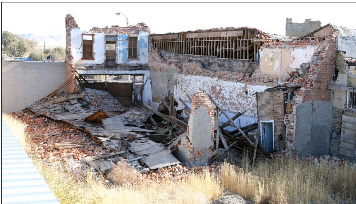
Figure 3. Collapsed, two-story San Marin Hotel, viewed from the back. The western wall (left side) has collapsed bringing down the second story floor and the roof; only the lower corners remain of the western wall. Wells ReMi Line 2 was laid out on the street in front of this building. Photograph by C.M. dePolo.
