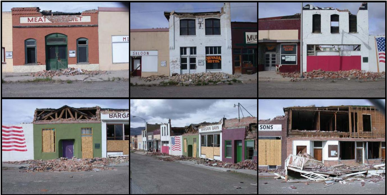
Figure 2. Photographs showing the extensive damage to the historic old town area on Front Street, Wells, Nev. (photos by D.A. Ponce).
