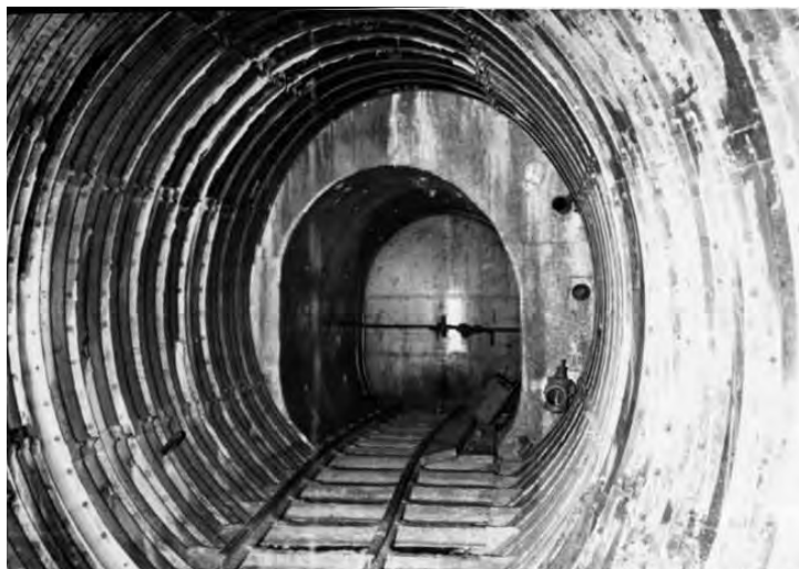
Figure 3. – Water door installed in the FAD workings by Eureka Corp. in 1941
