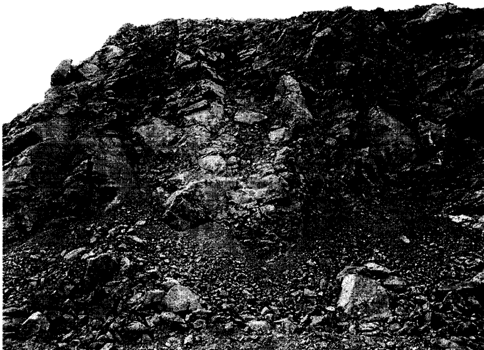
Figure 35. Marble, 1340 bench, Shepard pit. 20' bench height. The marble is the blocky material cropping out on the left side of the photo.
